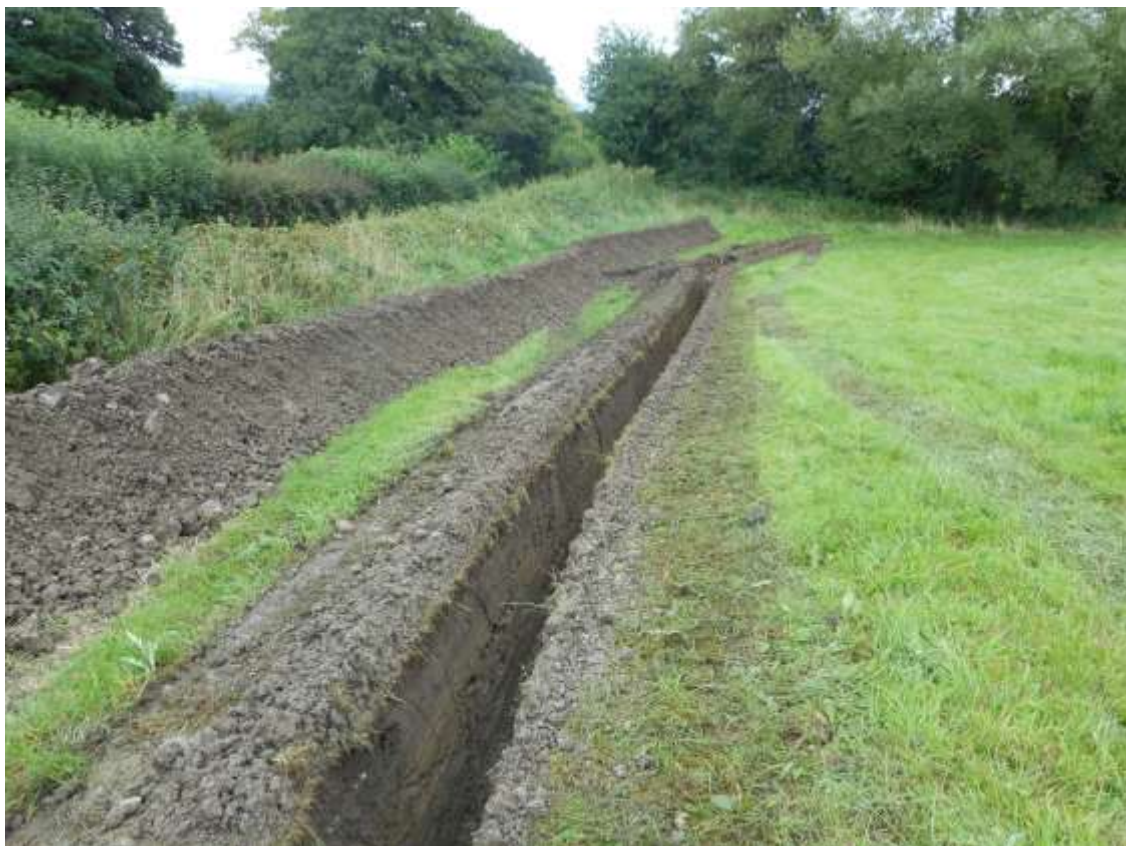
Plate 6: View E towards stream crossing showing trench in Field 4
