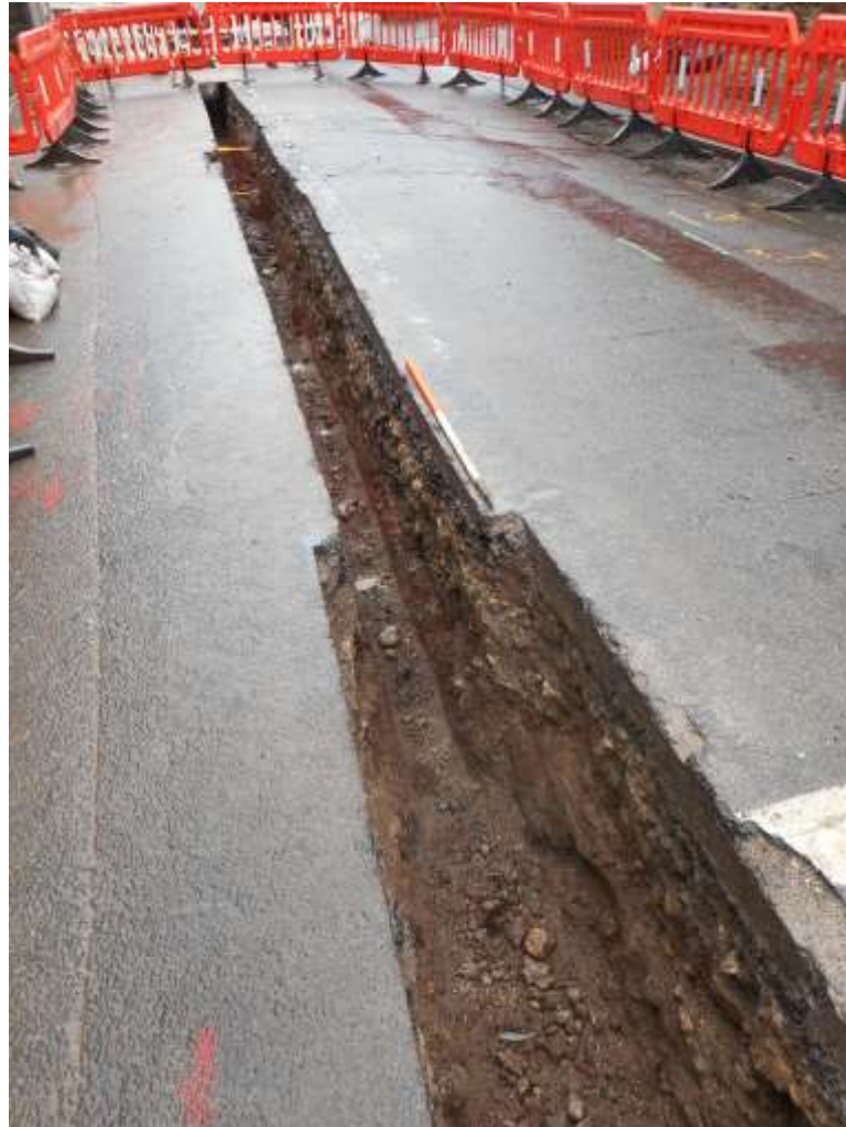
Plate 2: View NW of Trench 2
