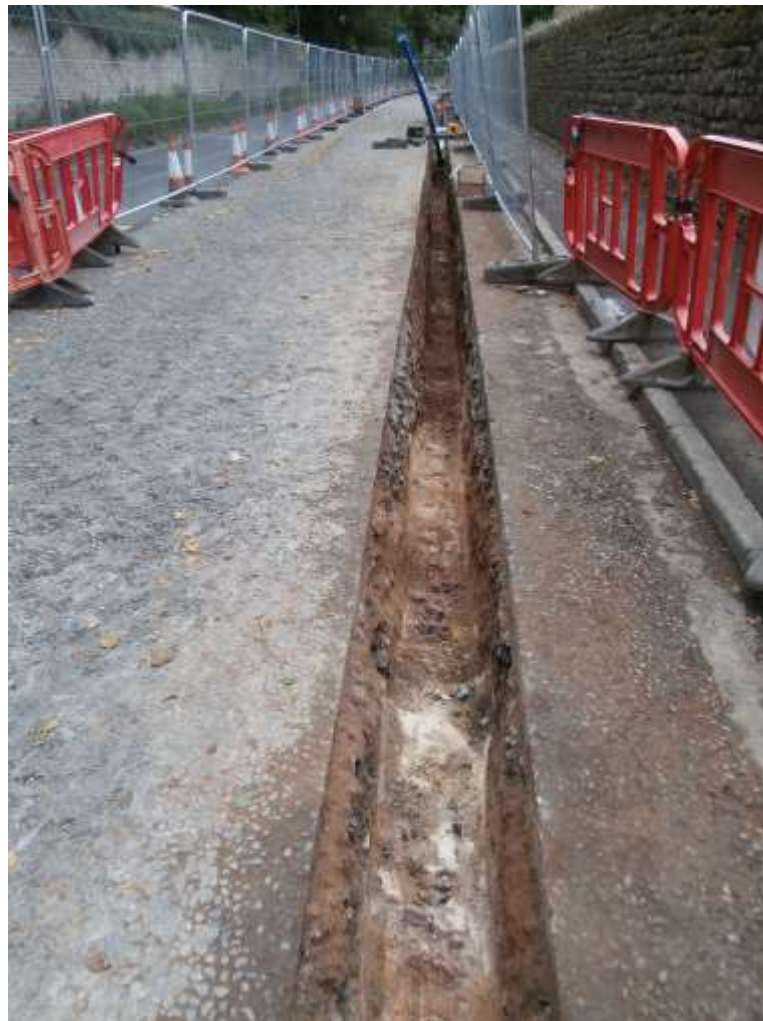
Plate 1: Trench 1, view to the SW
