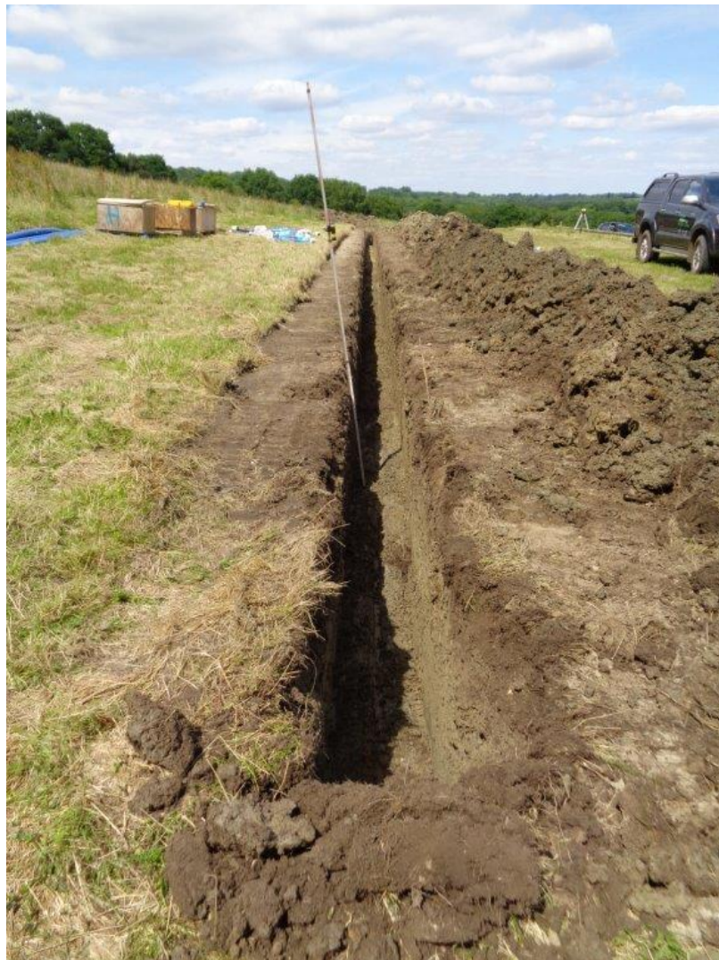
Plate 5: Post-excavation view NW showing extent of pipeline trench
