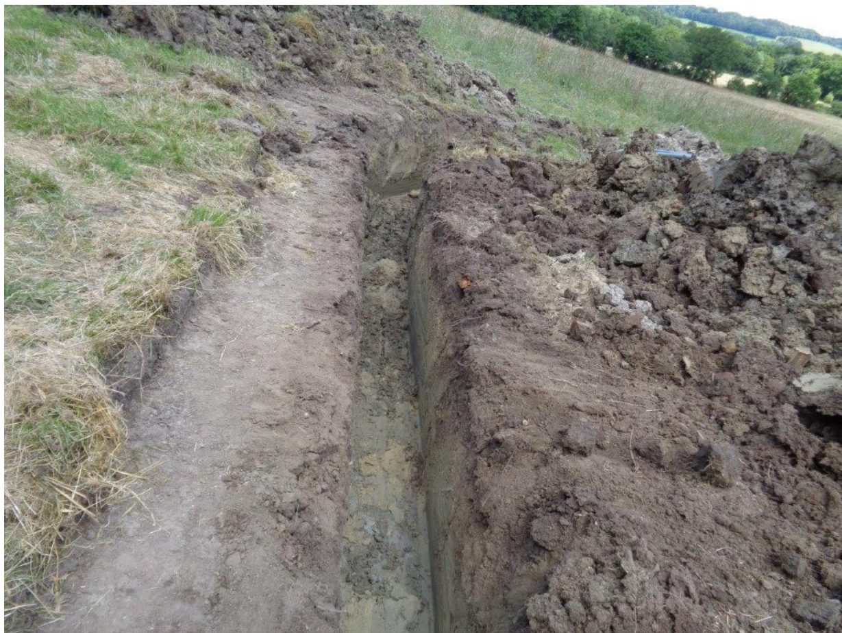
Plate 3: N end of trench showing bend to accommodate pipeline
