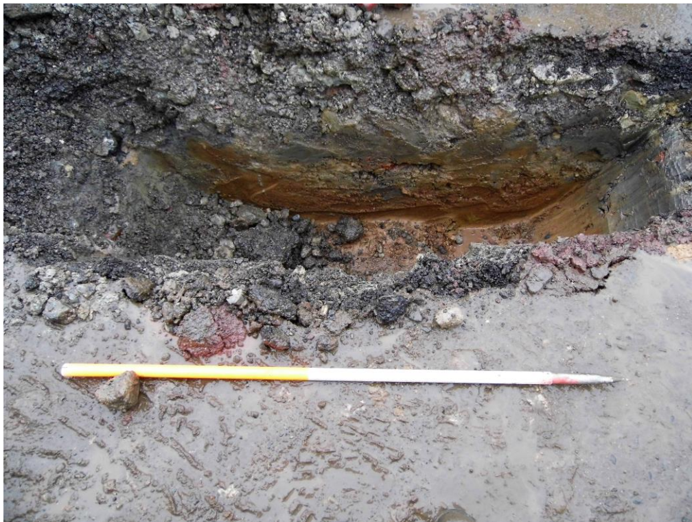
Plate 1: Access Pit 3 under excavation within the Scheduled Area; view N
