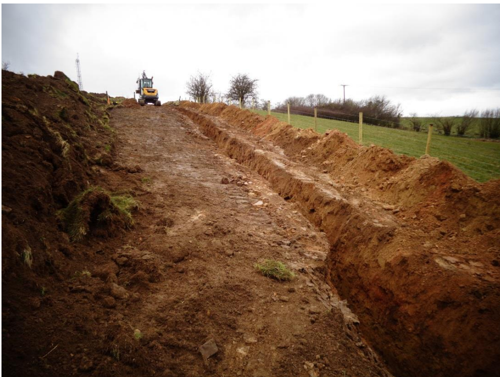
Plate 5: Upslope view NW of completed trench
