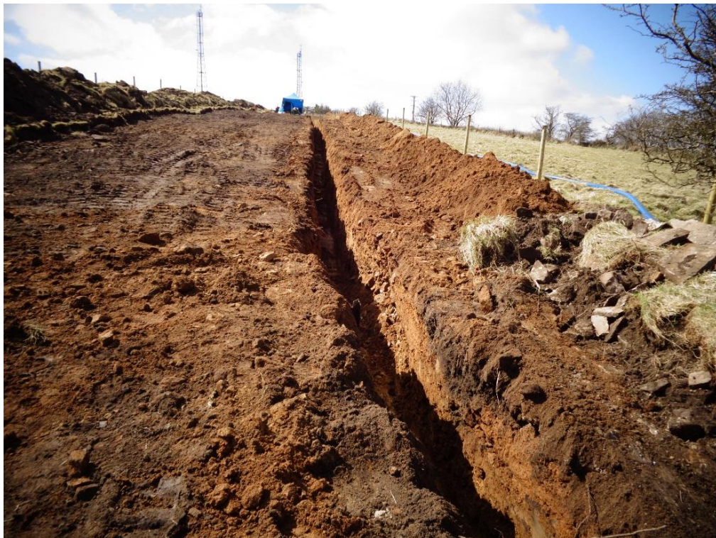
Plate 3: View W of trench, mid slope
