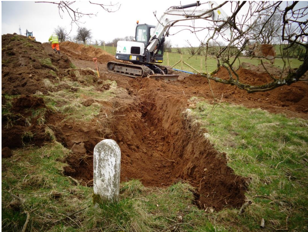
Plate 6: View NW showing water marker at trench terminus
