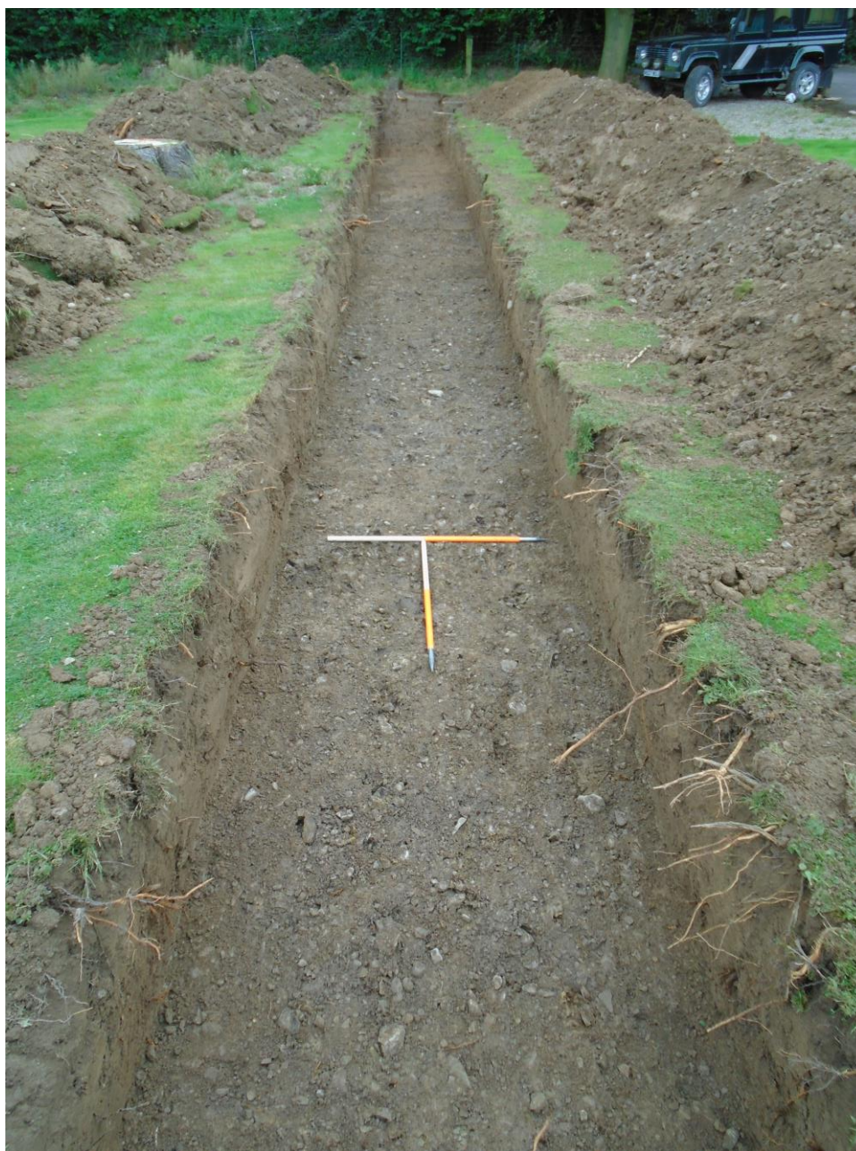
Plate 2: View SE of Trench 001
