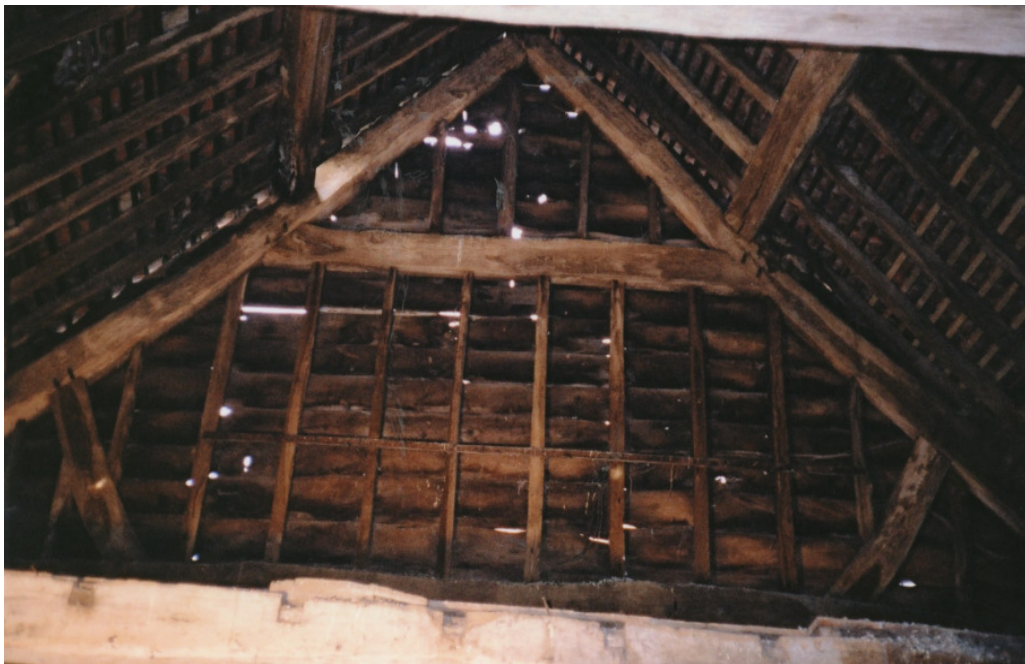
Fig. 10: Room 1 showing roof structure
