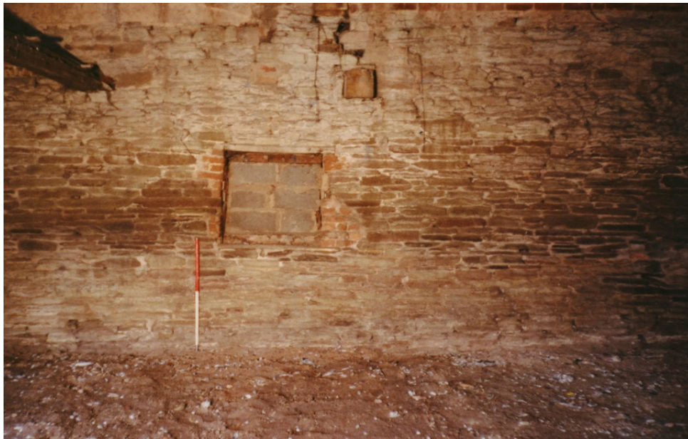
Fig. 8: Room 1 W-facing wall with blocked window
