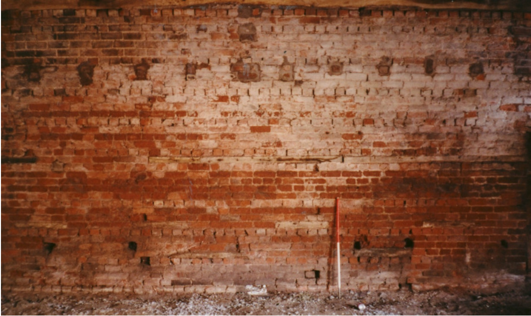
Fig. 13: Room 1 N-facing interior wall
