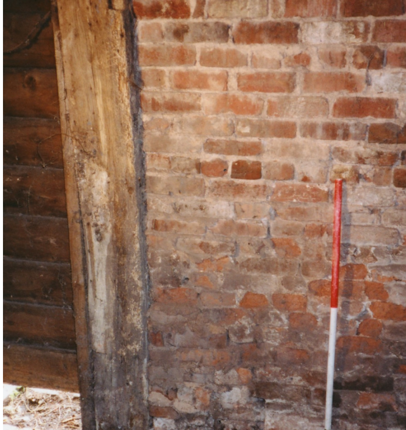
Fig. 17: Room 2 N-facing interior wall
