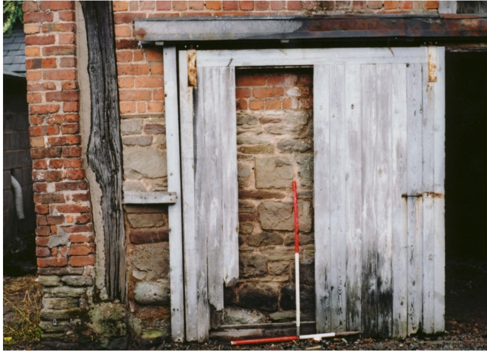
Fig. 5: W. Elevation showing 20 th century sliding door & timber frame
