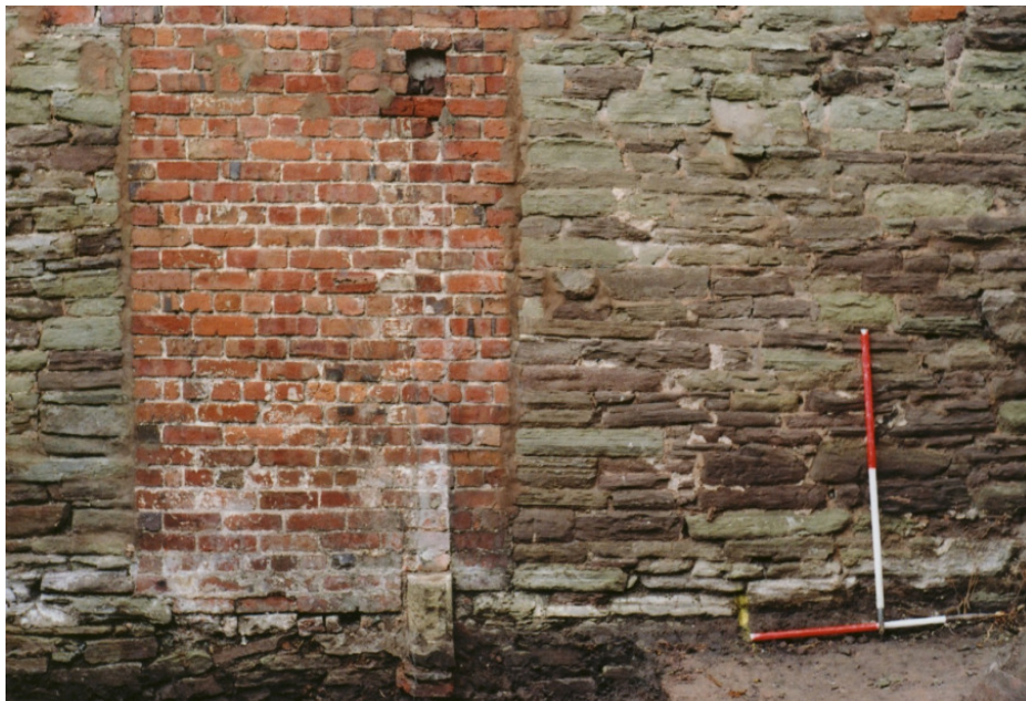
Fig. 18: Building 2 E-facing wall showing composite structure
