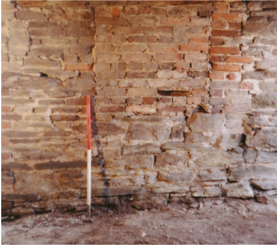
Fig. 7: Room 1 E-facing wall with blocked window
