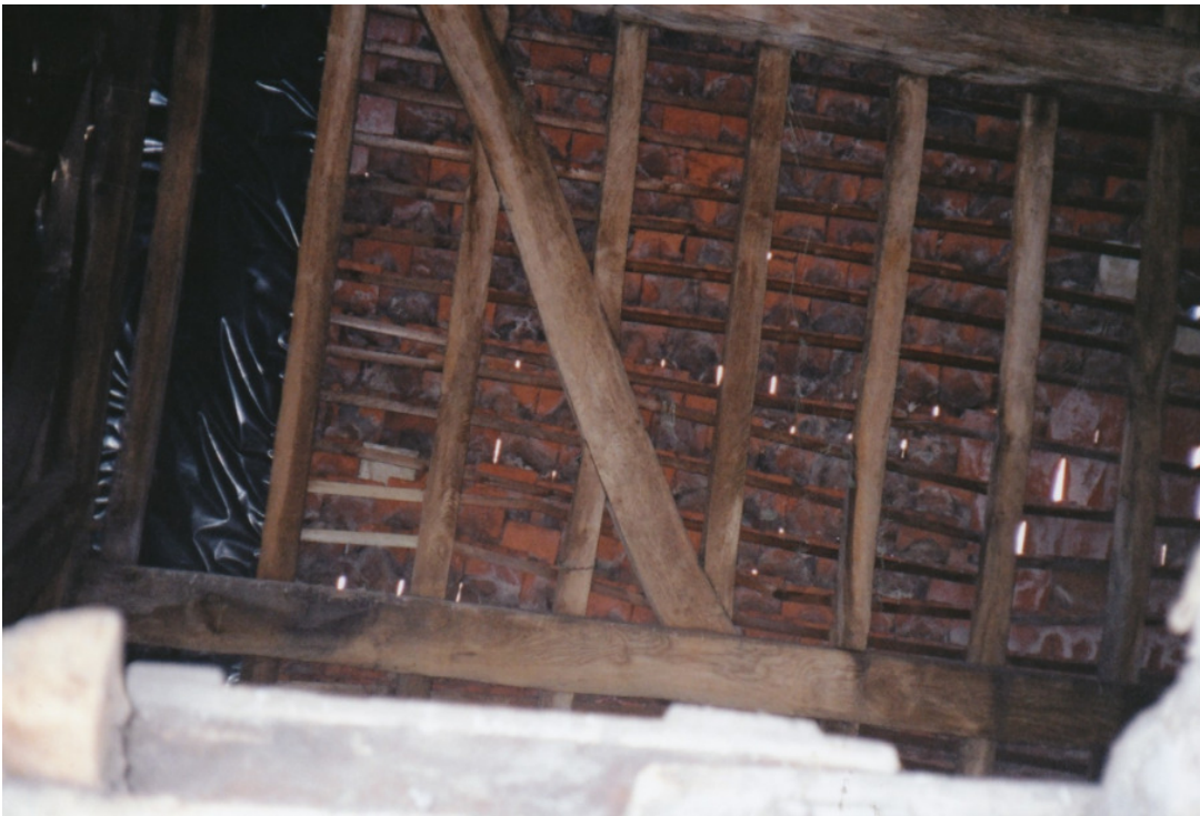
Fig. 12: Room 2 showing detail of roof structure
