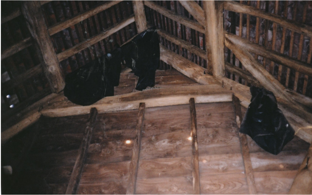
Fig. 11: Room 2 showing roof structure
