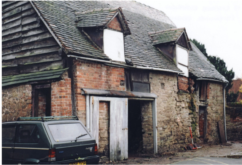
Fig 1: Exterior W elevation of Building 1
