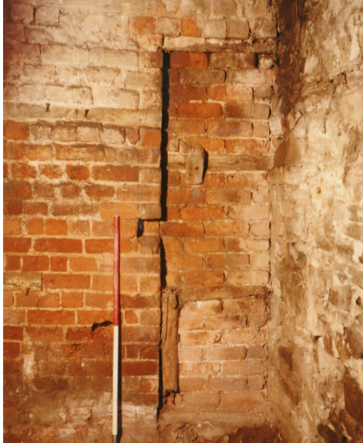
Fig. 15: Room 1 detail of N-facing interior wall showing blocked doorway
