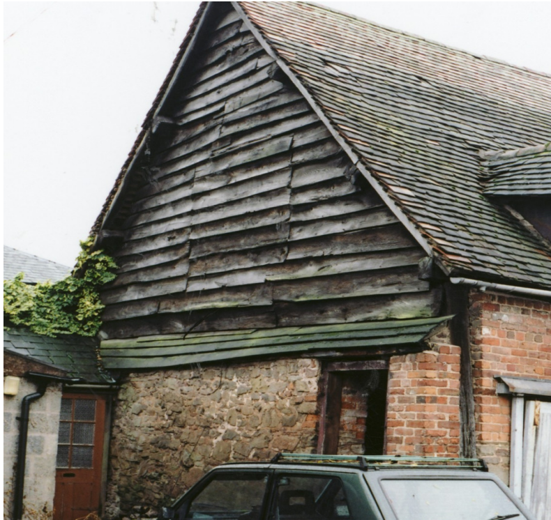
Fig. 3: N elevation showing pitch of roof & weatherboarding
