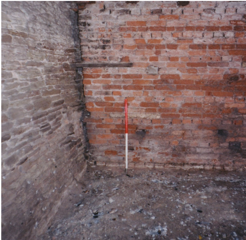
Fig. 14: Room 1 detail of N-facing interior wall
