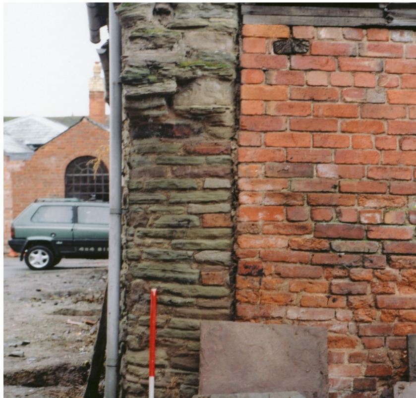
Fig. 2: Exterior S-facing wall showing bonding
