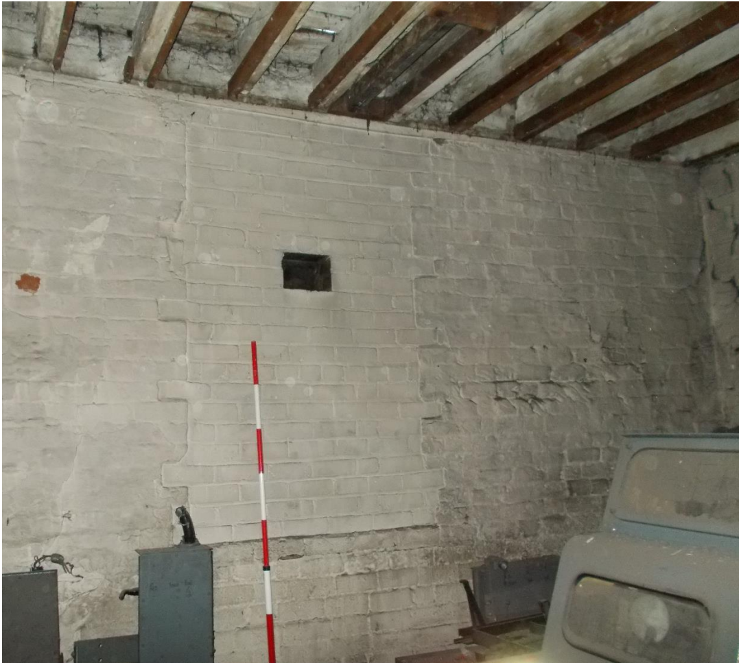
Plate 12: Internal view looking NNE showing blocked window with modern ventilation grille inserted in eastern bay of Building A
