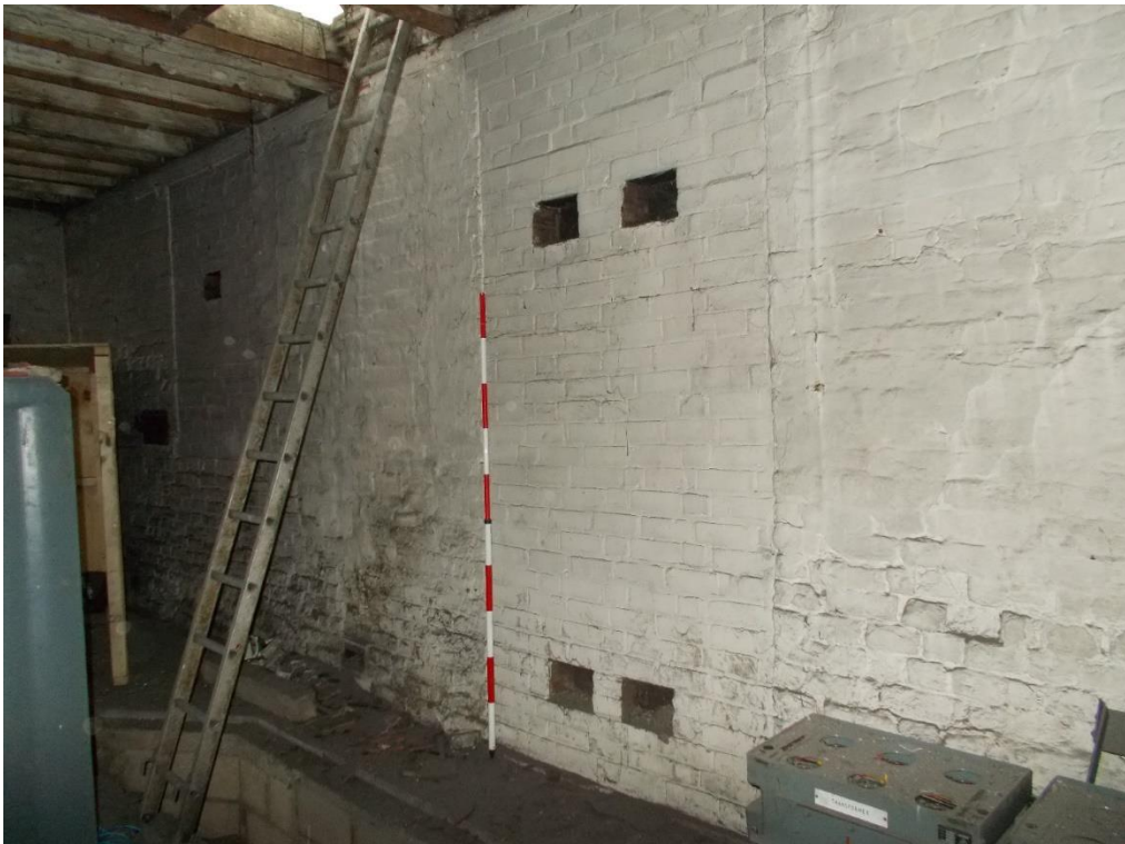
Plate 10: Internal view looking NW showing blocked doorway in N wall of Building A with hatch above and to left of doorway
