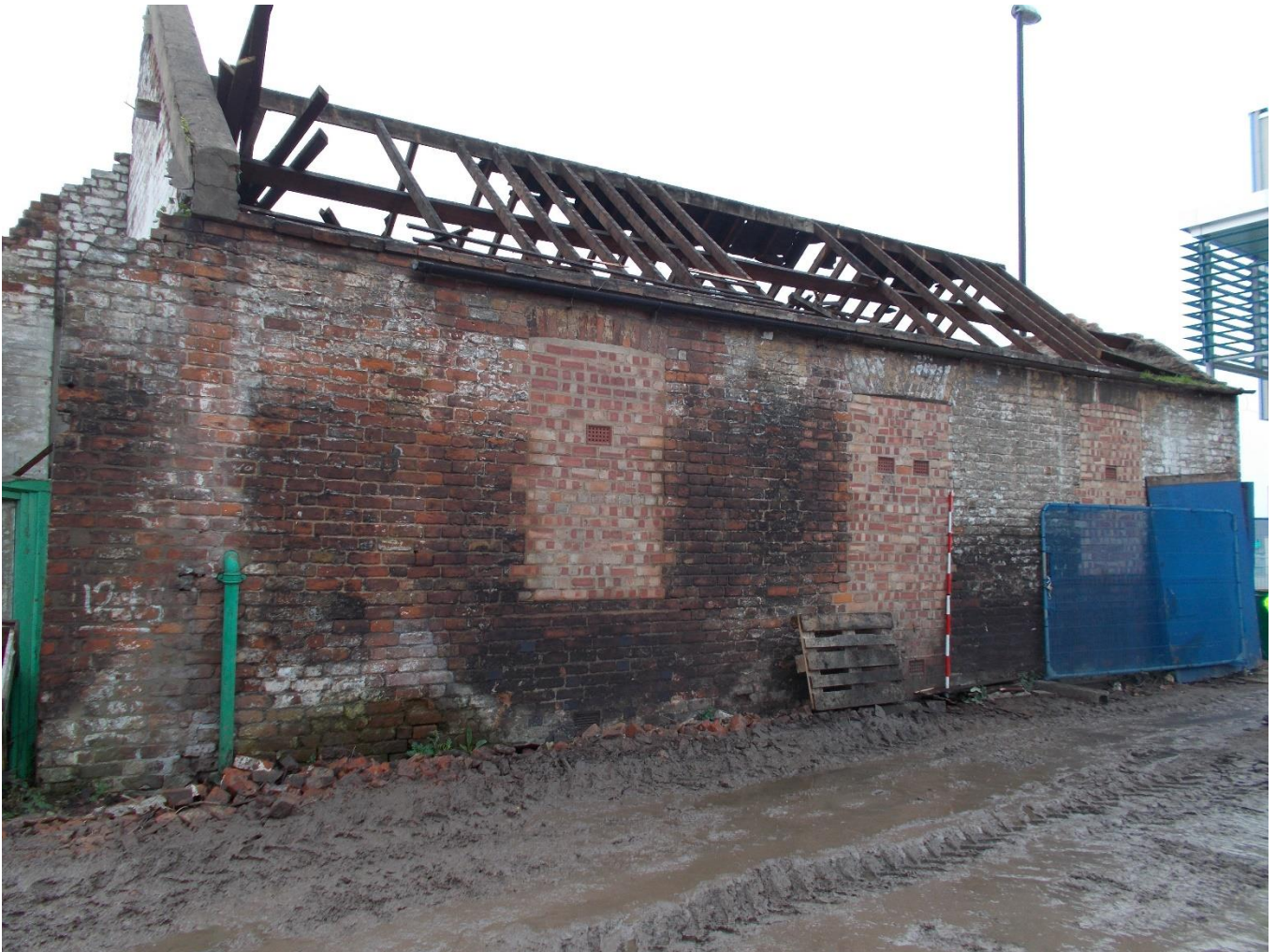
Plate 3: View looking SE showing N-facing elevation of Building A with doorway with gauged brick voussoirs flanked by two segmental arched windows, all bricked-up
