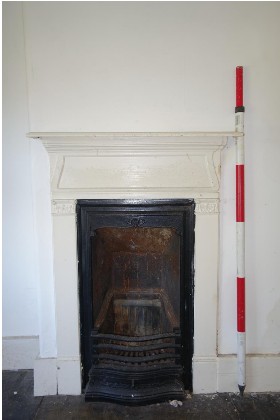
Plate 28: In-situ painted cast iron fireplace in N wall of Bedroom 4.
