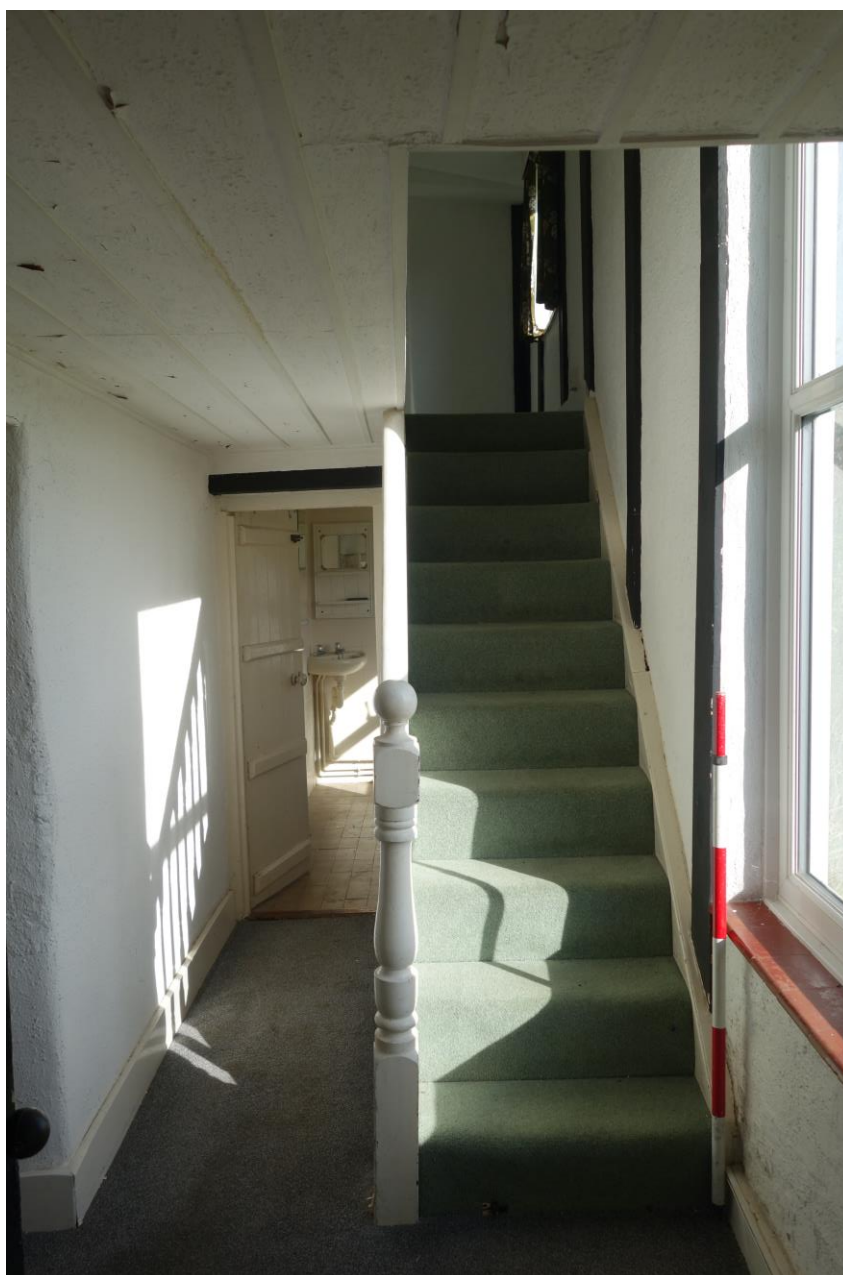
Plate 16: View N of Rear Hall showing shower room and staircase to first floor.
