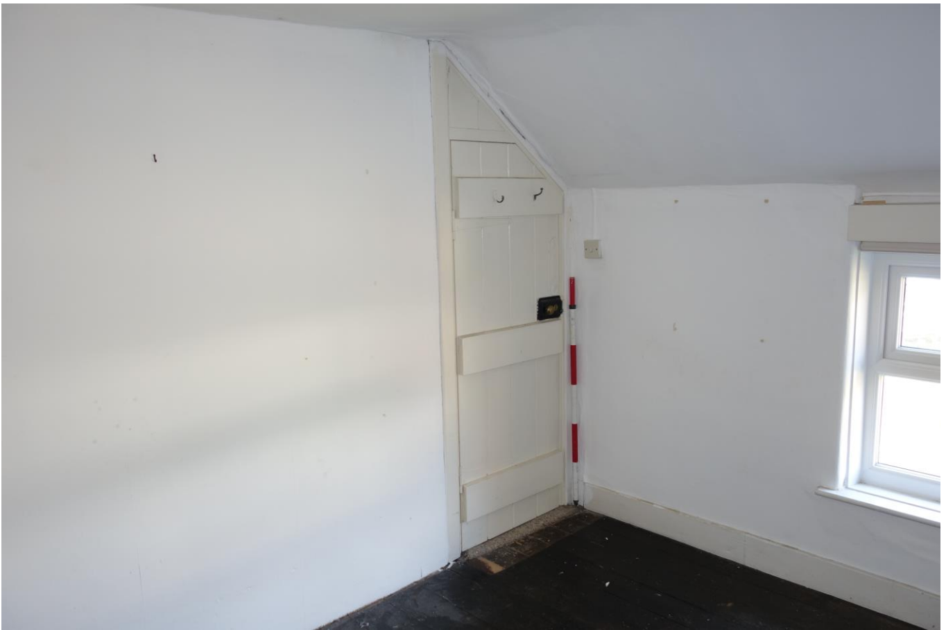
Plate 30: View SW of Bedroom 4 showing connecting door to Bedroom 2 with modern UPVC window shown right of picture.
