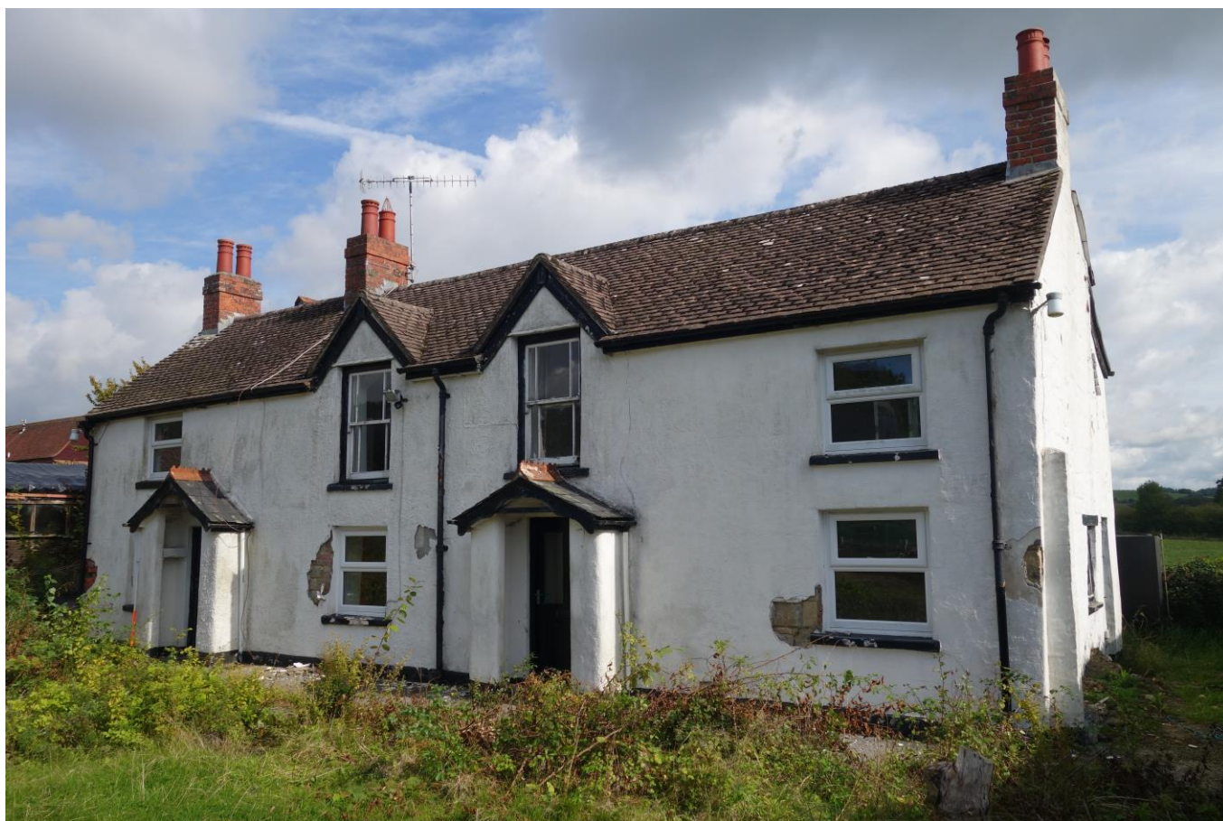
Plate 2: Oblique view NE showing front (W) and S elevations.
