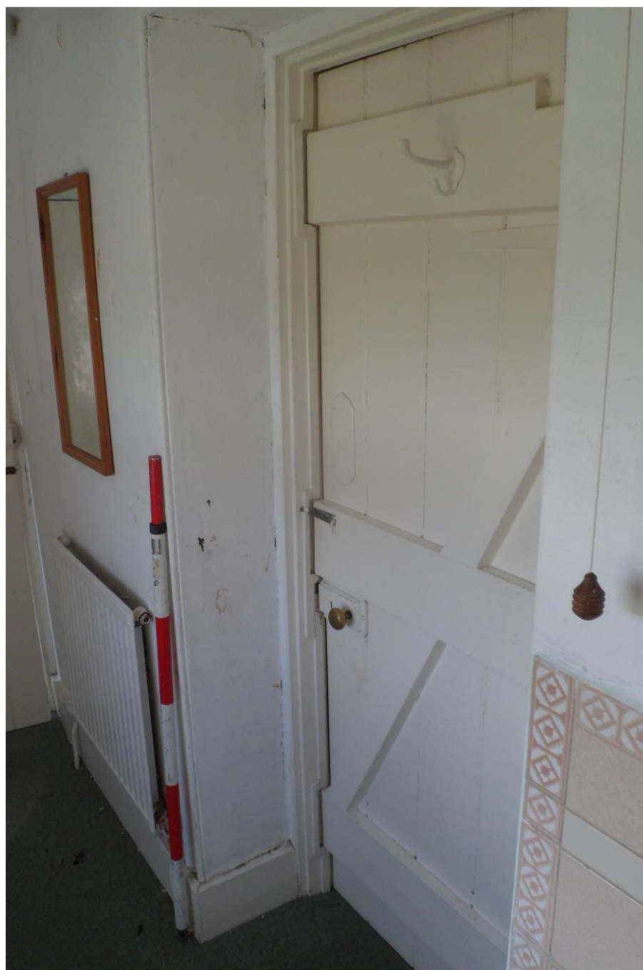
Plate 32: View SSW of connecting door from Bathroom into Bedroom 4.
