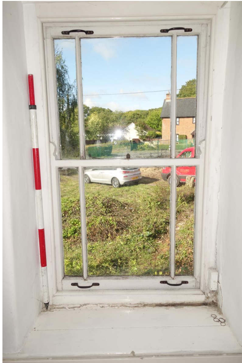
Plate 26: View W of timber sash window in Bedroom 2.
