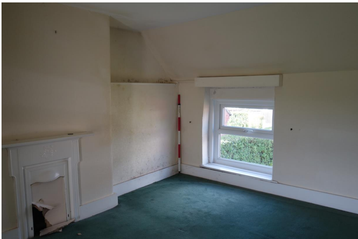
Plate 21: Bedroom 3 showing cast-iron fireplace and UPVC window in front elevation.
