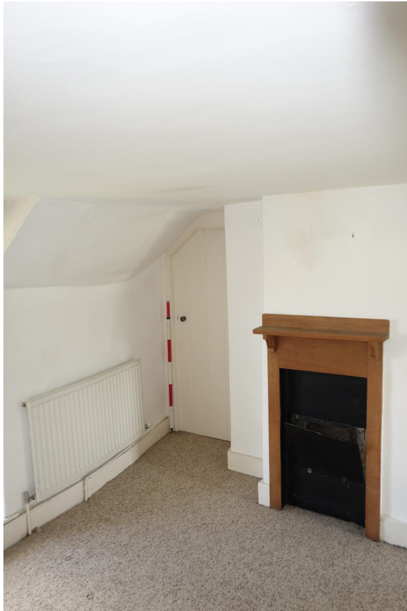
Plate 24: View NW of Bedroom 2 showing former blocked fireplace with 20 th century surround and connecting door with Bedroom 4.
