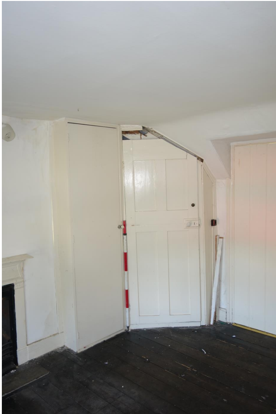
Plate 27: View NW of Bedroom 4 showing fireplace (left) and with partition housing hot water cylinder shown (centre) and connecting door into Bathroom (right).
