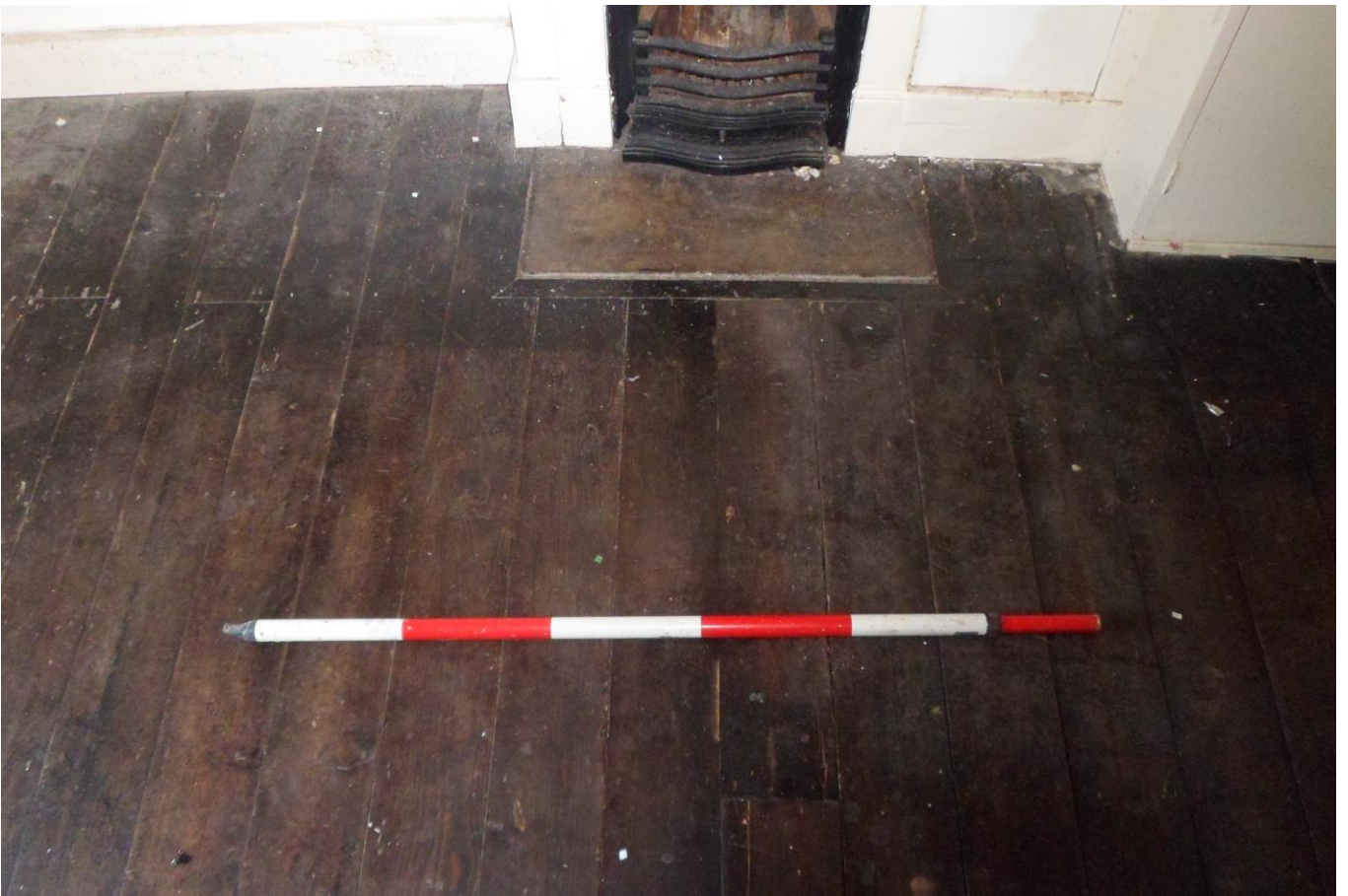
Plate 29: Exposed stained N/S softwood floorboards in Bedroom 4.
