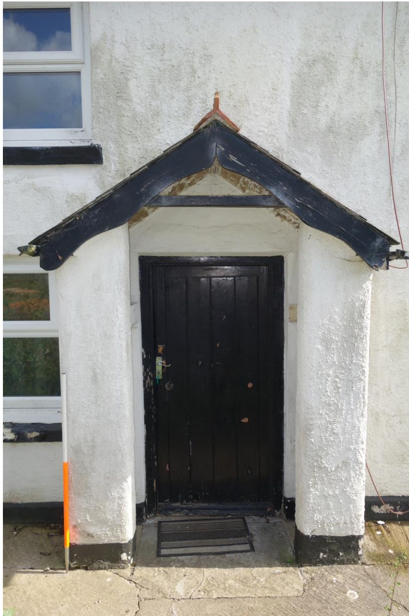
Plate 5: External frame and plank door opening into Living Room.
