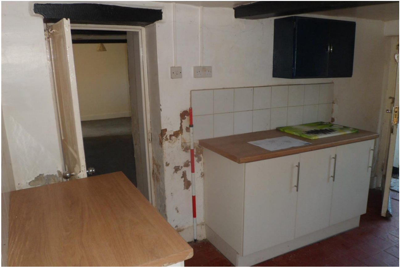
Plate 9: Doorway from kitchen through to Living Room showing exposed N/S ceiling beam, with front door shown right of picture.
