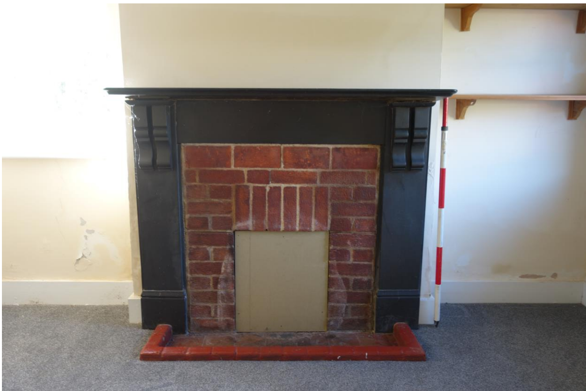
Plate 14: Brick fireplace in Study with slate fire surround and integrated mantel.
