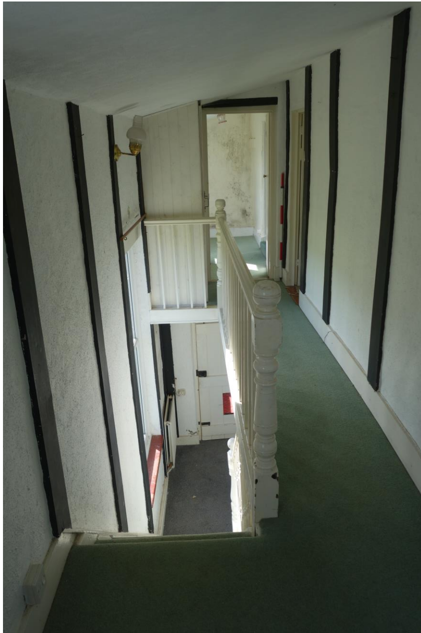
Plate 18: View S along Rear Hall (Upper) towards Bedroom 3.
