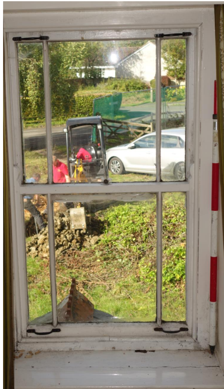
Plate 22: Bedroom 1 showing timber sash window in dormer with ridge tiles of front door porch visible
