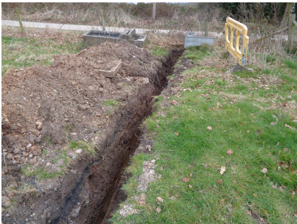
Plate 5: View N of Trench 2 showing brick and concrete inclusions within subsoil (402).
