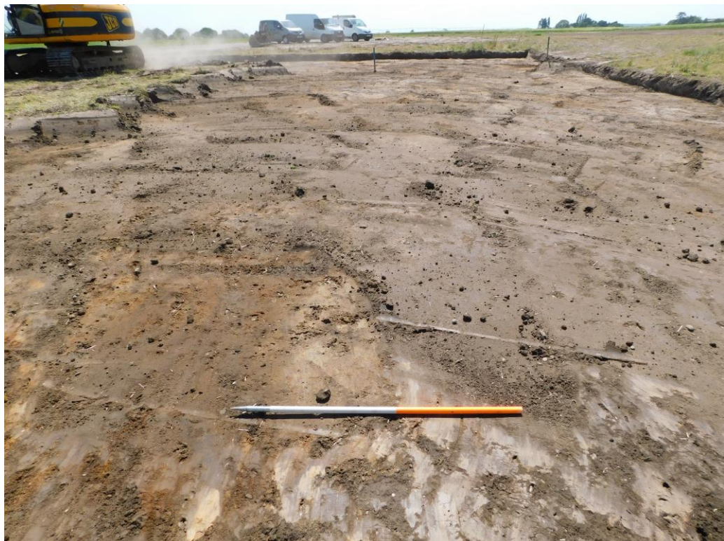
Plate 2: SW extent of topsoil strip
