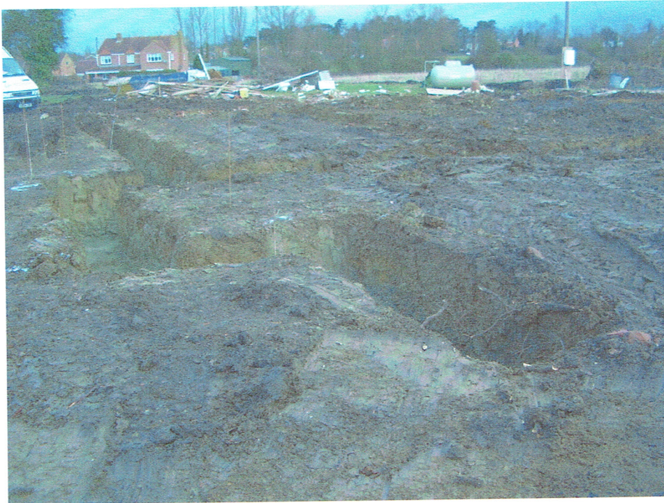
Plate 1: General view of site, looking N
