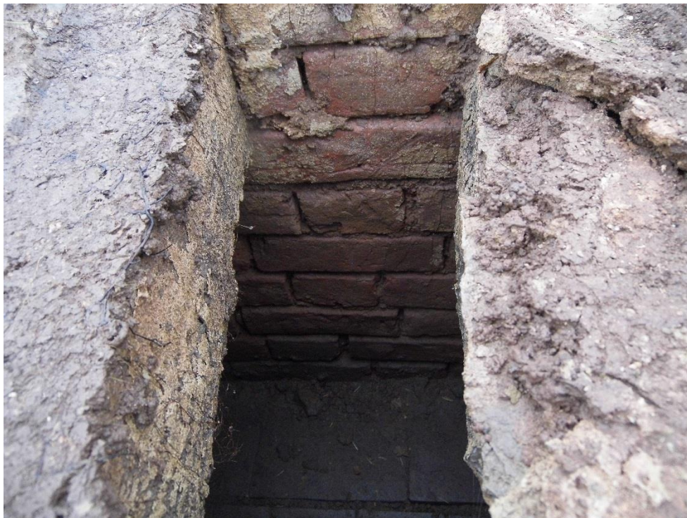
Plate 1: View inside inspection chamber (1009)
