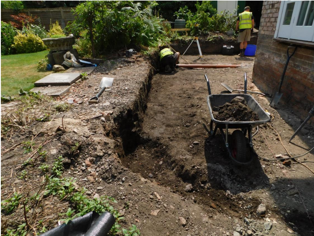
Plate 3: View SW showing foundation excavations
