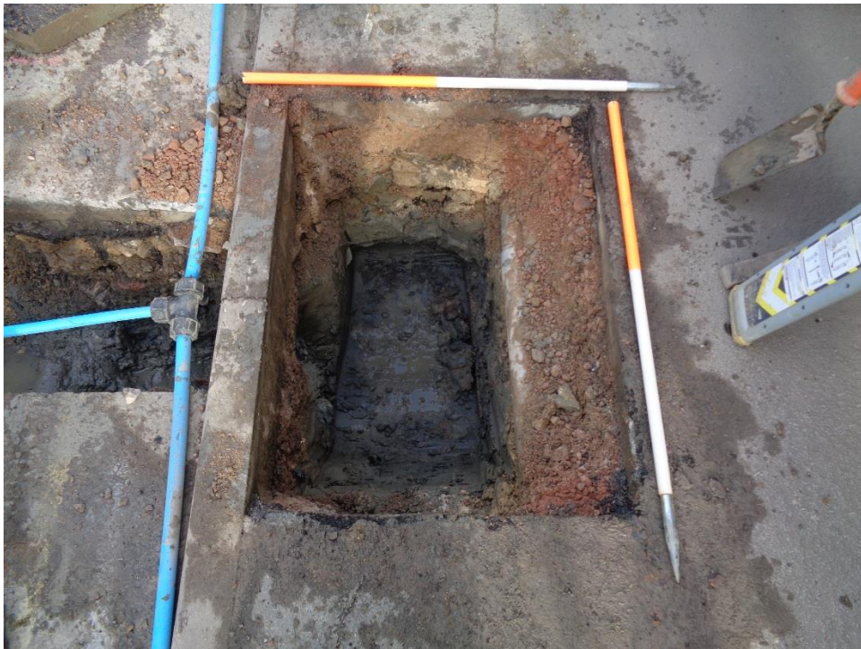
Plate 5: North Street: Earlier stone pavement (1005) sealing geological horizon (1004). SE-facing section.
