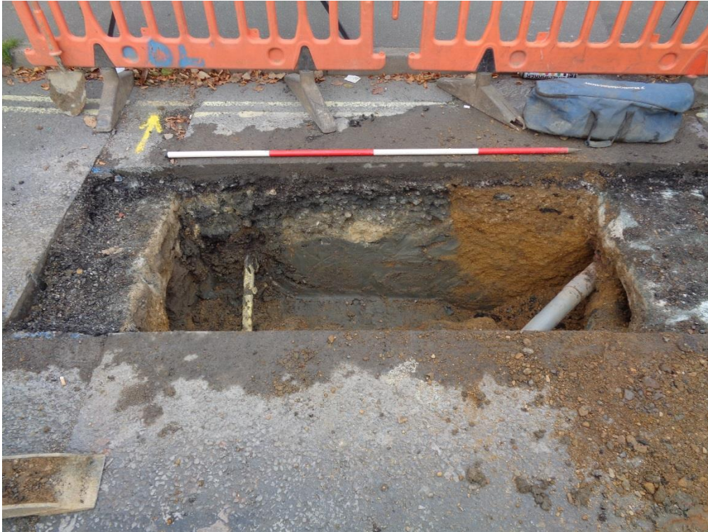
Plate 6: North Street: Possible rubble road surface (1006) sealing geological horizon (1004). SW-facing section.
