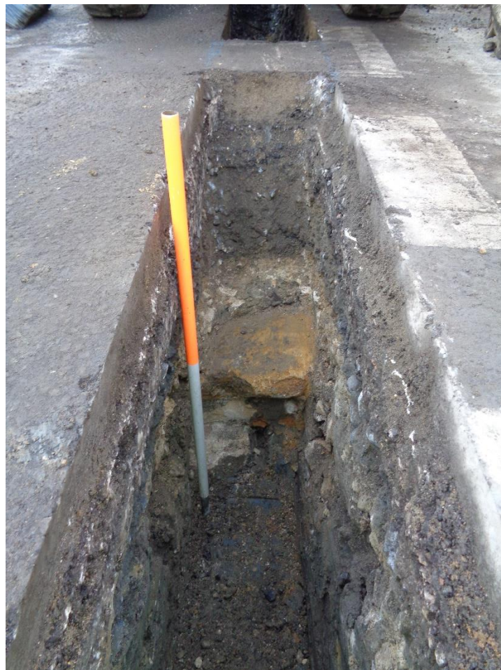
Plate 8: Road junction, masonry culvert (1009) of unknown date. View NW.
