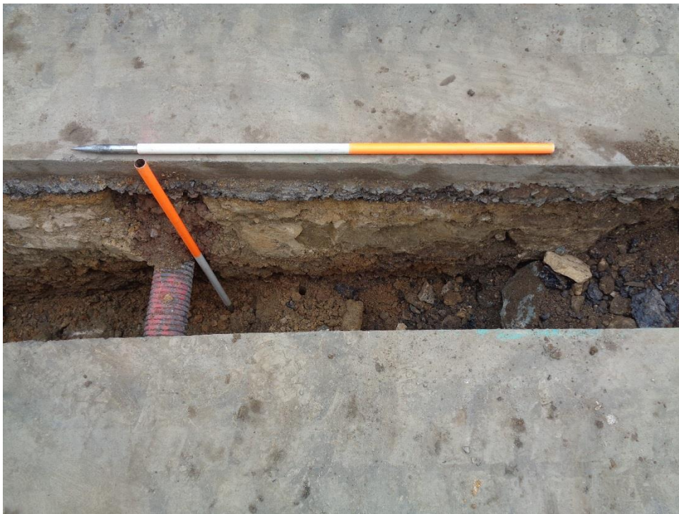
Plate 1: NW-facing trench section showing stone-lined culvert (0011)/[0013], sealing made ground (0006).
