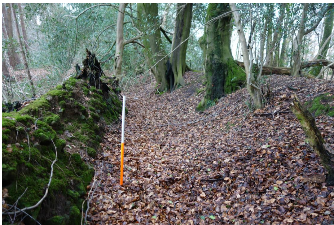
Plate 2: View SE along well-preserved section of revetment wall and ditch located about 200m SE of the site
