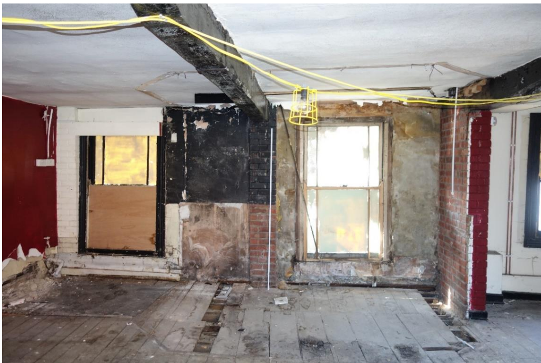
Plate 8: Internal view looking S within first floor of Block A showing brick pilaster marking construction break
