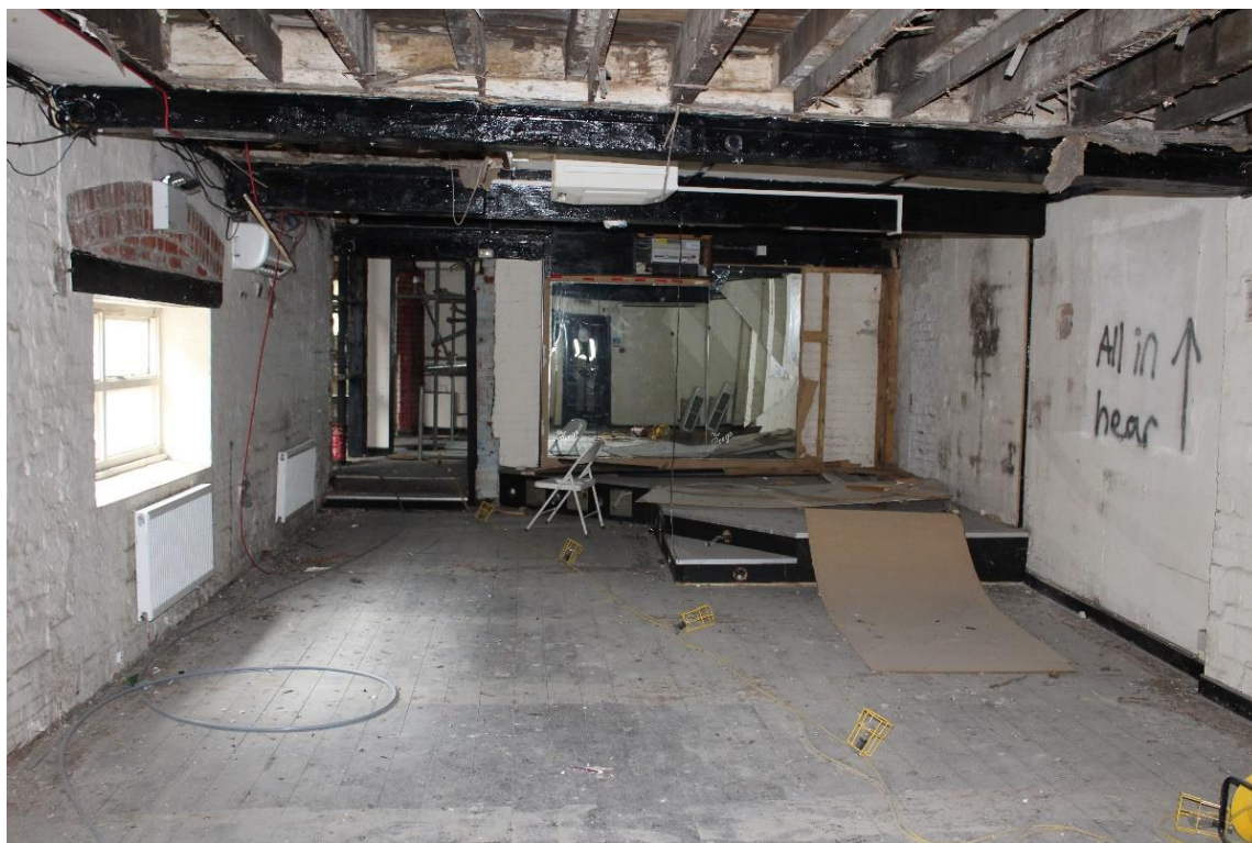
Plate 21: View looking S showing interior of Block C at first-floor level with exposed ceiling beams and joists and floorboards with horizontal indentations
