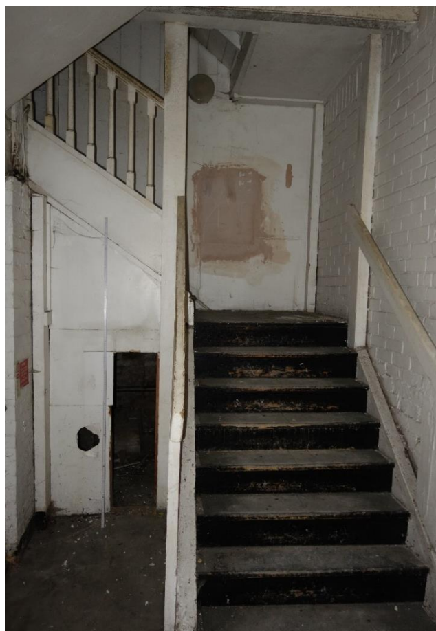
Plate 27: Internal view looking W showing dog-leg staircase with closed string, moulded handrail and stick balusters provides leading from ground floor to first floor within Block D
