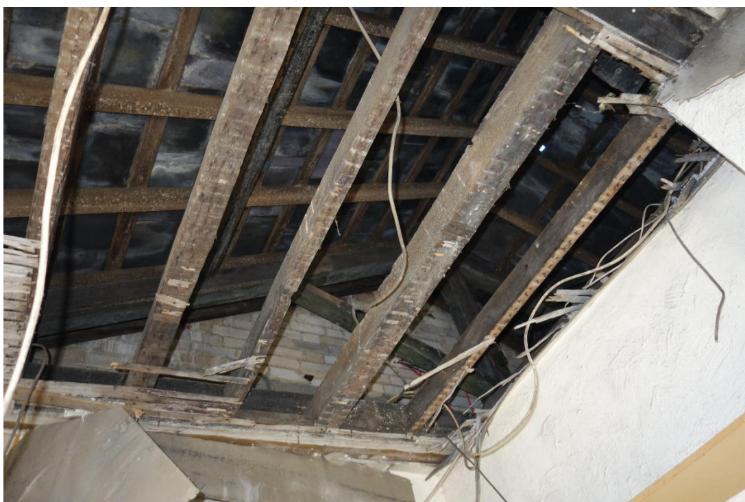
Plate 29: Internal view showing kingpost roof-truss within Block D
