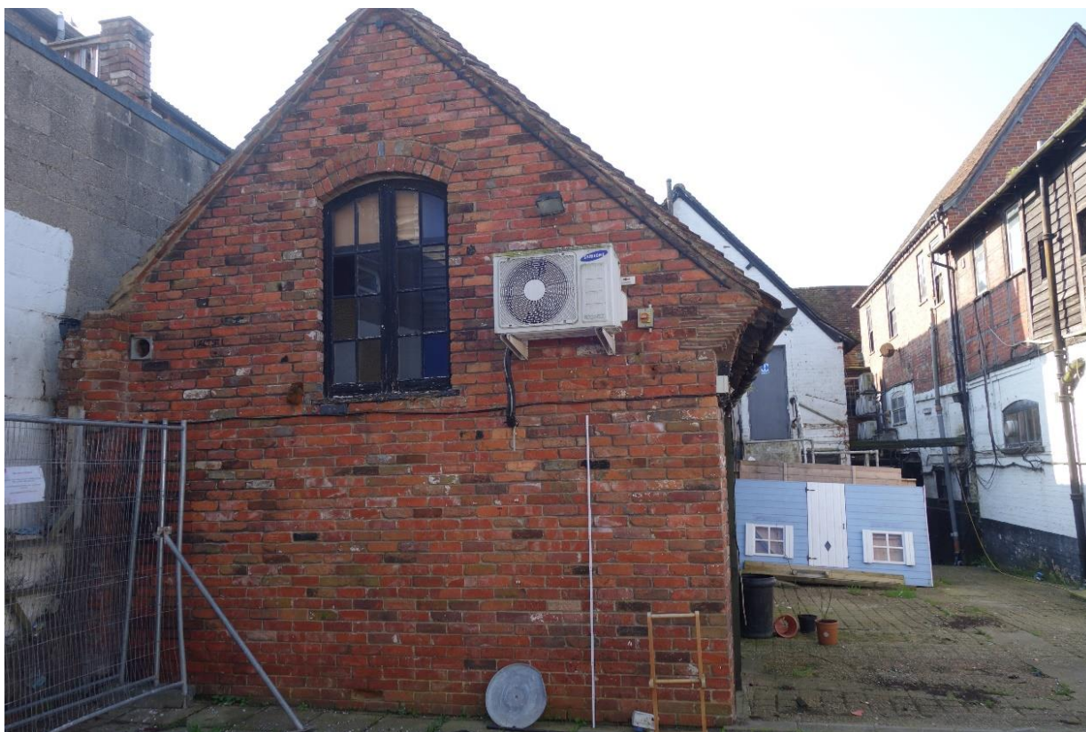
Plate 30: View looking S showing N-facing gable elevation of single-storey brick range (Block E) with segmental-arched casement window
