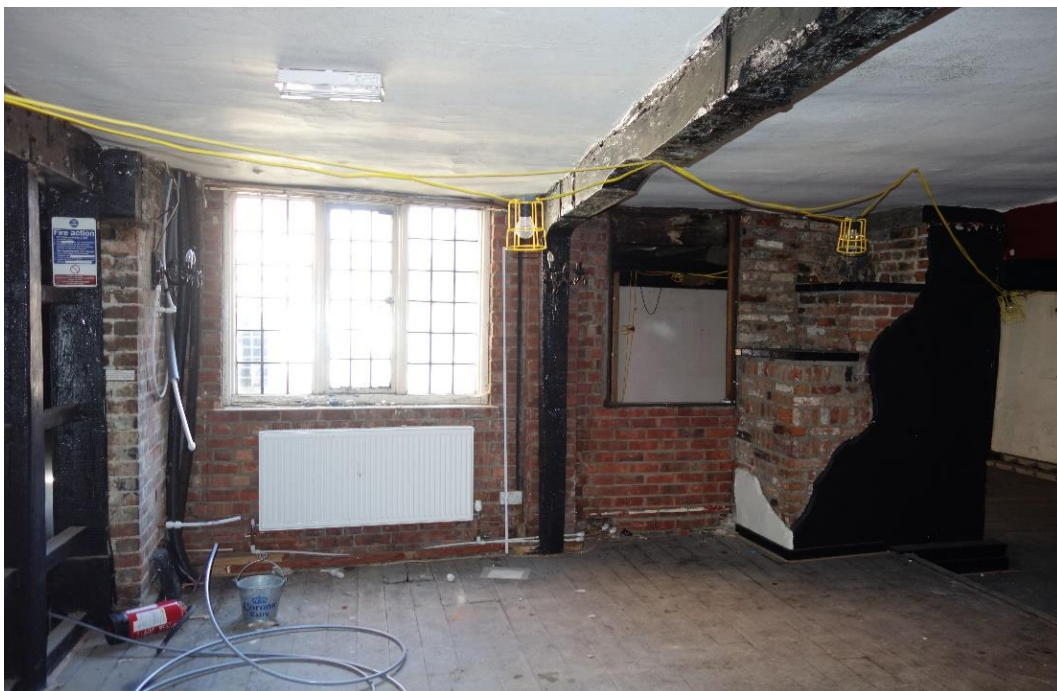
Plate 10: Internal view looking N within first floor of Block A showing modern brick wall with mullioned window, with remains of brick chimneystack visible to right of picture
