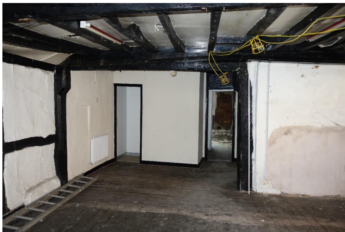
Plate 15: Internal view looking S showing southernmost bays of first floor within Block B with jowelled wall-posts and square-framed panels with lath-and-plaster infill
