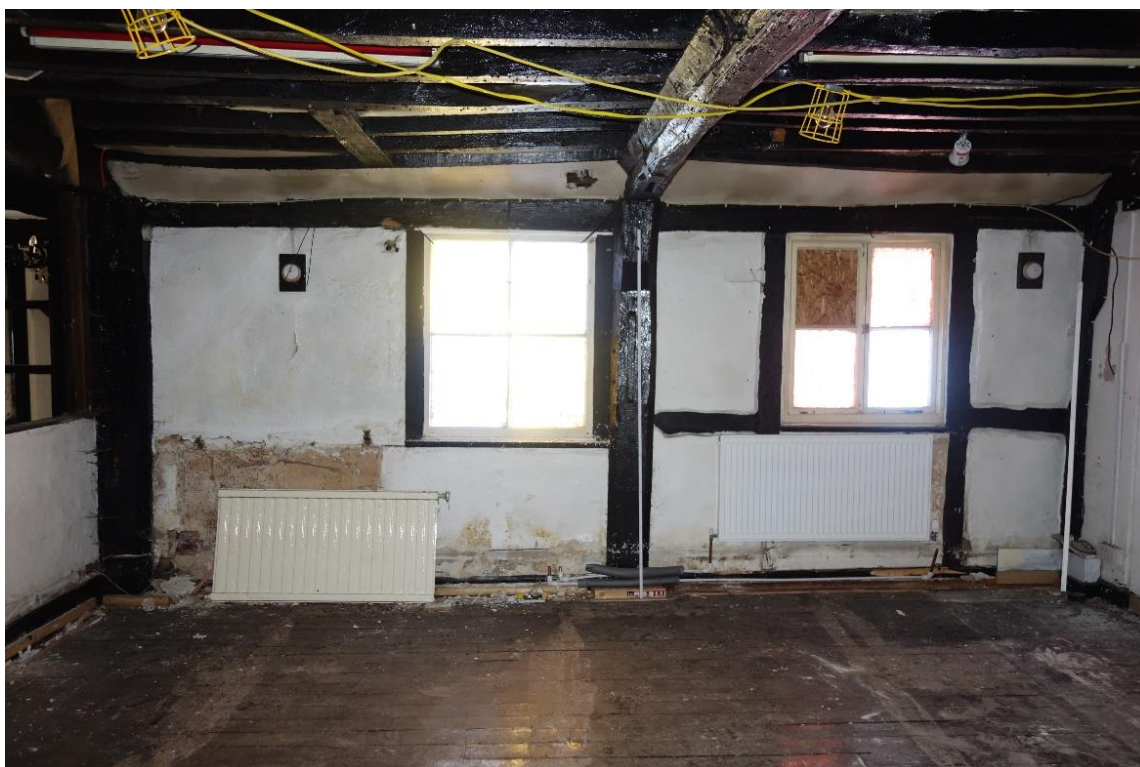
Plate 16: Internal view looking W within southernmost two bays of Block B showing W wall with timber-framed panels with brick and lath-and-plaster infill and modern casement windows, as well as exposed ceiling beams and wall-posts
