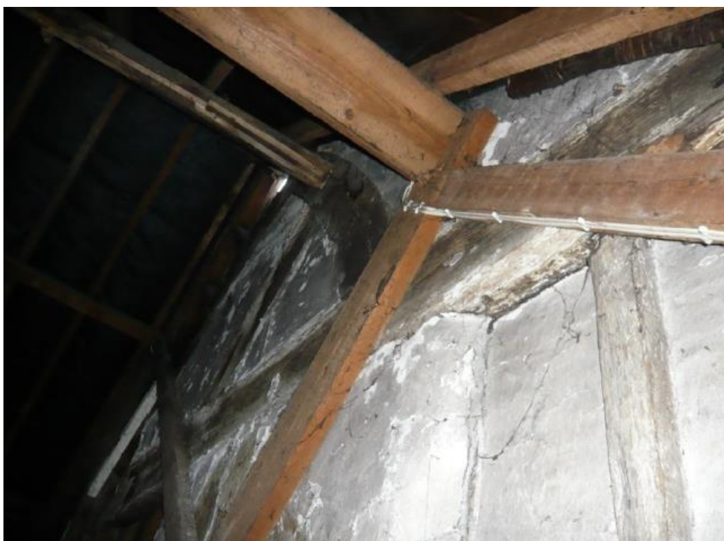
Plate 11: View within roof-space of Block A showing original timber-framing with scissor-braces above partition between fourth and fifth bays
