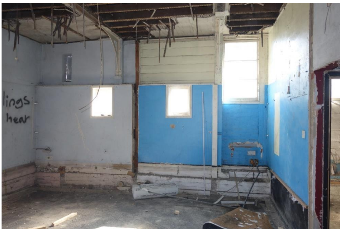
Plate 28: Internal view looking E within first floor of Block D showing ceiling beams supported by arched steel braces
