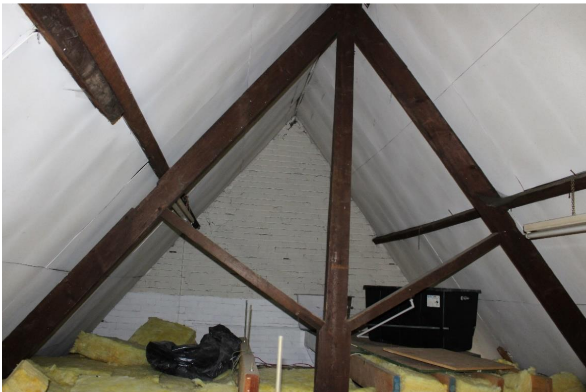
Plate 24: View showing kingpost roof-trusses within roof-space of Block C
