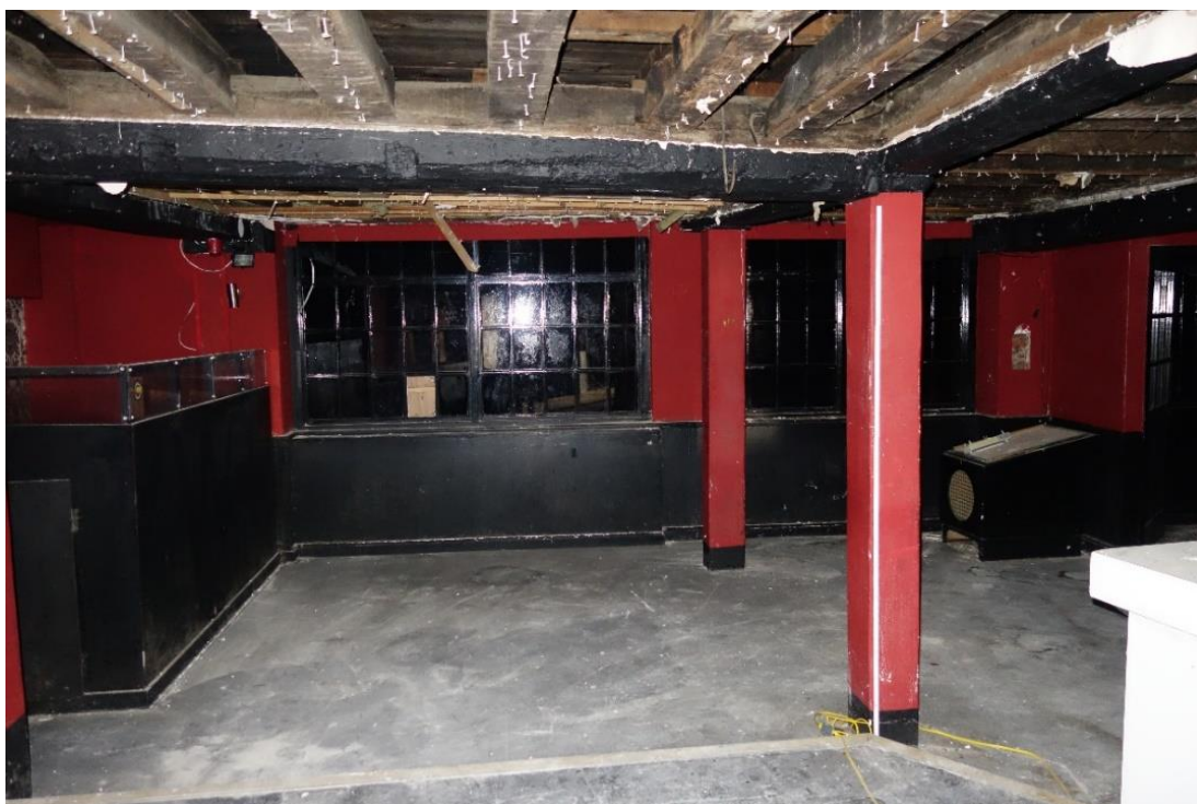
Plate 3: Internal view within ground floor of Block A showing exposed ceiling beams and joists and modern latticed glazing
