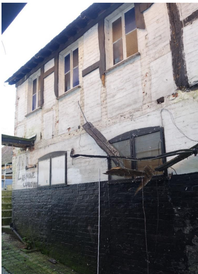
Plate 12: View looking NE showing W-facing elevation of Block B with segmental-arched windows at ground level and upper storey with false timber-framing
