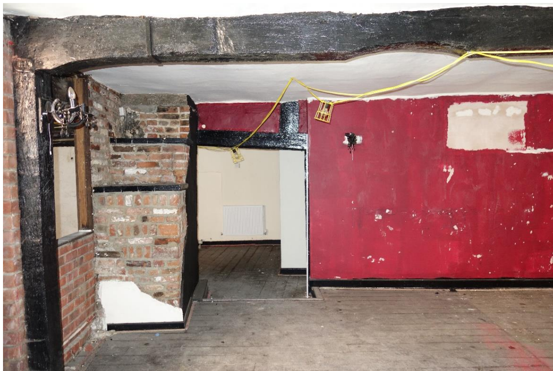
Plate 7: Internal view looking E showing partition wall between fourth and fifth bays within first floor of Block A, with exposed chamfered beam
