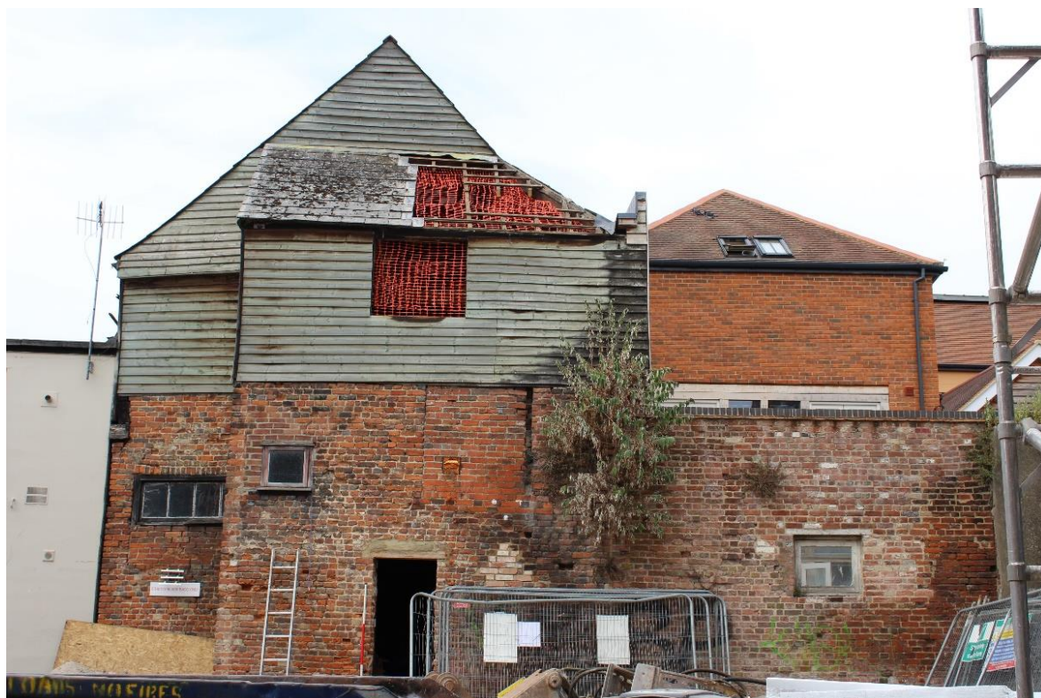
Plate 36: View looking W showing E gable end of Block G with eastern extension with catslide roof
