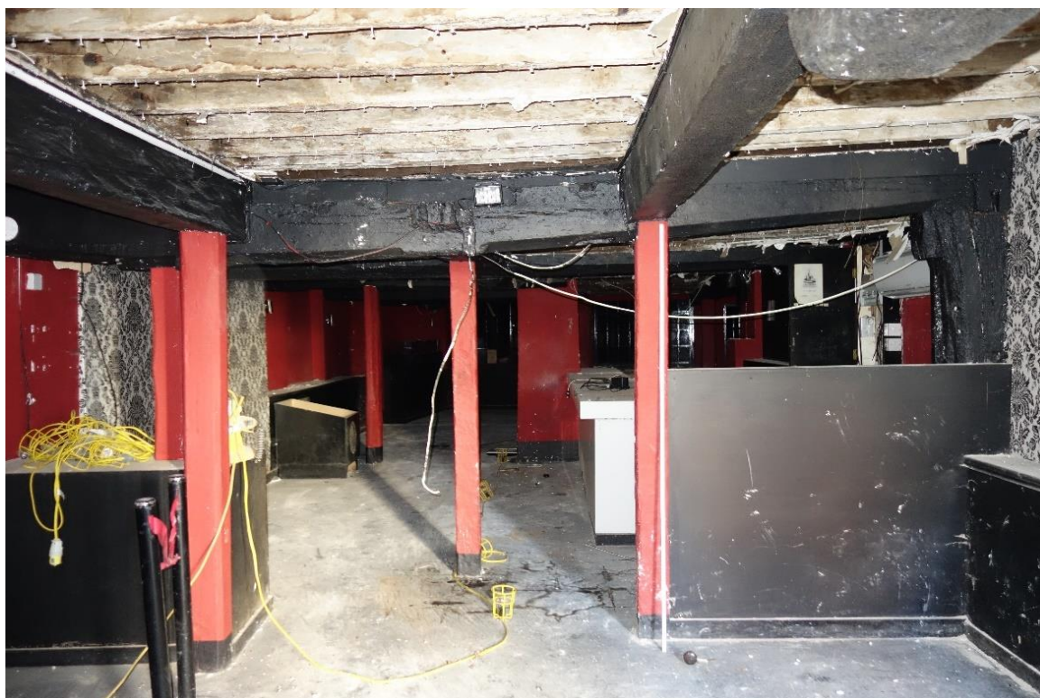
Plate 14: Internal view showing ground floor of Block B with exposed ceiling beams and joists
