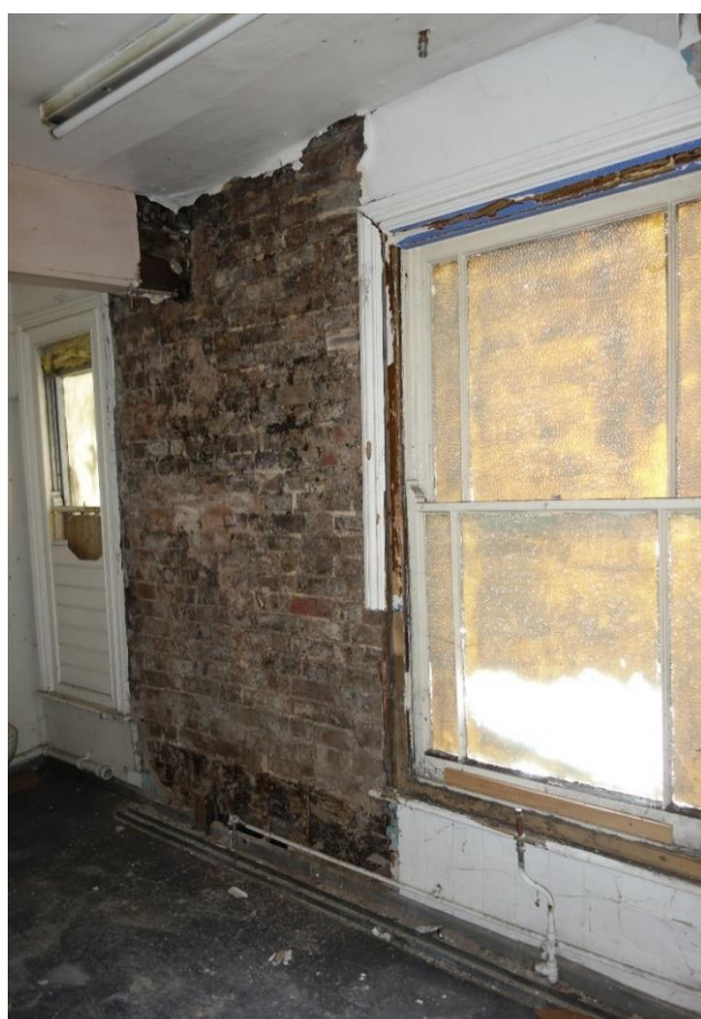
Plate 9: Internal view looking SE showing S wall within easternmost two bays of Block A with exposed brickwork
