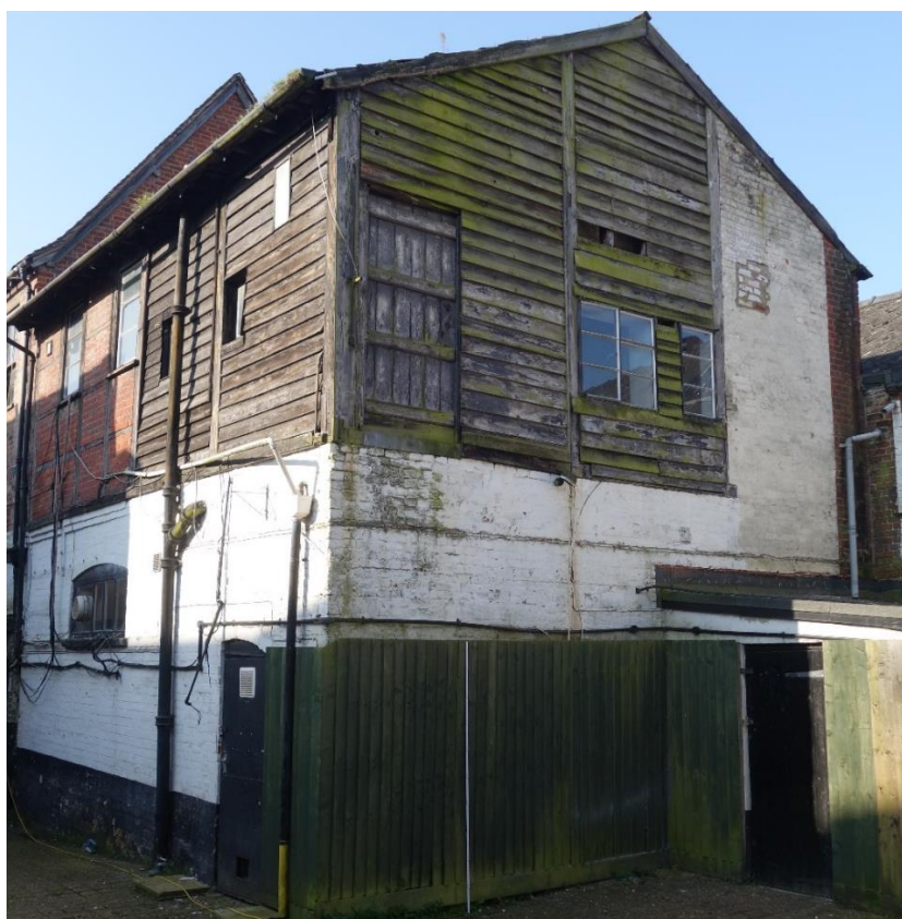
Plate 25: View looking SW showing two-storey range of brick and weatherboard construction (Block D) with weatherboard cladding in northernmost two bays
