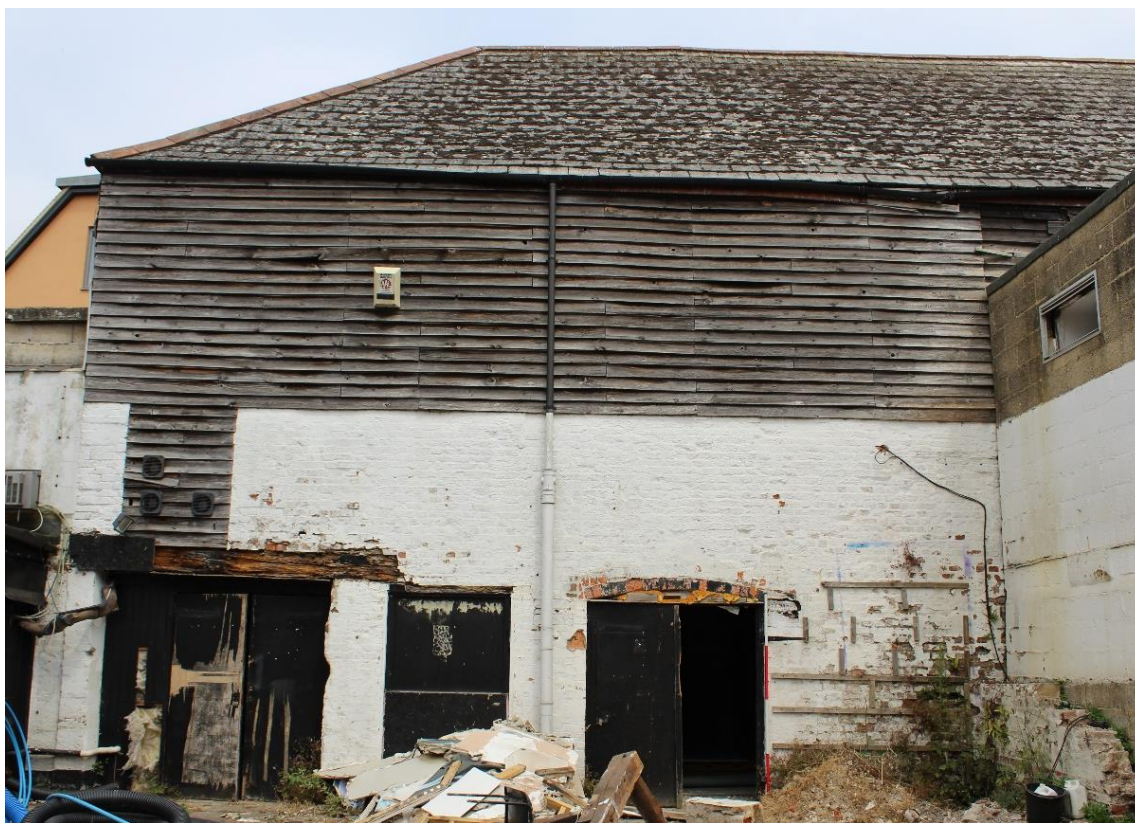
Plate 35: View looking N showing S-facing elevation of Block G, of brick and weatherboard construction
