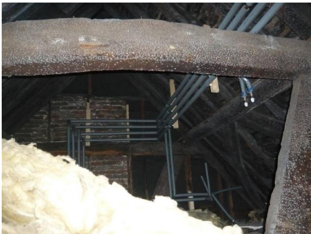
Plate 17: Internal view showing roof-space within southernmost two bays of Block B, with collar and tie-beam trusses of 16 th Century date
