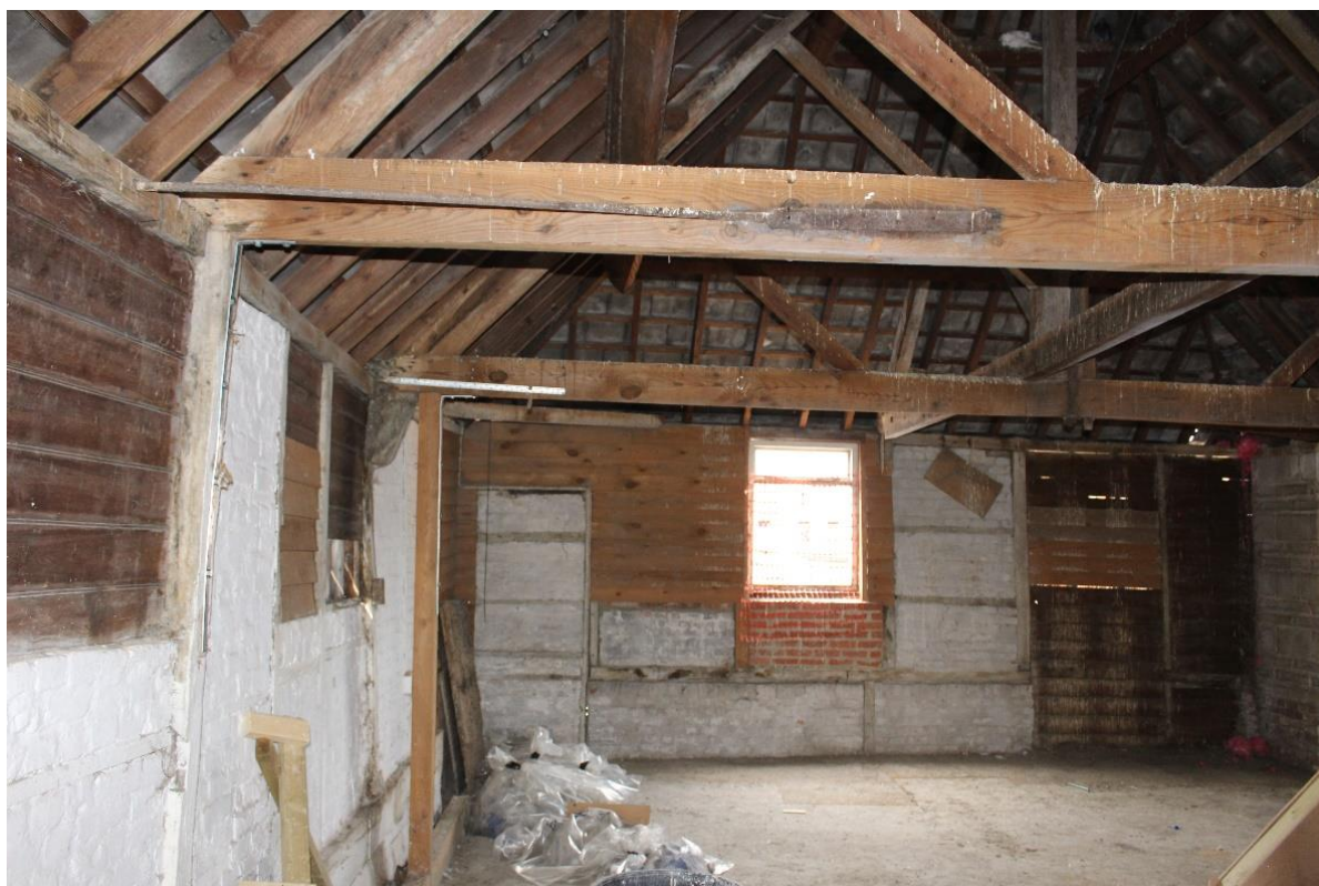
Plate 39: Internal view looking W showing upper floor of Block G with window openings in S wall (blocked by weatherboarding)
