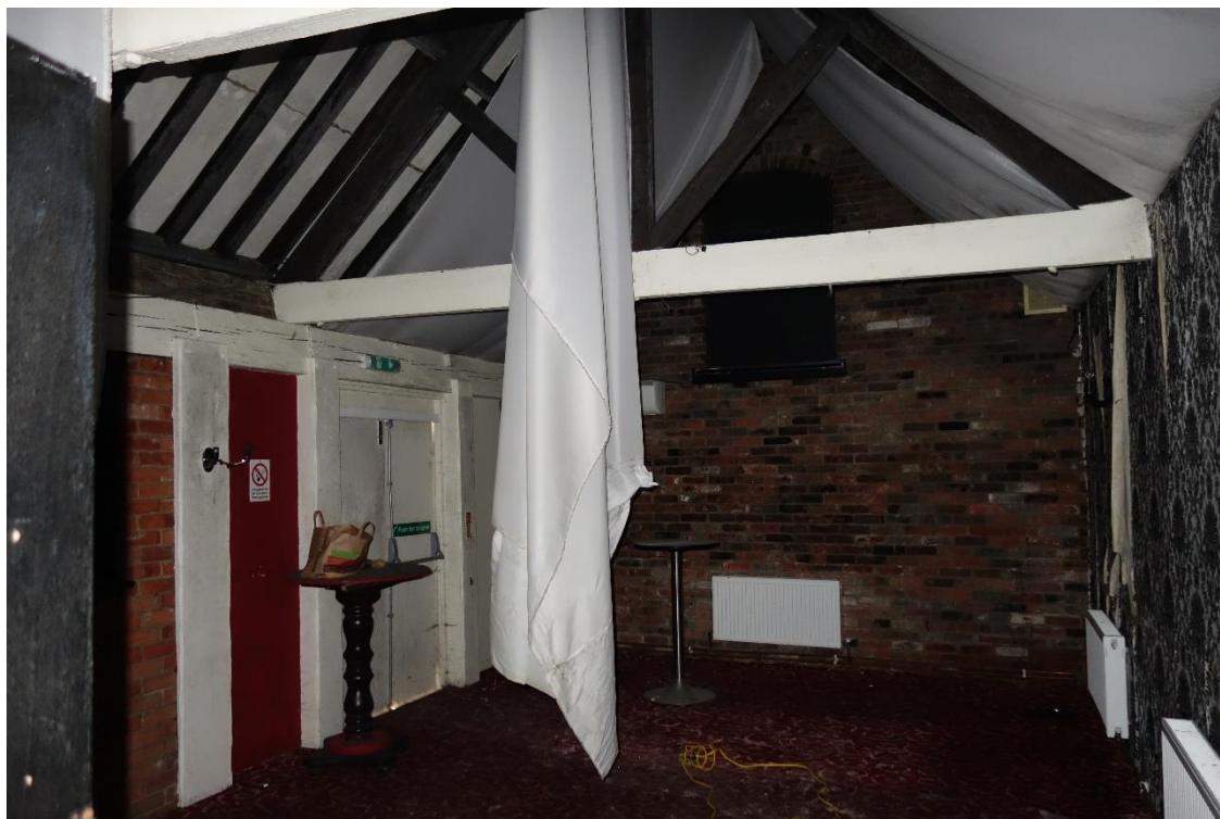
Plate 32: Internal view looking N showing kingpost roof-truss within single-storey range (Block E)
