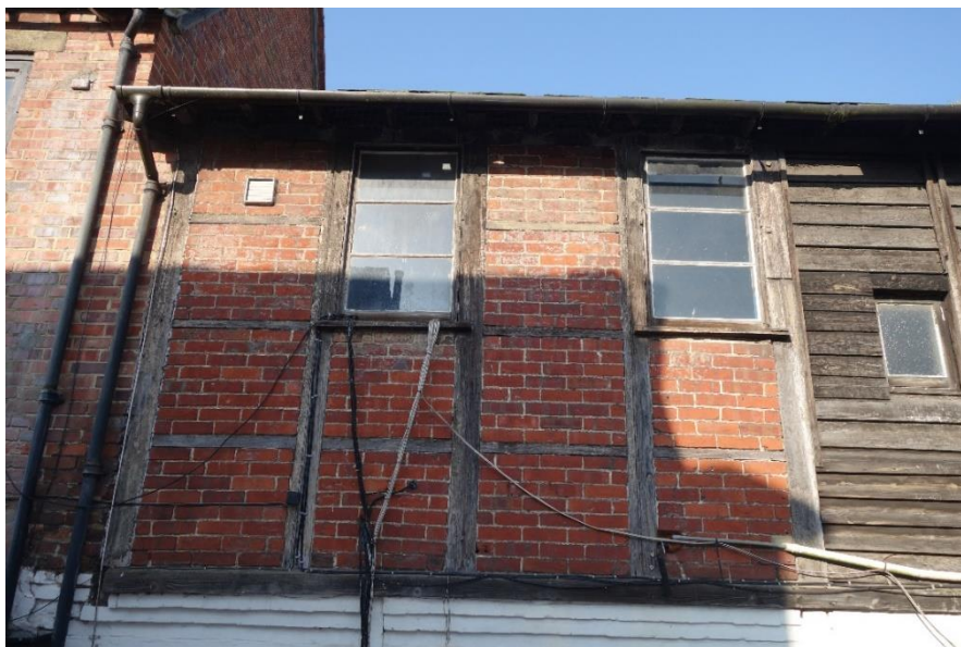
Plate 26: View looking W showing timber-framing with brick infill and casement windows in upper storey of Block D, with weatherboard cladding to right of picture
