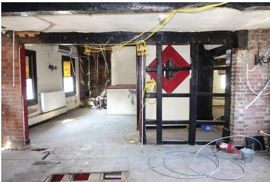
Plate 6: Internal view looking W within first floor of Block A showing modern timber-studded partition with beam above supported by brick wall-stubs
