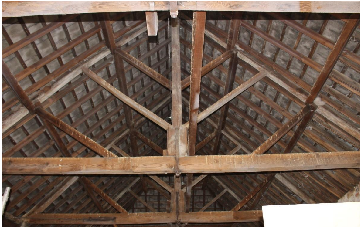
Plate 40: Internal view looking W showing kingpost roof-trusses in upper storey of Block G
