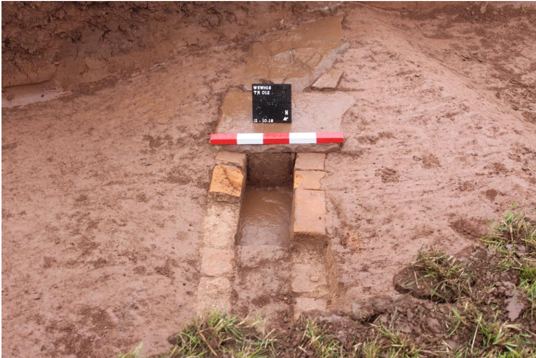
Plate 6: View SE of culvert [012005] within Trench 012
