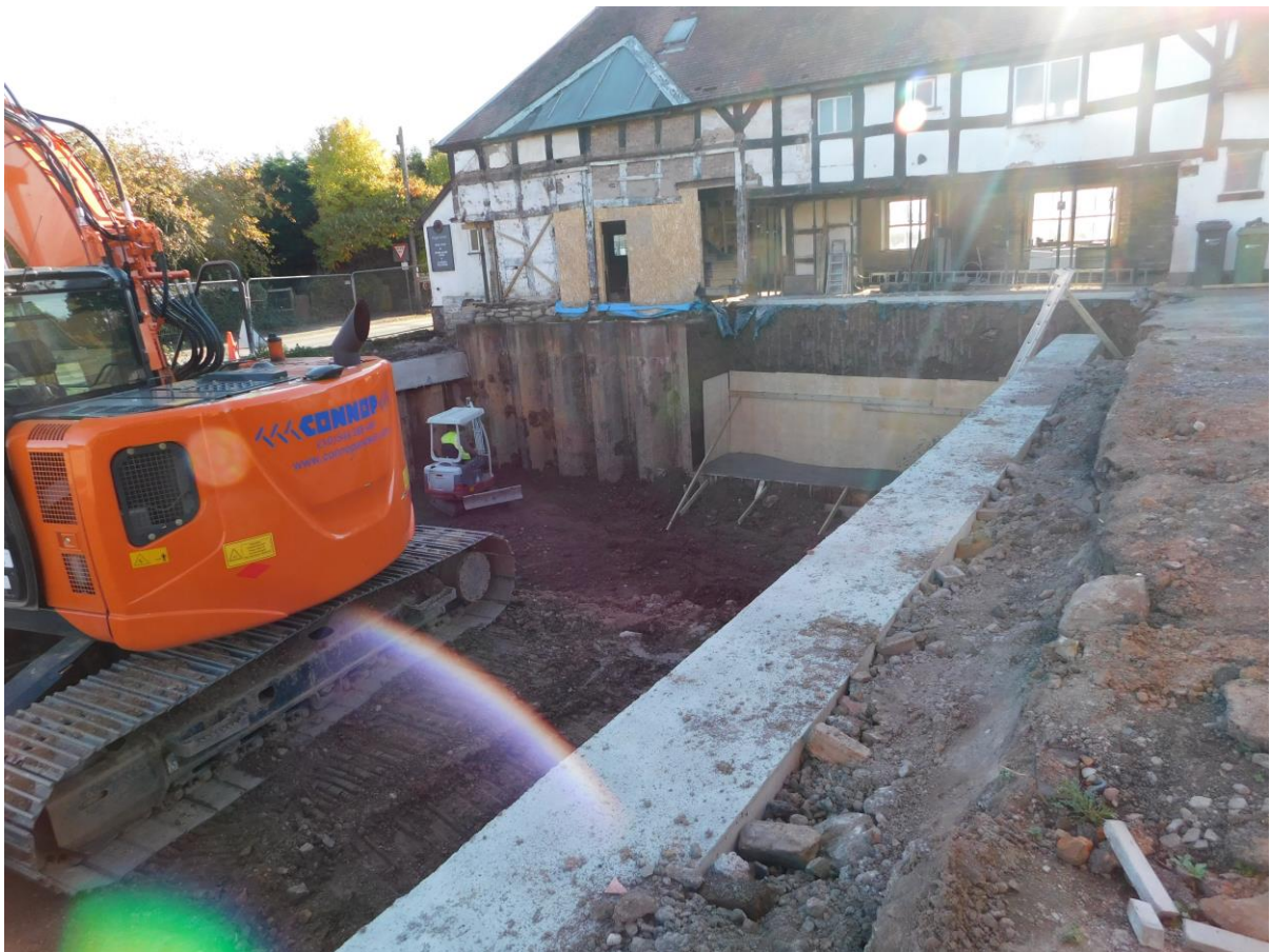
Plate 1: View SW of basement excavations nearing completion
