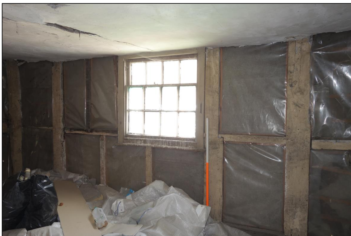
Plate 35: Internal view looking SW showing W wall of SW room at second floor level (No. 45) with later 4/8 sash window inserted, with a section of thin-scantled studding flanked by thick-scantled square panels
