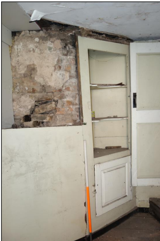
Plate 43: Internal view E showing detail of chimneybreast and recessed cupboard in NE corner of first floor room (No. 43) Plate 44: Internal view looking SE showing panelled door leading to staircase from first to second floor (No. 43)
