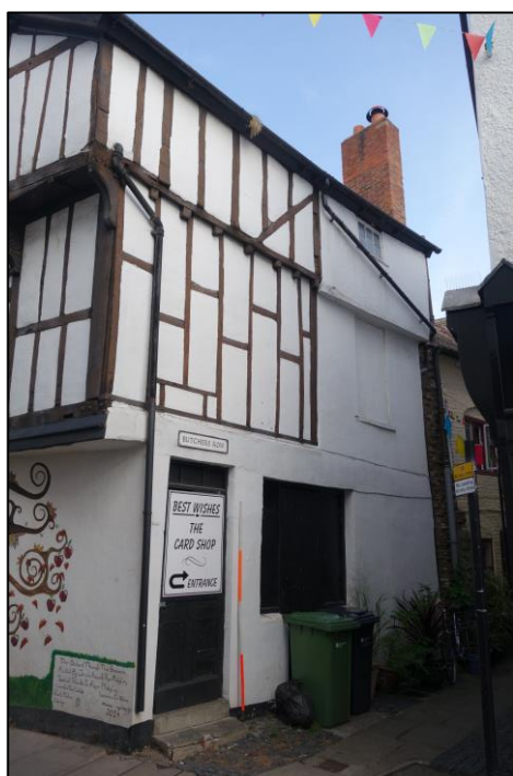
Plate 3: View looking NW showing rear elevation of No. 45 High Street with exposed thin-scantled timber framing Plate 4: View looking E showing W-facing frontage of No. 43 High Street with jettied storeys above 19 th century shop front
