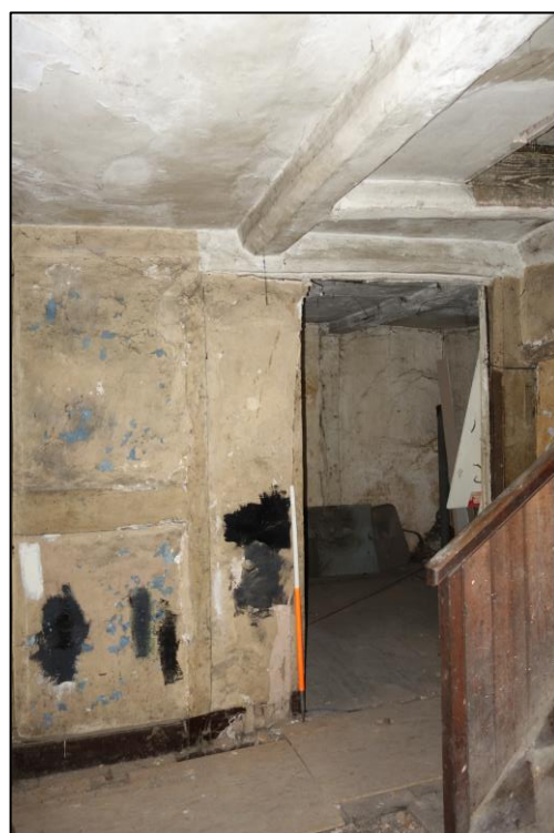
Plate 11: Internal view SW showing staggered partition wall between SE and SW compartments on first floor (No. 45) Plate 12: Internal view showing partition wall between SE and NE rooms on first floor (No. 45) showing square framed panels to left of picture and exposed ceiling beams
