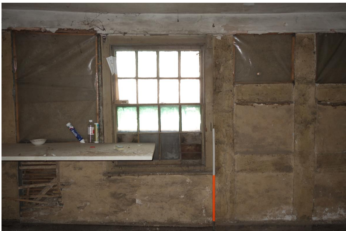
Plate 20: Internal view looking W showing 8/8 sash window in SW room on first floor (No. 45) flanked by thick-scantled square panels with lath-and-plaster infill
