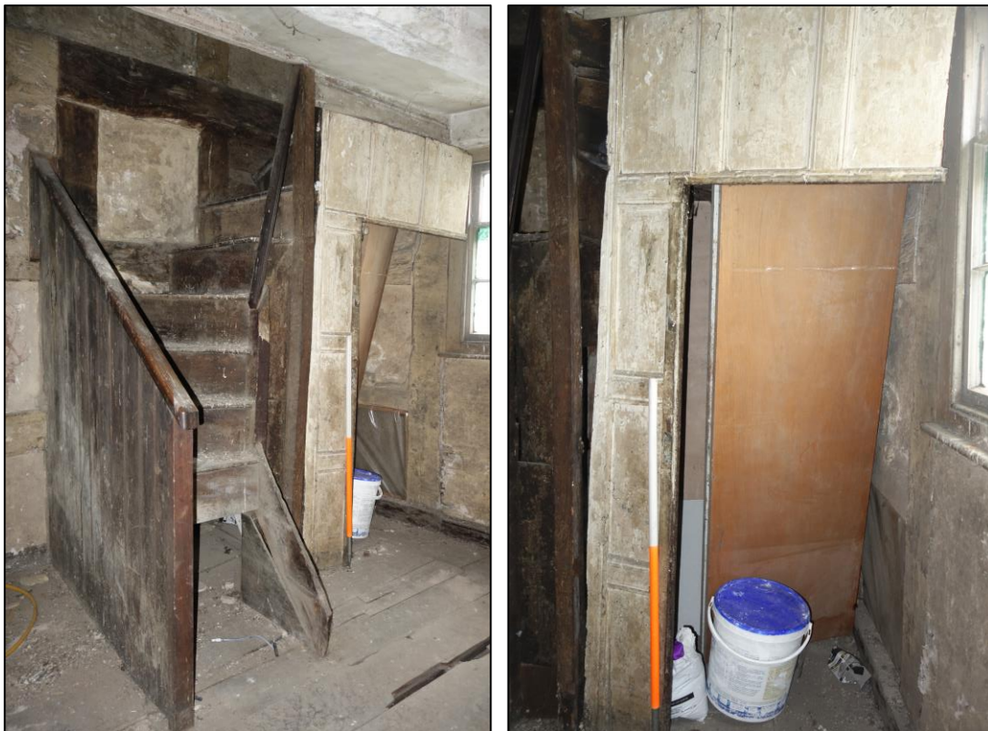
Plate 14: Internal view SE showing oak staircase leading up to second floor (No. 45) with oak panelling to right Plate 15: Internal view E showing section of oak panelling in SE room (No. 45) to right of staircase
