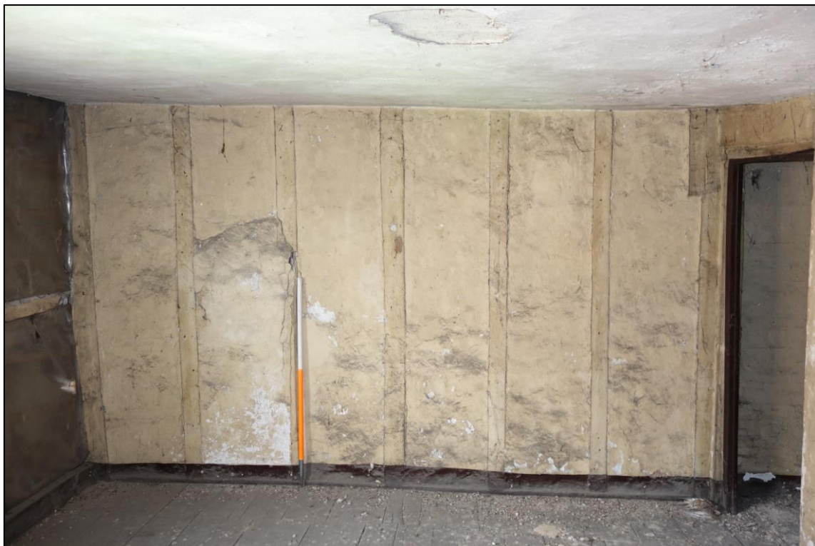
Plate 37: Internal view looking N showing N wall of SW room at second floor level (No. 45) showing close studded framing with thin scantling
