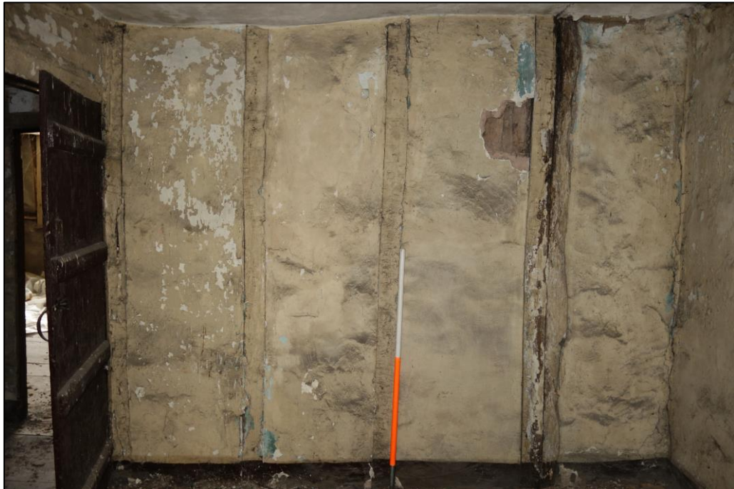
Plate 31: Internal view W showing close-studded framing in W wall of NE room at second floor level (No. 45)
