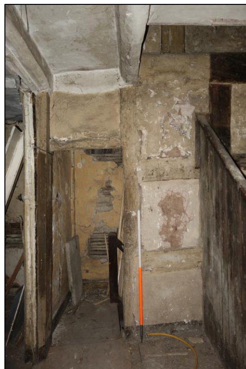
Plate 9: Internal view S across from first floor landing (No. 45) with thick-scantled square framed panels to right of picture Plate 10: Internal view E showing doorway inserted in timber framed wall leading from landing to first floor room (No. 45)
