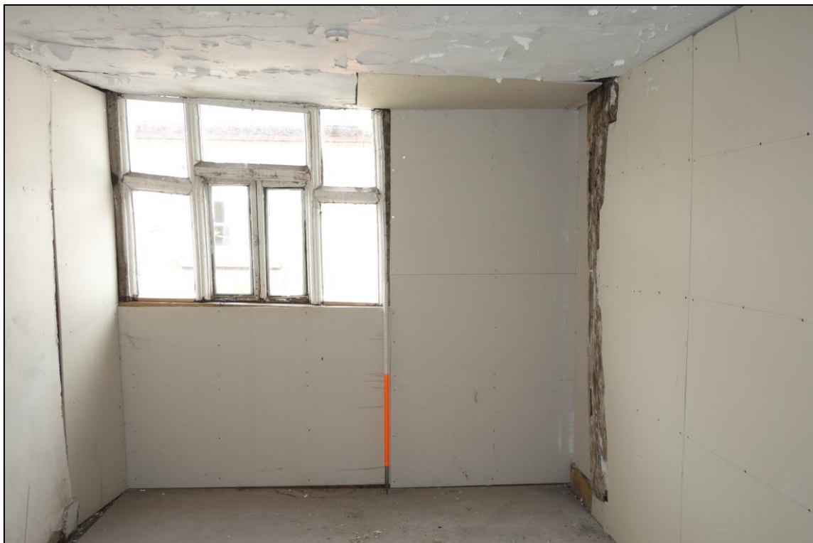
Plate 46: Internal view looking W showing westernmost bay of second floor room (No. 43) together with mullioned and transomed window with central casement
