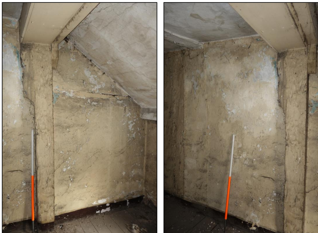
Plate 32: Internal view looking NE showing jowelled vertical post in N wall with infilled slots supporting transverse beam in easternmost bay of NE room at second floor level (No. 45)
