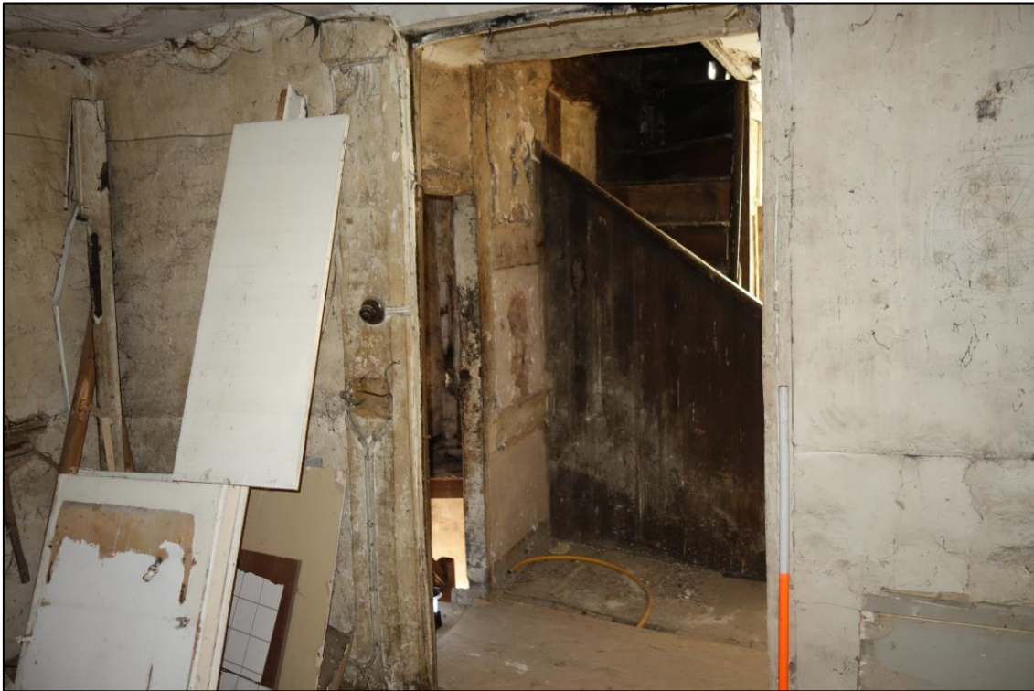
Plate 16: Internal view looking S showing doorway to NE room (with first floor landing in background) showing chamfered vertical post adjoining doorway, carrying ceiling beam
