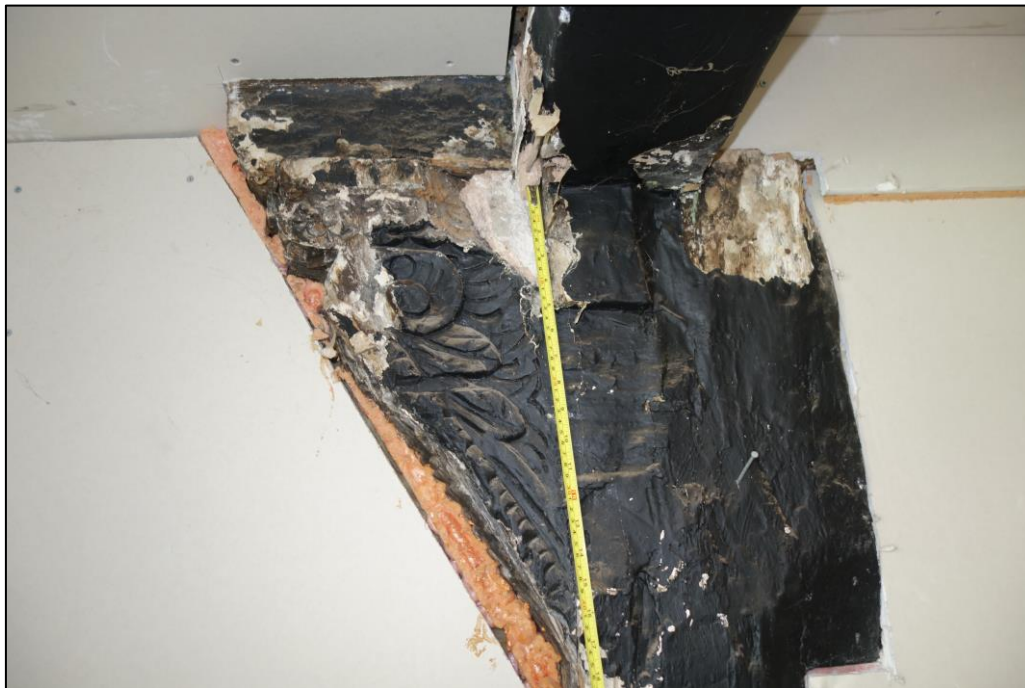
Plate 41: View showing detail of enriched scrolled bracket at top of vertical post in N wall of western bay of first floor room (No. 43)
