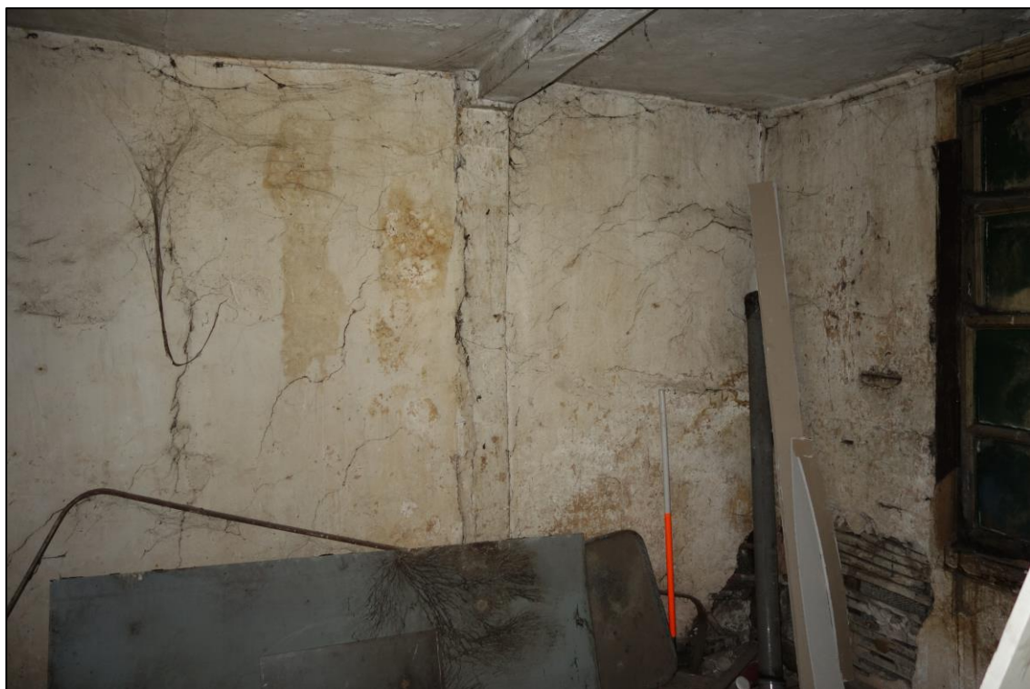
Plate 17: Internal view looking N showing vertical post and ceiling beam marking vertical construction break for easternmost bay (with 6/6 sash window to right of picture)
