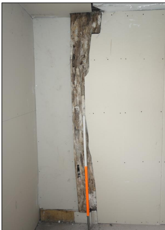
Plate 48: Internal view N showing jowelled vertical post with infilled slots within western bay of second floor room (No. 43) Plate 49: Internal view looking SE (No. 43) showing stairs leading from second floor room to roofspace
