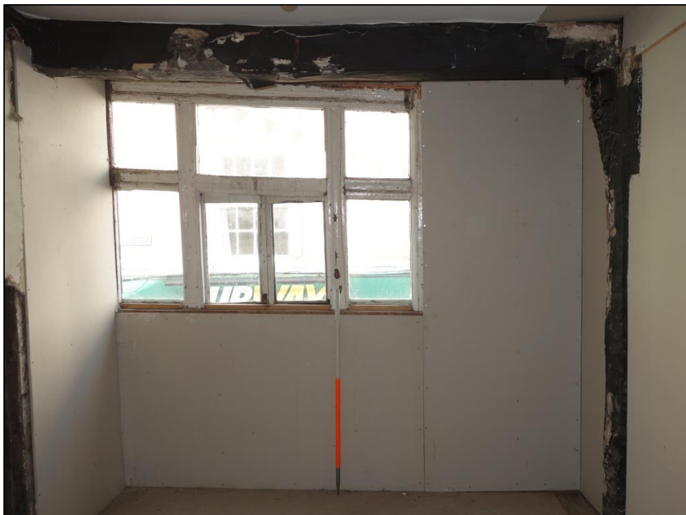
Plate 39: Internal view looking W showing westernmost bay of first floor room (No. 43) with mullioned and transomed window and exposed transverse beam carried on a jowelled vertical post (to right of picture)
