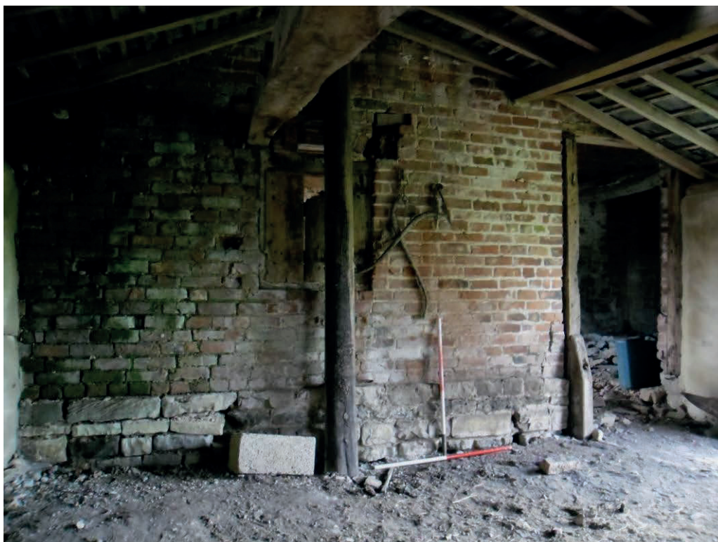
Plate 11: Internal view of horse engine house looking SE showing subsidiary tie beam inserted into segmental arched window in NW facing elevation of Barn A
