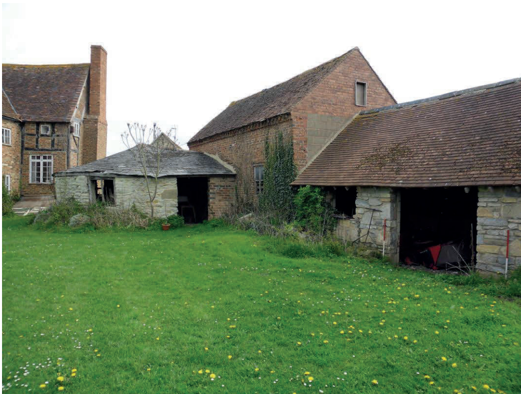
Plate 1: View looking ENE showing the NW facing elevation of Barn A with the attached horse engine house (Barn B) to the NW and the single storey stone barn to the SE (Barn C)
