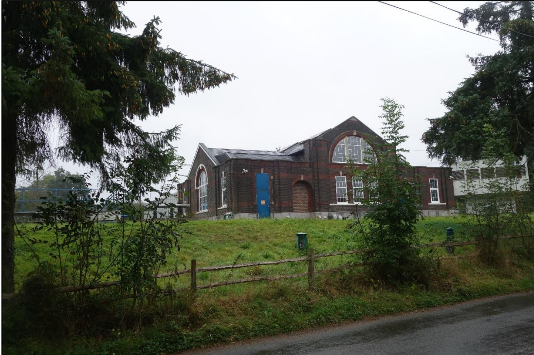
Viewpoint 1: View looking NE towards Forest Row Water Treatment Works
