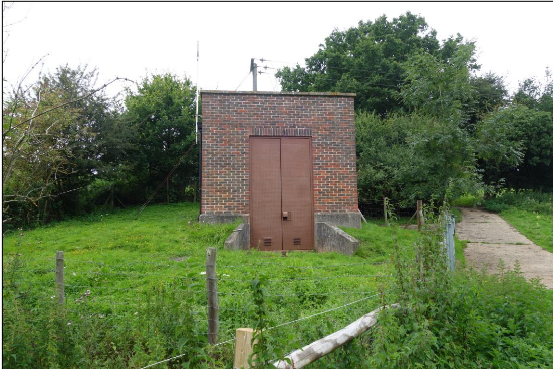
Viewpoint 1: View NE towards electricity sub-station adjacent to Sharnden Borehole, at SE terminus of route
