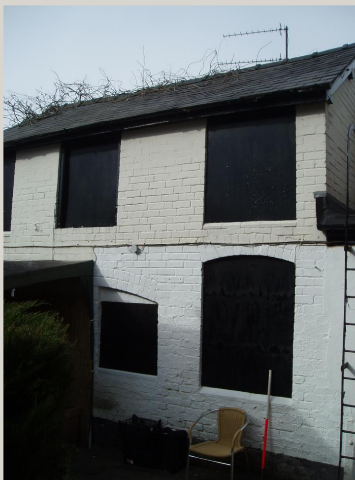
Plate 4: E elevation of Area 2 (formerly stables) showing bricked-up double-door (partially obscured by covered passageway)
