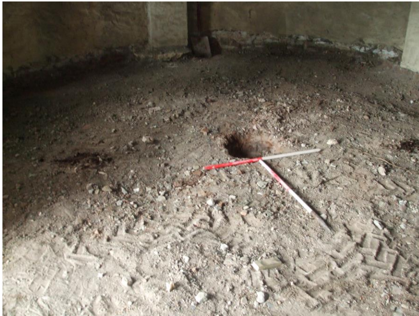
Plate 3: View looking NW showing interior of engine house following reduction of ground levels, with circular slot for the horse engine drive shaft in the centre of the turning circle
