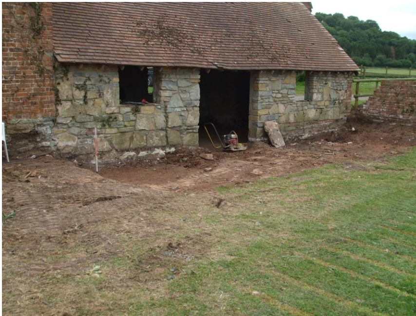
Plate 5: View looking SE showing reduction of ground levels immediately adjacent to the NW facing elevation of single storey barn structure (Barn C)
