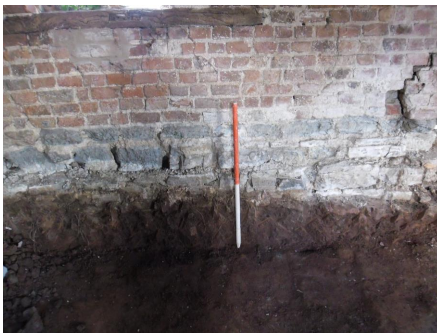
Plate 1: Internal view looking NW showing the foundation courses of the NW wall of the two-storey barn and the deposits revealed in section beneath the wall
