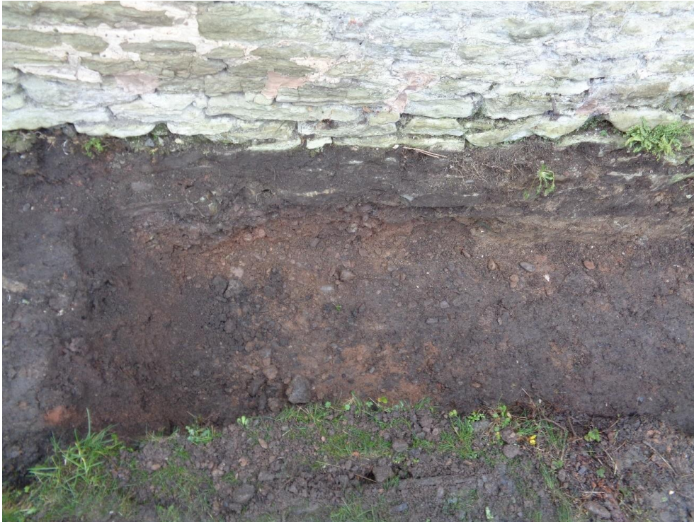
Plate 3: Drainage Trench 001 showing masonry foundations, topsoil (03001) & natural (003002).
