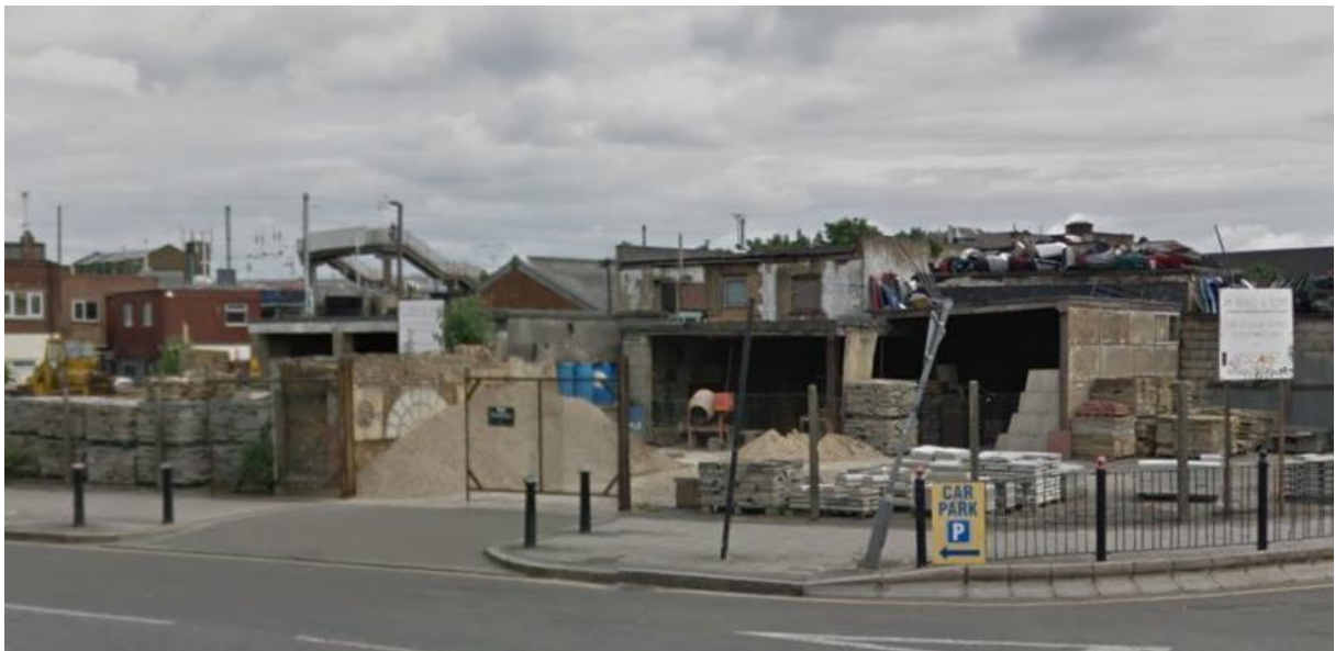
Plate 2: View looking NE showing the site at Nos. 1-2 Hepscoth Road, Hackney Wick, currently occupied by a stone merchant's premises
