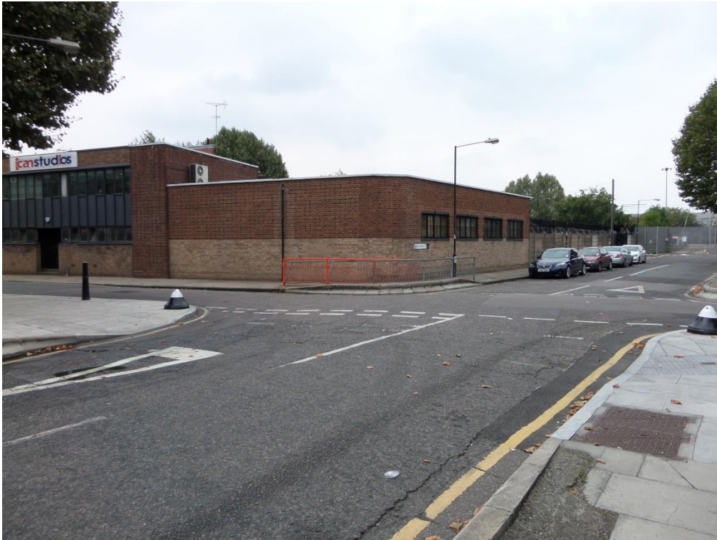
Plate 3: View looking NNW of two-storey building adjacent workshop at corner of Monier Road and Smeed Road
