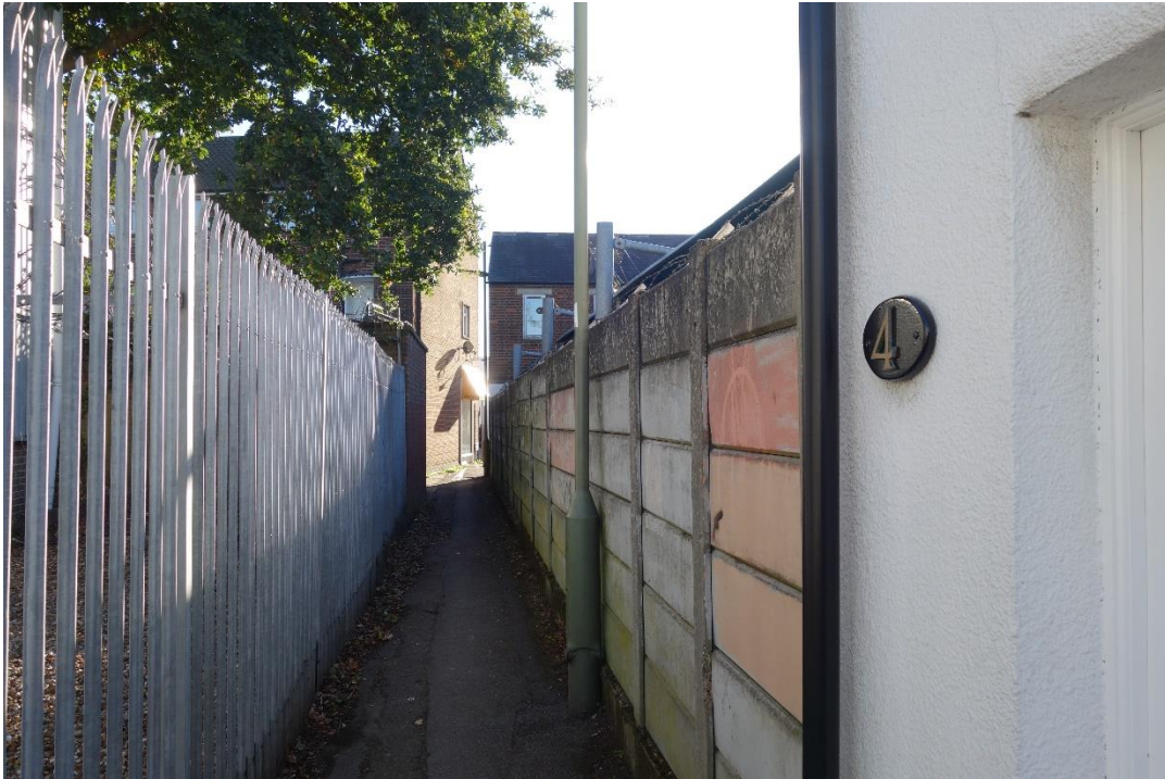
Plate 2: Current east facing view from along Nursery Row towards No. 151 (Border 2018)
