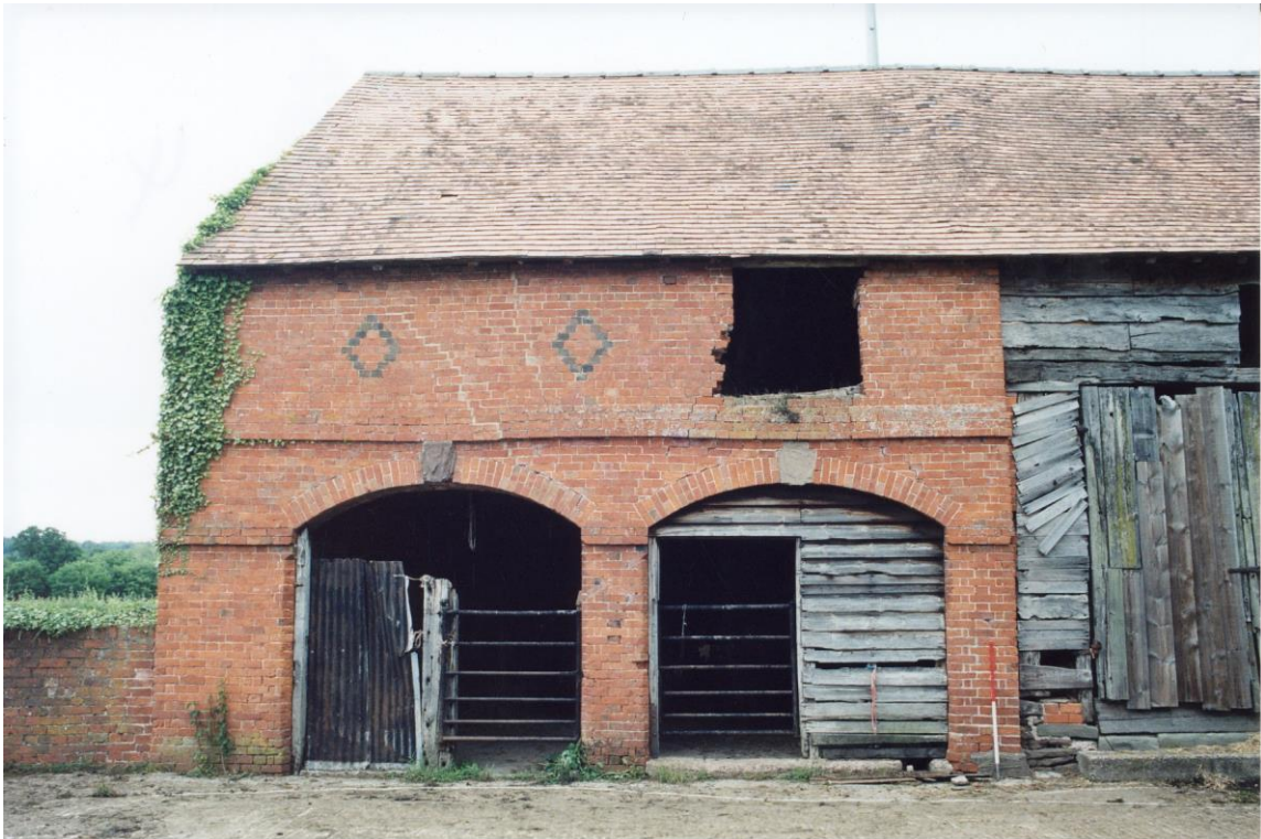
PLATE 4 BARN I SHOWING 19TH CENTURY EXTENSION
