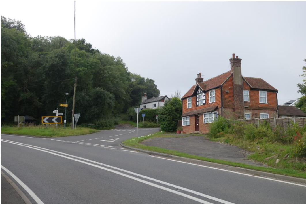
Viewpoint 41: View looking SSW along A267 road towards former Bicycle Arms public house of late 19 th century date
