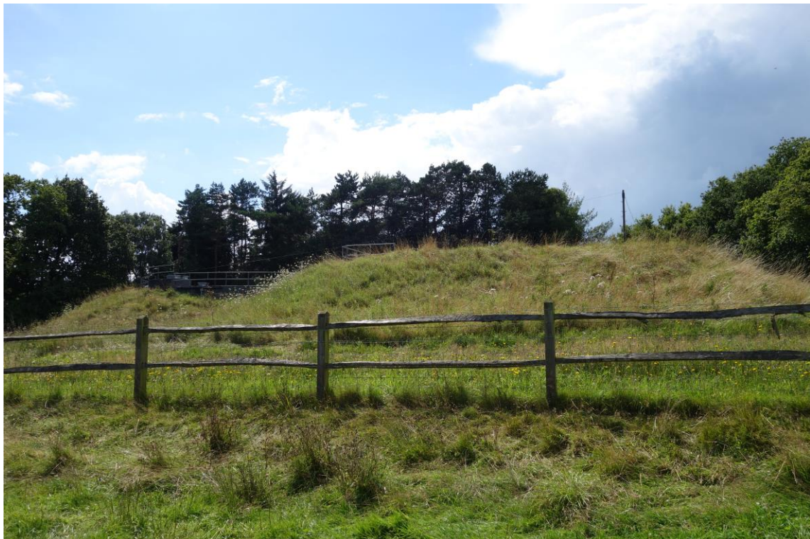
Viewpoint 46: View looking SSW towards modern covered reservoir on summit of Cottage Hill
