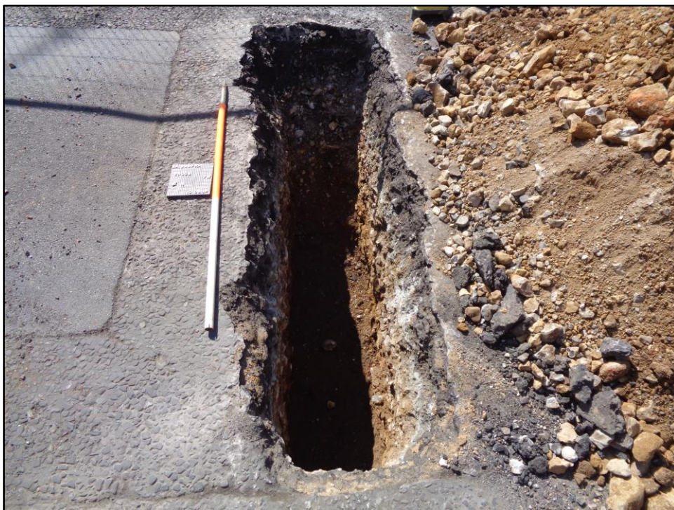
Plate 3: Overview of Trench 002, looking SSW with 1m scale
