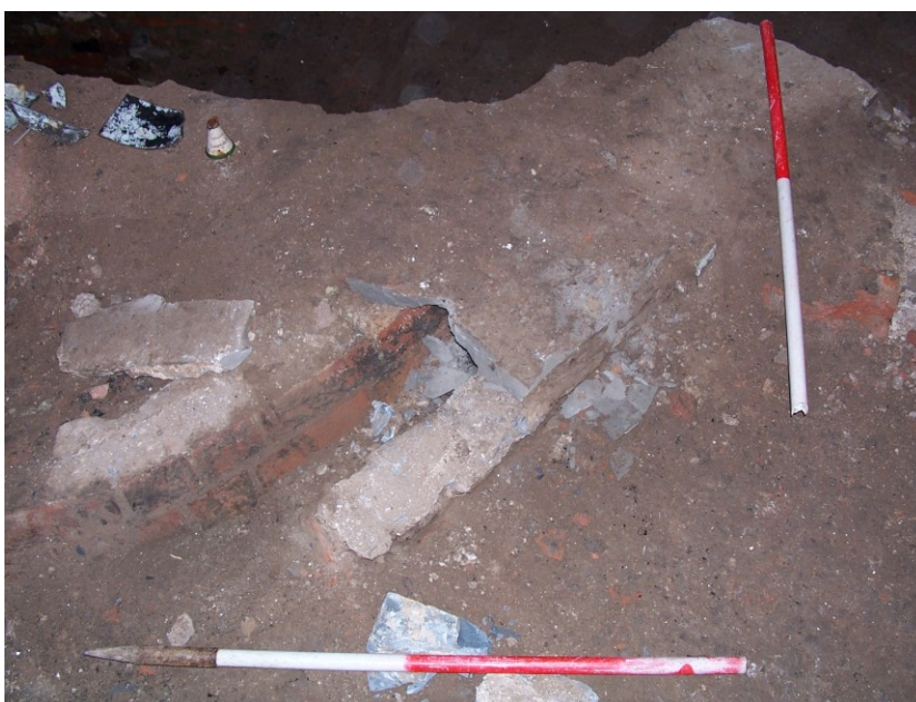
Plate 6: Internal view looking SE showing brick-lined drain [209] with remains of stone capping (212)
