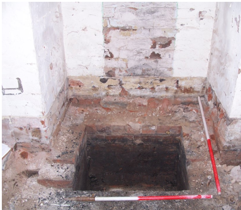
Plate 5: Internal view looking W showing rectangular brick shaft [205] at base of hearth at W end of building
