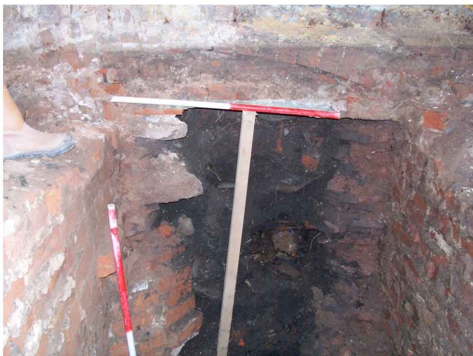
Plate 8: Internal view looking N showing segmental arched doorway (220) set into N wall of building
