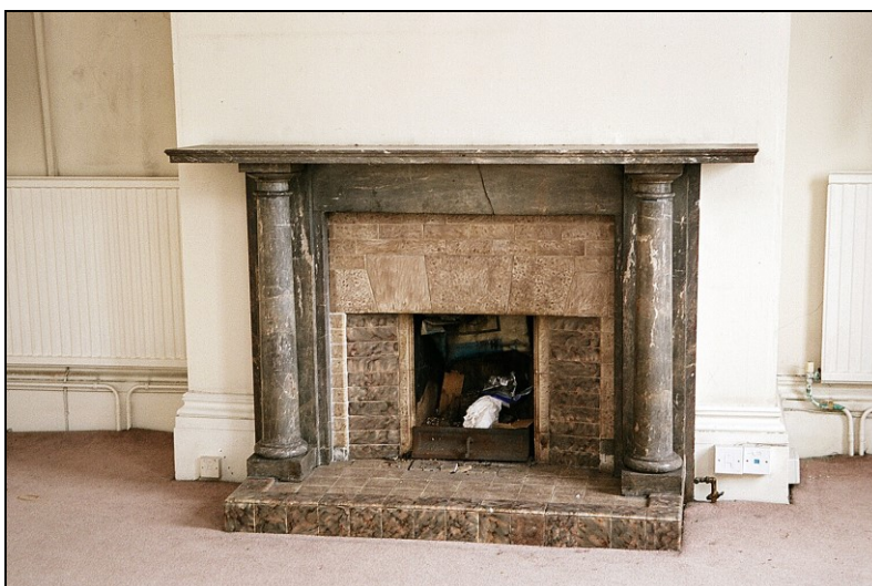
Plate 56: View showing Art Deco ceramic fireplace and recessed tiled hearth of 1930s date set within marble surround and mantelpiece supported by Tuscan columns
