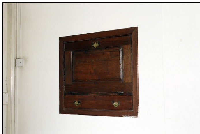
Plate 59: View showing mid-late 19 th century pantry hatch in dining room
