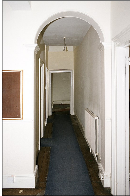
Plate 58: View N down first-floor passageway with round-headed archway supported by pilasters in foreground
