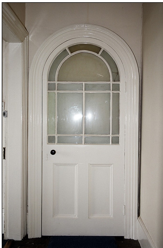
Plate 46: View showing round-headed, partially glazed door with semicircular oversight within a fluted architrave dated to c.1830-40
