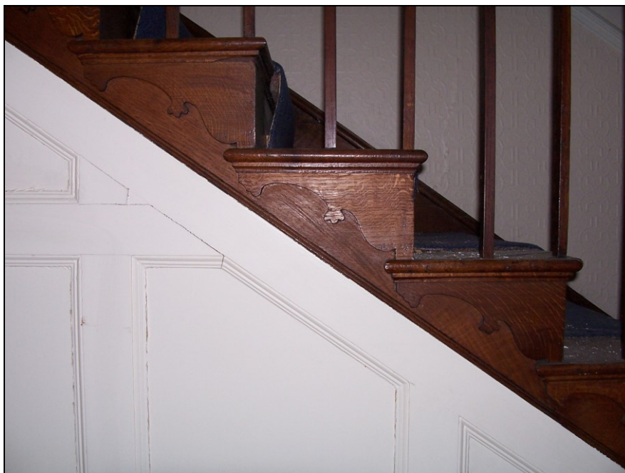
Plate 27: View showing detail of staircase showing applied brackets with plain Vitruvian scroll motif
