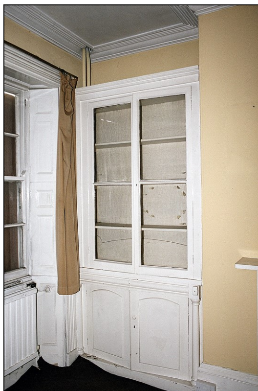
Plate 30: View SE showing two-tiered panelled cupboard of c.1830-40, the upper portion glazed while the lower portion is decorated with Tuscan columns
