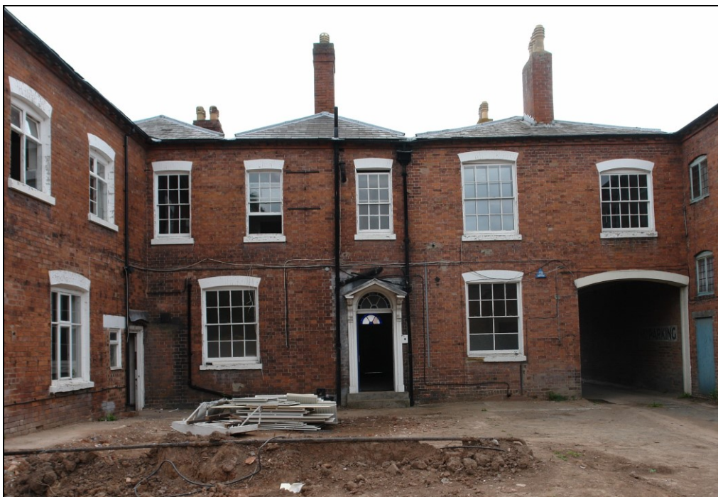
Plate 8: View E showing the rear elevation of No. 38 South Street
