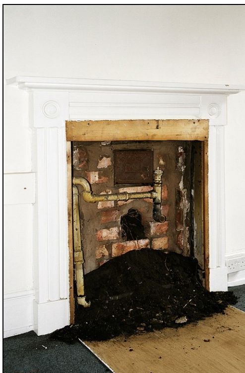
Plate 62: View showing wooden mantel and fluted fireplace surround with paterae
