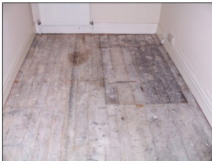
Plate 37: View S showing wooden hatch leading to cellarge
