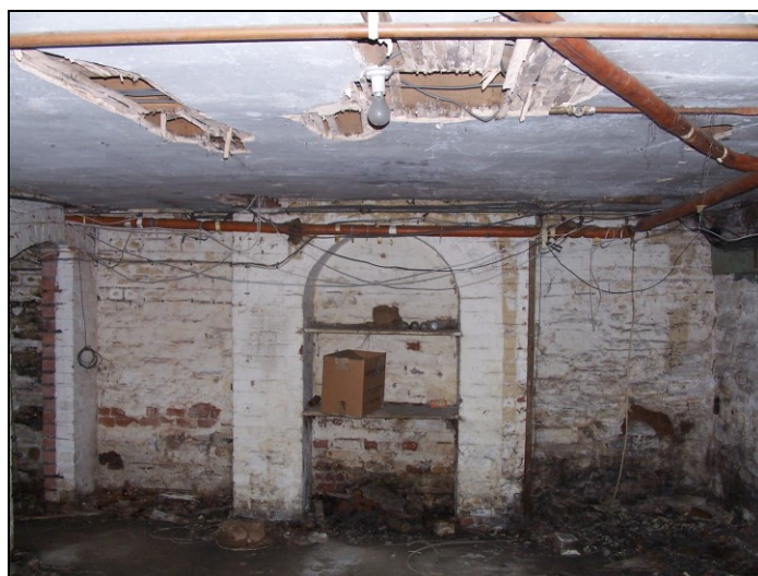
Plate 21: View W showing round headed alcove at W end of 'Spirit Stores'
