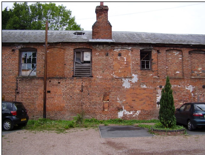
Plate 17: View N from Foxes Court showing central part of S-facing elevation of outbuilding range with partially blocked segmental-arched door and window openings at ground- and first-floor level
