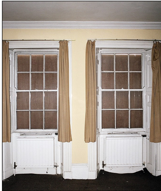
Plate 31: View E showing two 12-pane double-hung sash windows set within shouldered, fluted architraves with foliage decoration in the spandrels
