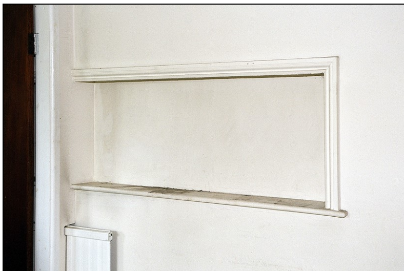
Plate 65: View NW showing long rectangular recess for wall cupboard
