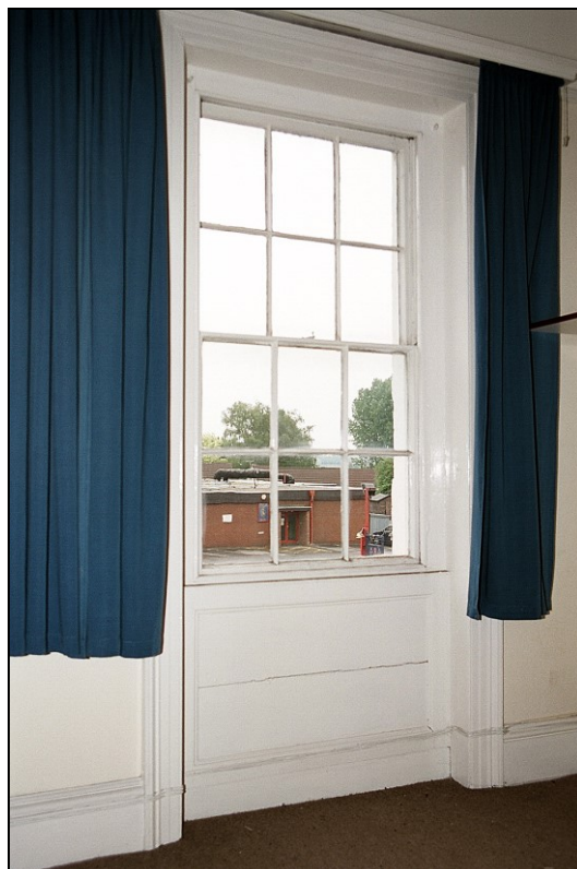
Plate 50: View SE showing 12-paned sash window within shouldered, fluted architrave
