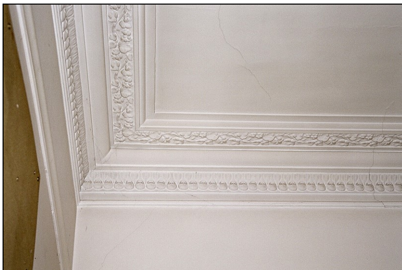
Plate 55: Detail of deep covered ceiling with enriched ovolo-moulded cornice and central panel bordered with moulded frieze with vine and leaf detailing of c.1830-40 date
