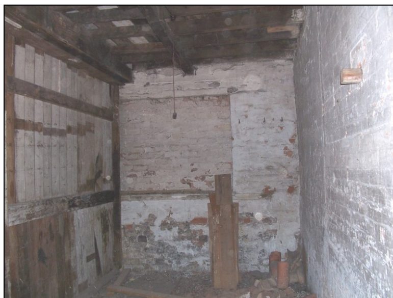
Plate 69: View S showing recess for blocked-up doorway in S wall of outbuilding range
