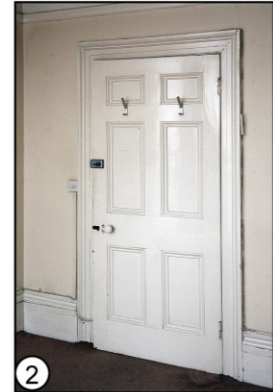
6 panelled door within fluted architrave, c. 1830 - 40
