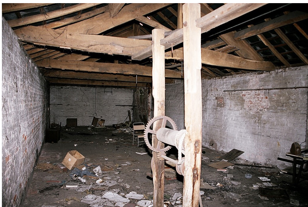
Plate 74: View W showing pulley mechanism and exposed kingpost roof trusses
