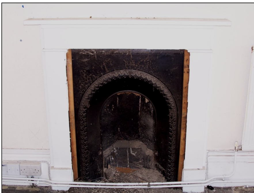
Plate 47: View N showing round-headed iron fireplace surround with repeating flowerhead motif of late Victorian date set within plain wooden surround and mantel of early-mid 19 th century date
