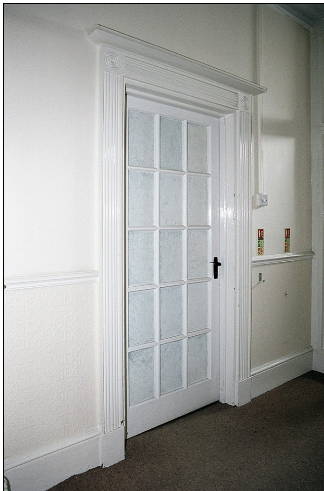
Plate 25: View NE showing modern 15-pane glazed door within a reeded, shouldered architrave with 'bullseye' paterae dated to c.1830-40
