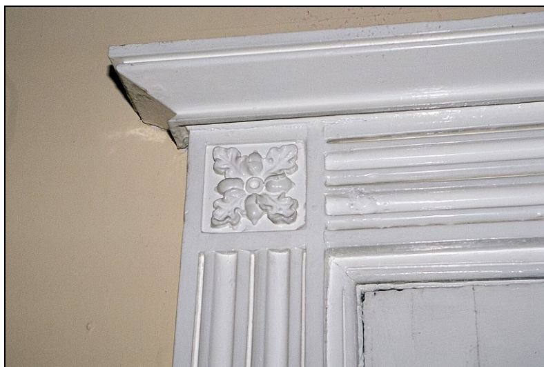
Plate 32: Detail showing quatrefoil foliage decoration in spandrel of doorcase
