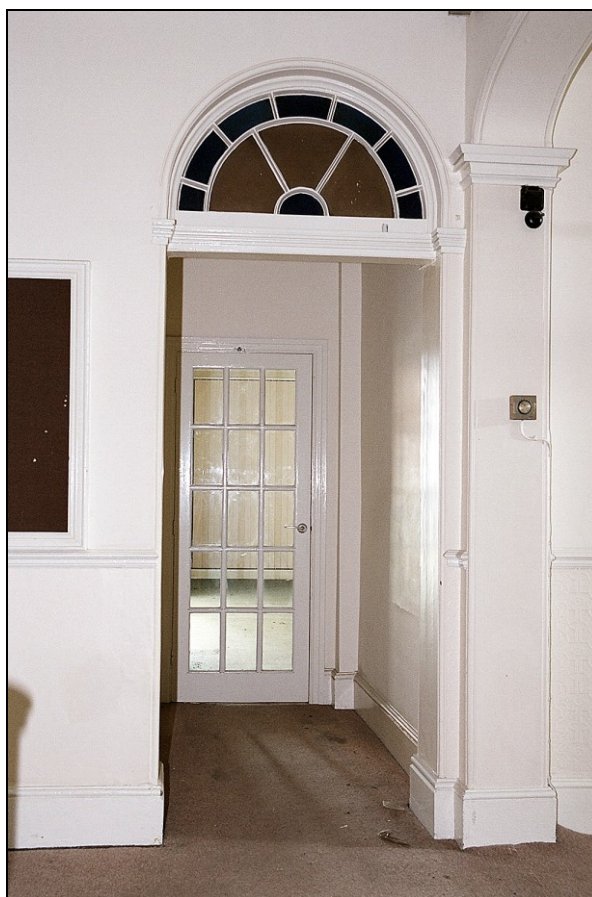
Plate 35: View N from ground-floor landing showing archway with semicircular glazed overlight
