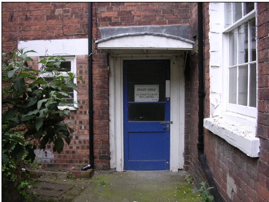
Plate 11: View N showing entrance to N wing of house with cambered porch, to left of which is evidence of a bricked-up doorway with modern window inserted
