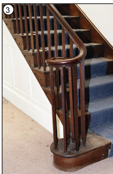
③ Open well staircase with cluster newel & stick balusters, c. 1830 - 40
