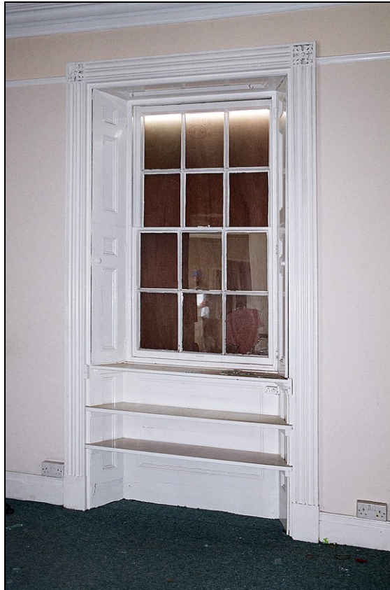
Plate 36: View SE showing 12-pane sash window within fluted architrave with quatrefoil decoration in spandrels
