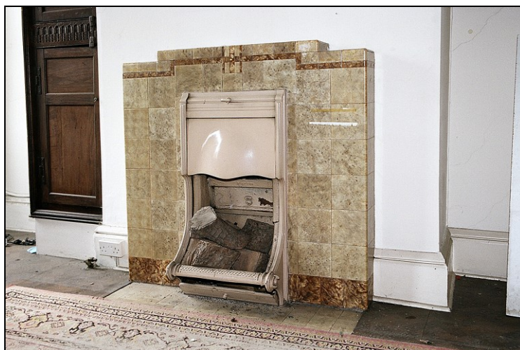
Plate 60: View looking SE showing ceramic Art Deco fireplace and tiled hearth of early 1930s date
