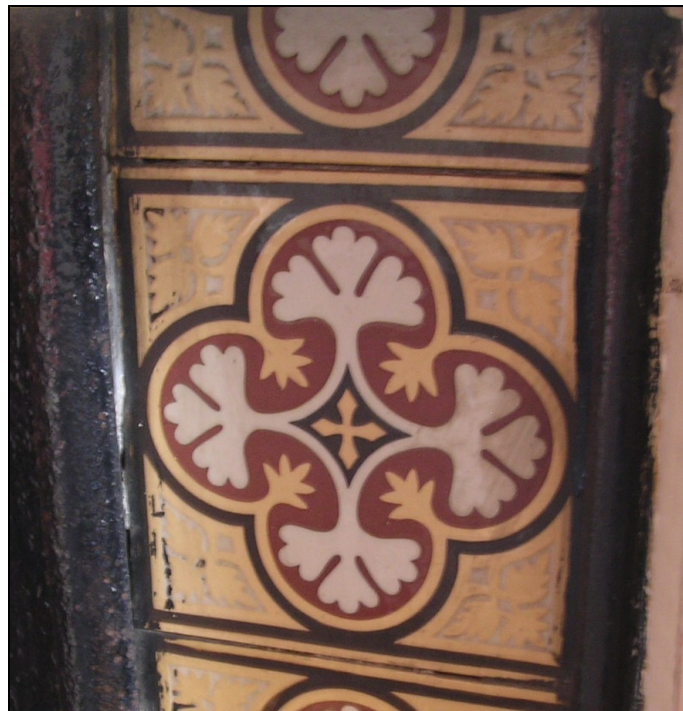
Plate 53: Detail of Neo-Gothic encaustic tile of c.1875 designed by William Godwin & Son of Lugwardine
