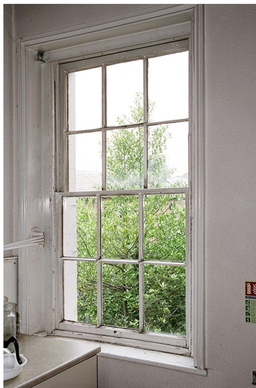
Plate 63: View W showing 12-paned sash window in single-celled room recently used as a kitchen
