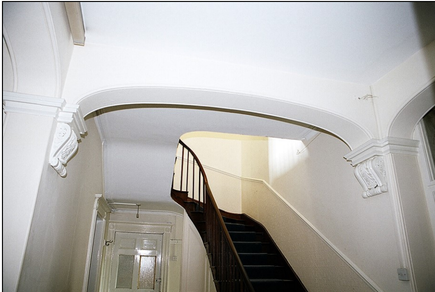
Plate 26: View showing detail of archway leading to ground-floor landing and stairwell supported by consoles with acanthus-leaf detailing
