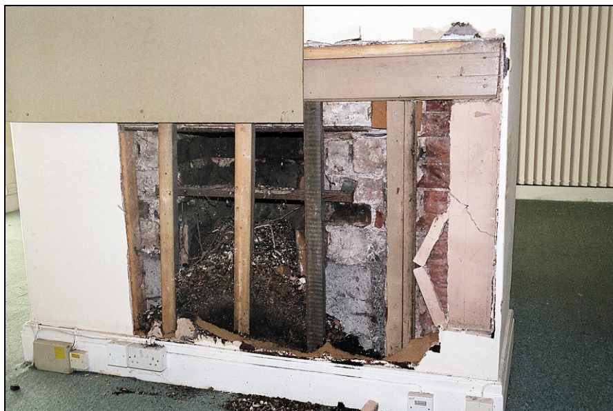
Plate 38: View N showing remains of fireplace removed after the room was converted into an open-plan arrangement in the 1960s-70s
