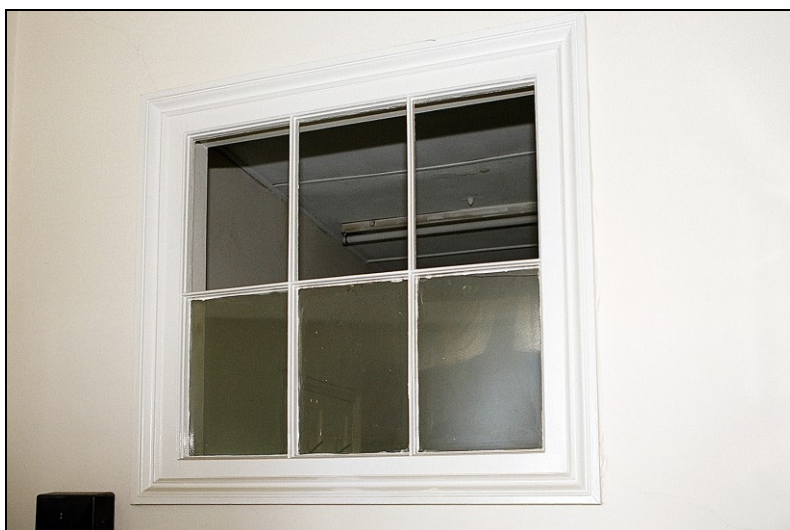
Plate 61: View looking N showing six-paned margin-glazed window in N wall
