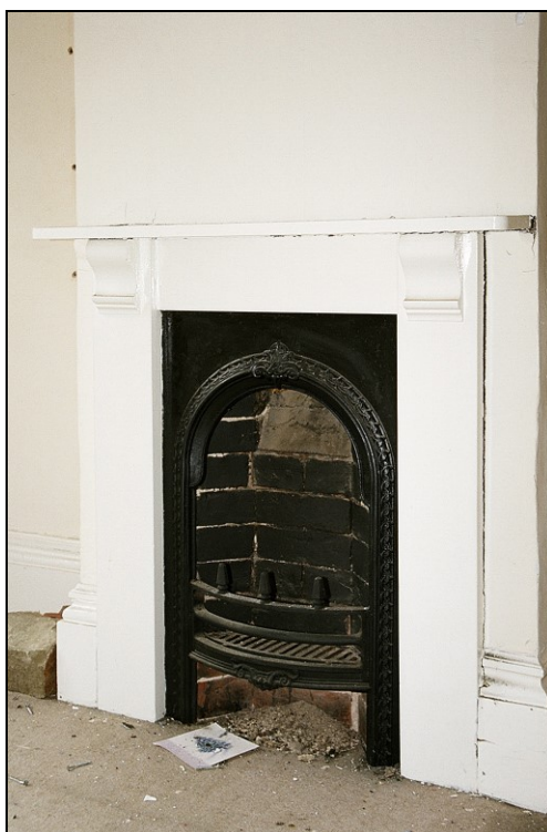
Plate 45: View showing late Victorian cast-iron basket-grate fireplace within earlier wooden surround with mantelpiece supported by plain scrolled brackets
