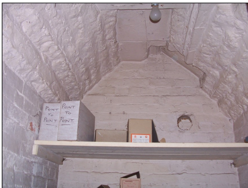
Plate 43: View showing interior of strongroom (1876) with barrel-vaulted roof
