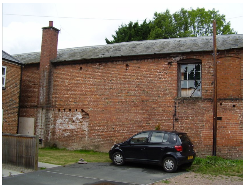
Plate 18: View N showing western part of rear elevation to outbuilding range
