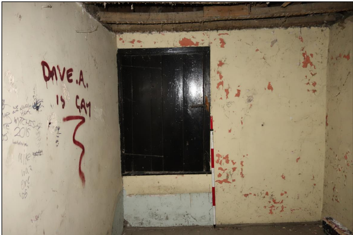
Plate 27: Internal view looking S showing hatch with plank and batten door leading to loft off first floor landing
