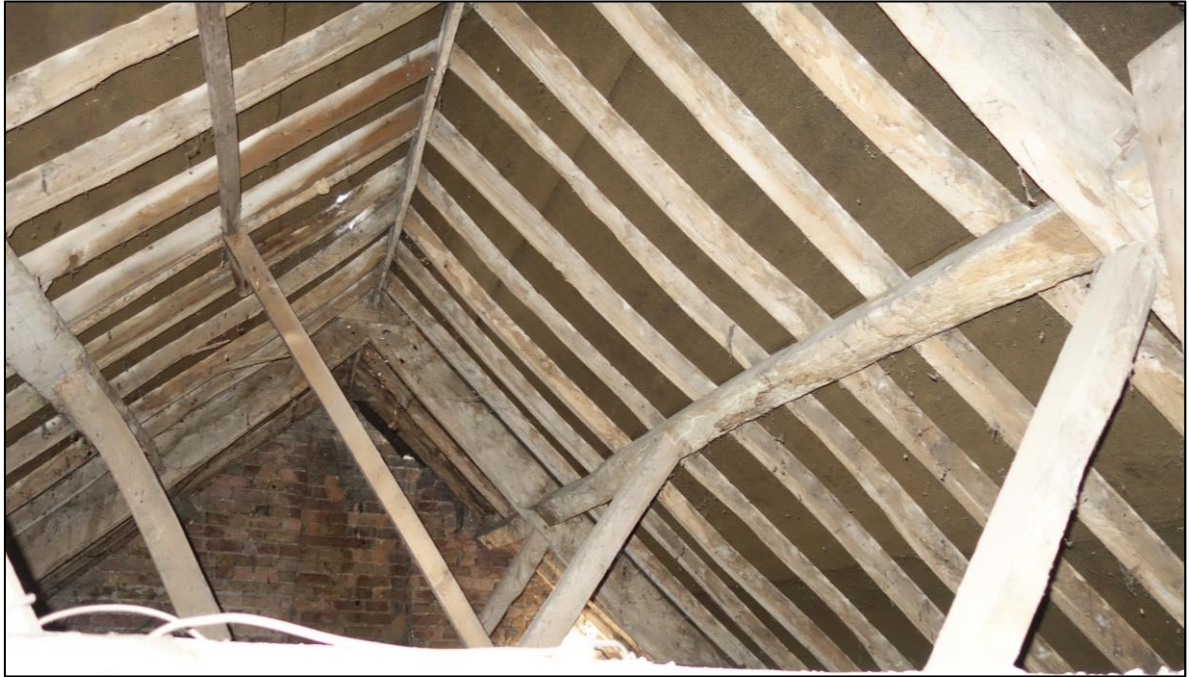
Plate 33: Internal view looking N showing detail of roof structure with angled struts connected to the principal rafters
