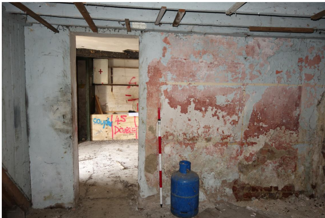
Plate 13: Internal view looking N showing doorway in N wall of central compartment with whitewashed walls and exposed ceiling joists
