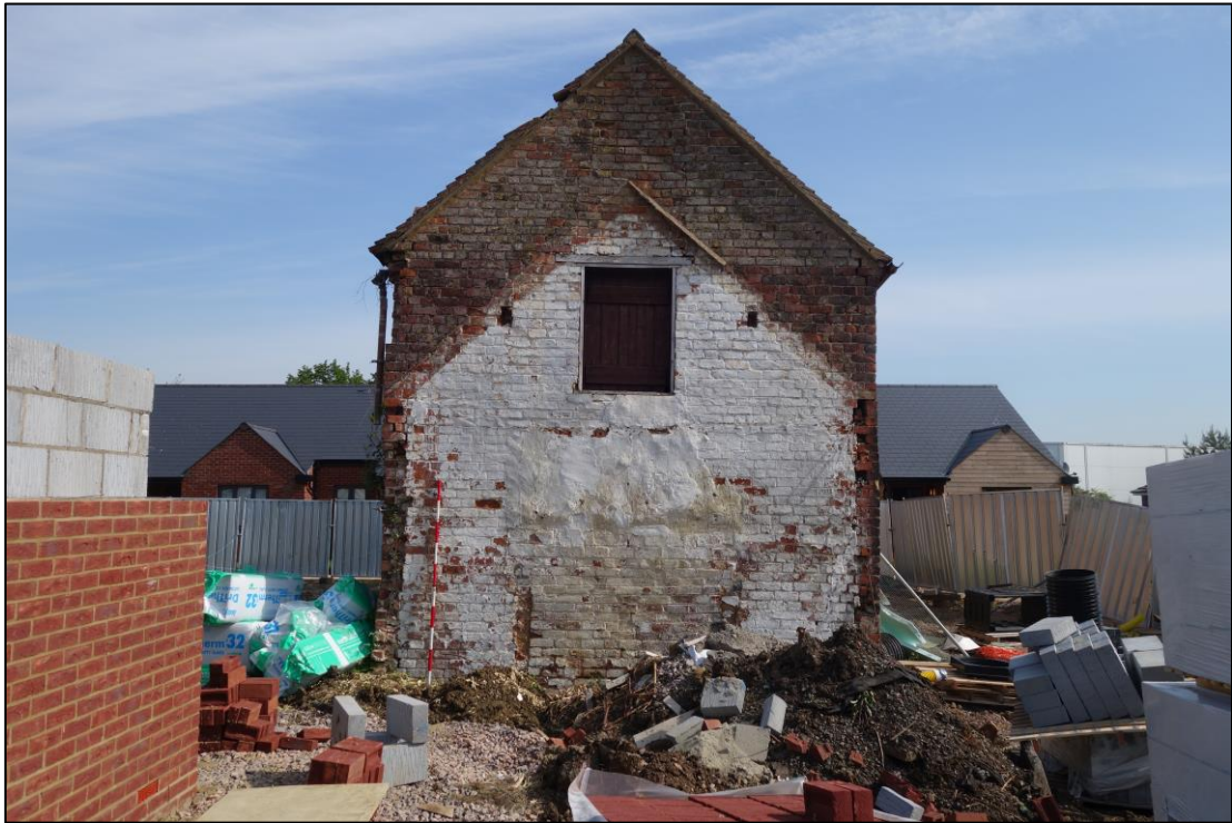
Plate 5: External view looking N showing S-gable elevation of 'Old Coach House'
