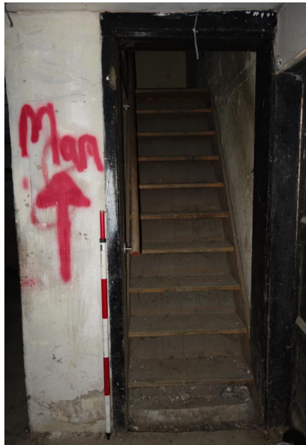
Plate 20: Internal view looking S showing staircase leading to first floor landing
