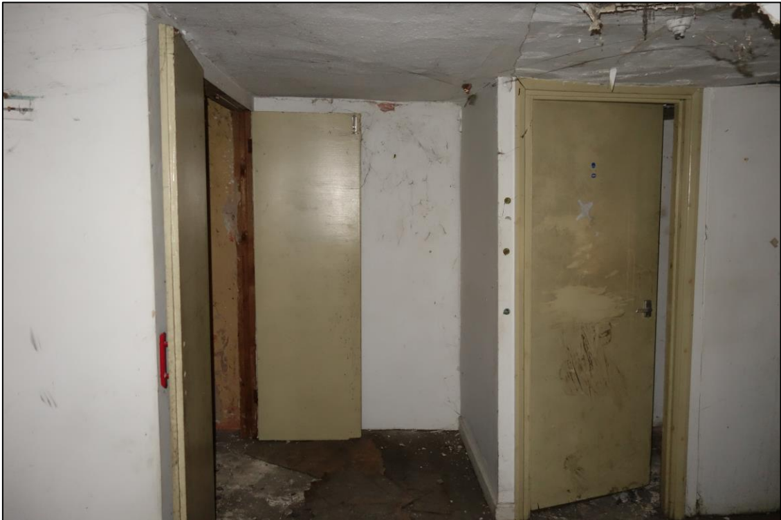
Plate 23: View looking N showing interior of northern compartment on first floor
