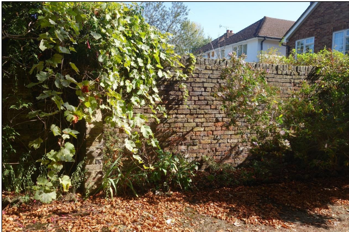
Plate 4: View looking NE showing central portion of boundary wall, laid in Flemish Stretcher Bond
