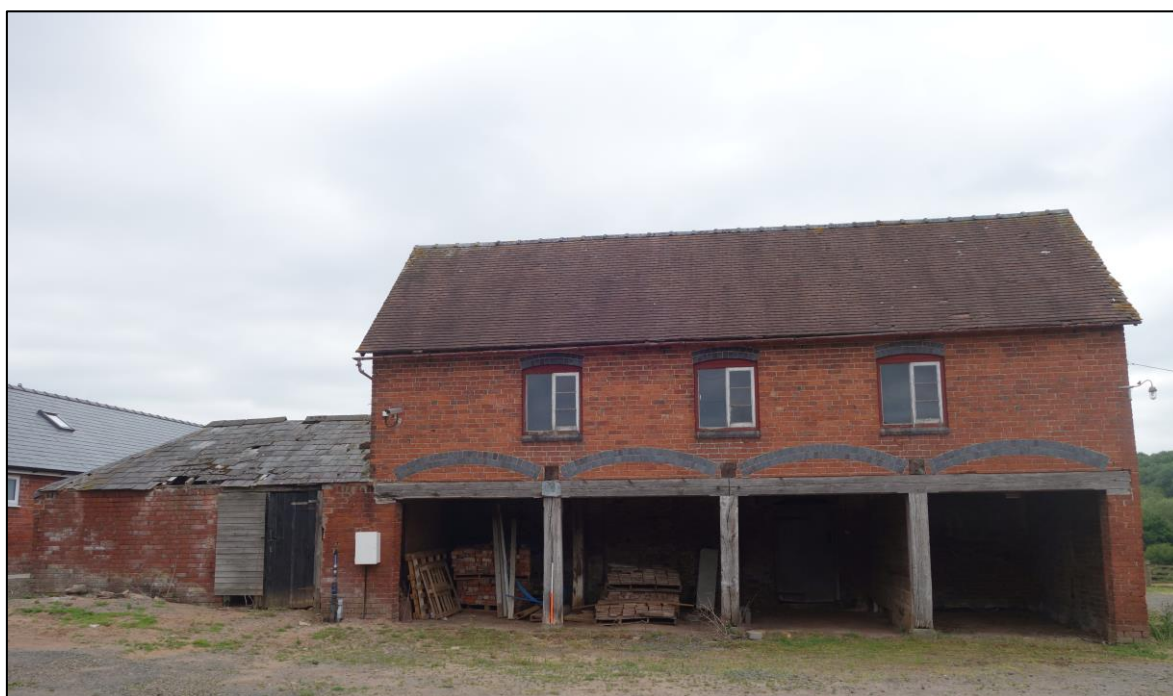
Plate 3: View looking SE showing principal NW-facing elevation of granary/cartshed with attached single storey outbuilding to the NE
