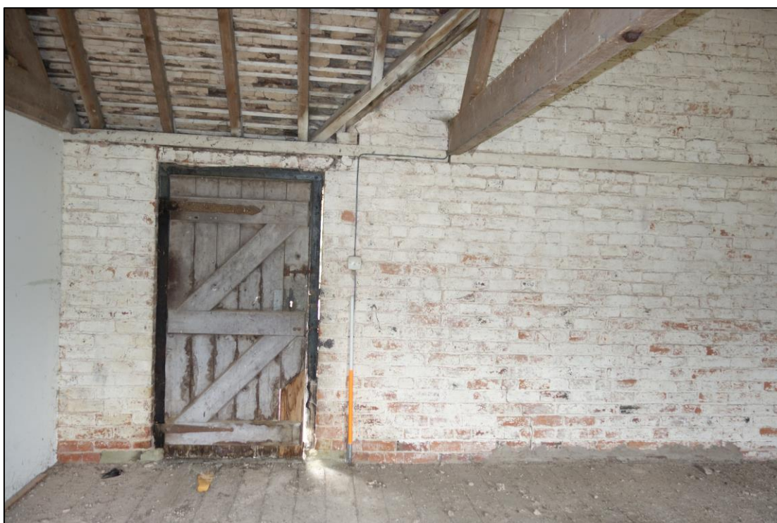
Plate 21: Internal view SE showing plank-and-batten door in SE wall of first floor granary
