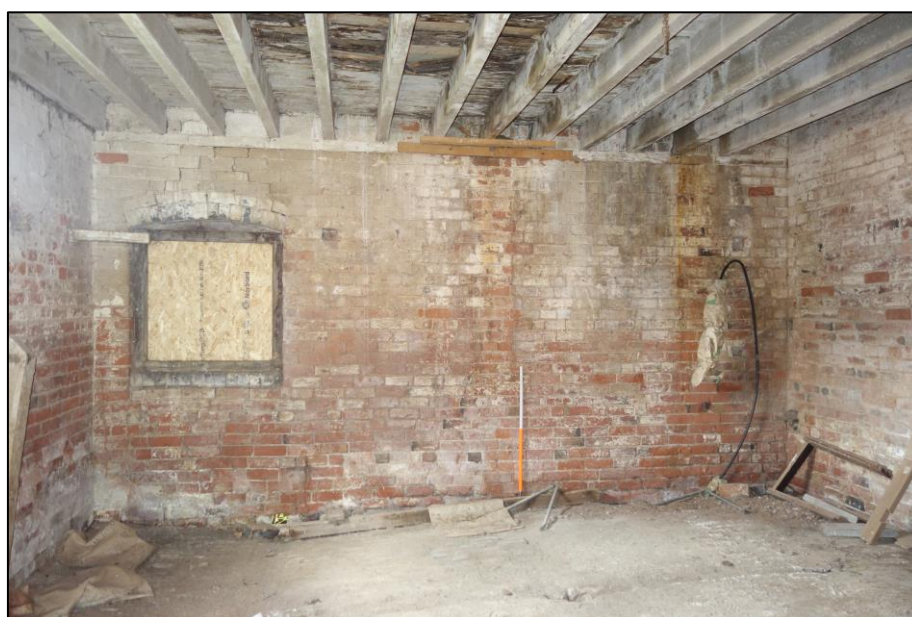
Plate 34: Internal view looking SE showing interior of granary and segmental-arched window (now boarded up)
