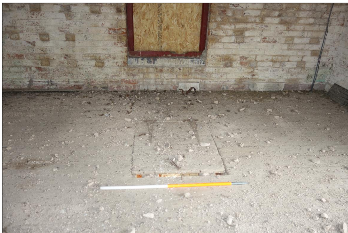
Plate 26: Internal view looking SW showing detail of floorboards and trap door in SW bay of granary
