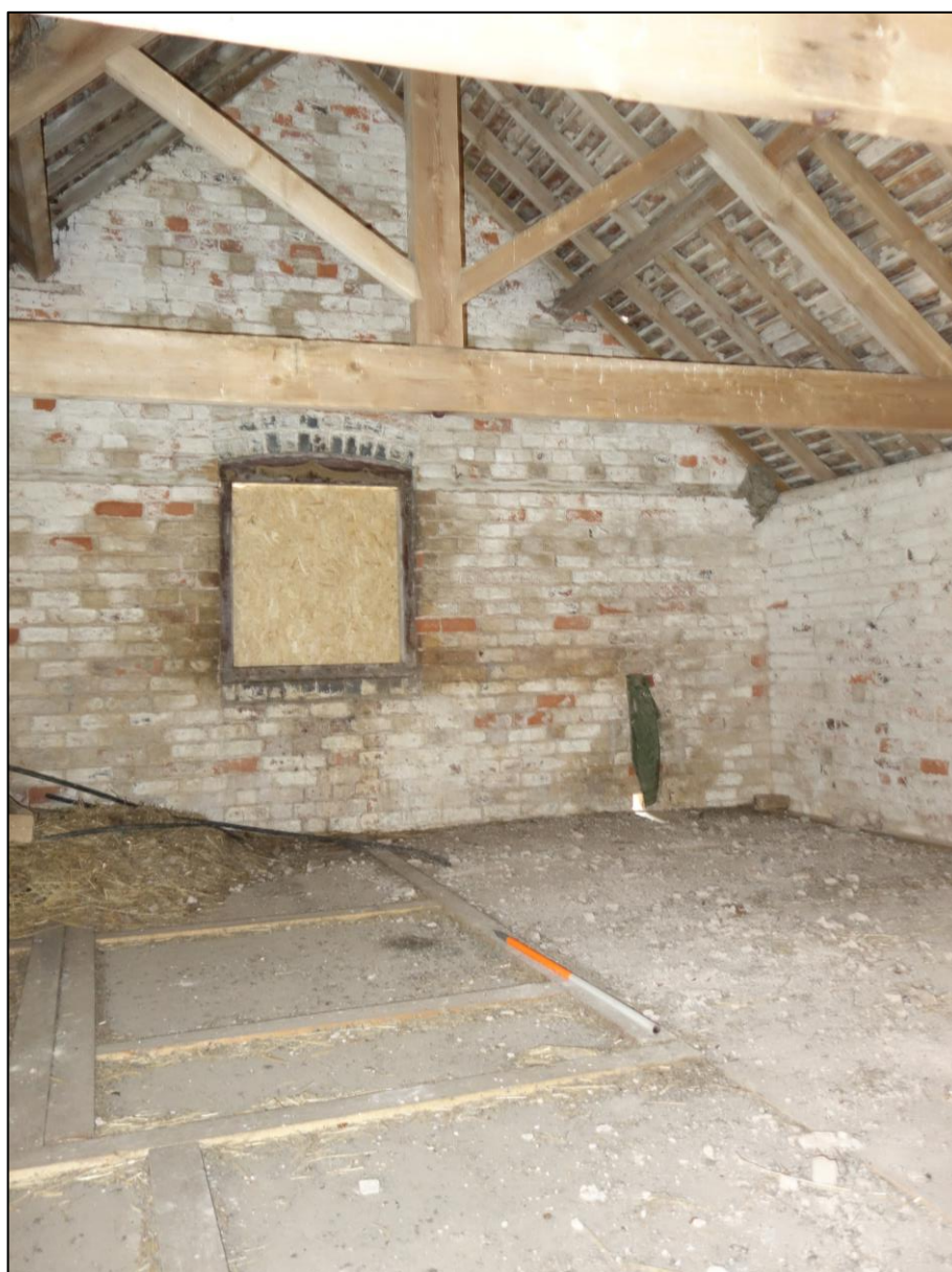
Plate 37: View looking SE showing southeasternmost bay of hayloft with segmental-arched window in SE wall and partially denuded flooring in loft
