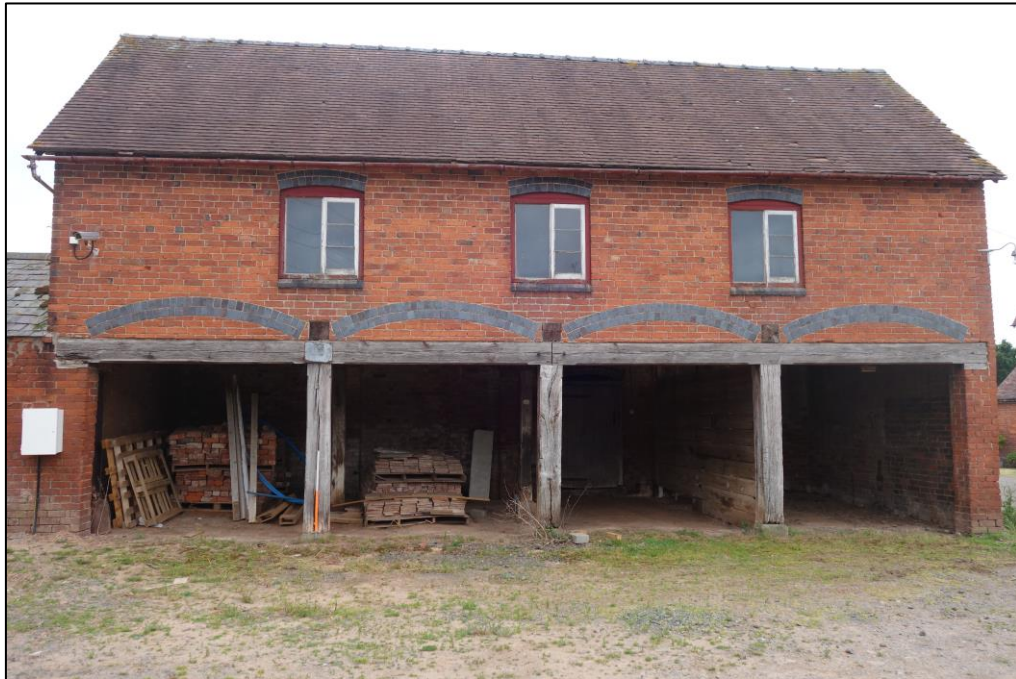
Plate 4: View looking SE showing open-fronted cartshed and first floor granary with segmental-arched casement windows
