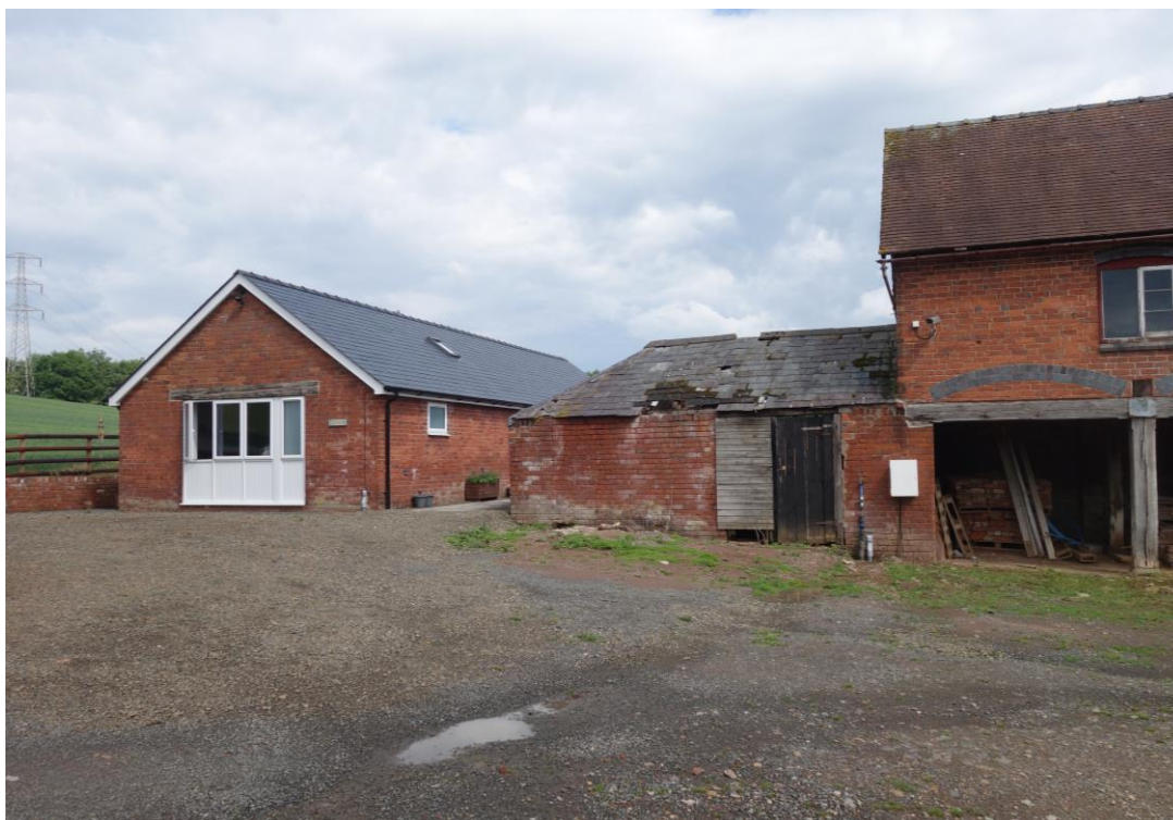
Plate B: View showing late 20 th century outbuilding (now converted into a bungalow) to NE of the traditional farm building
