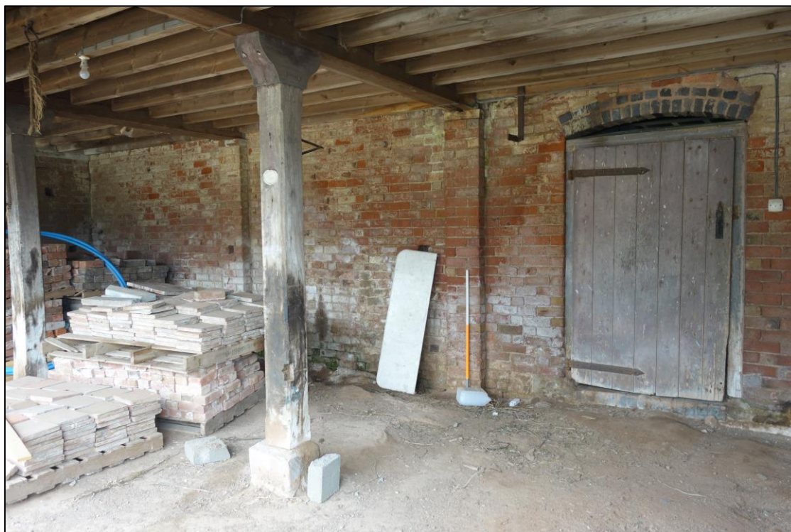
Plate 15: View E showing interior of central bays of cartshed with segmental-arched doorway in wall leading to stable range (to right of picture)
