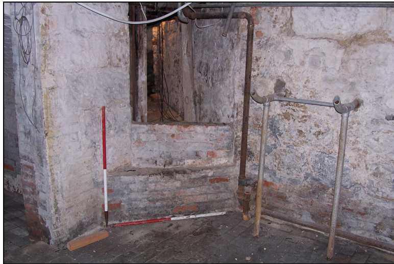
Plate 6: View SW showing entrance from cellarage into passage
