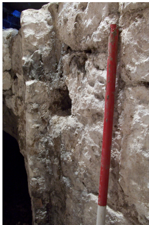
Plate 9: Detail showing slots within masonry wall of passage adjacent to chamber entrance, looking SW
