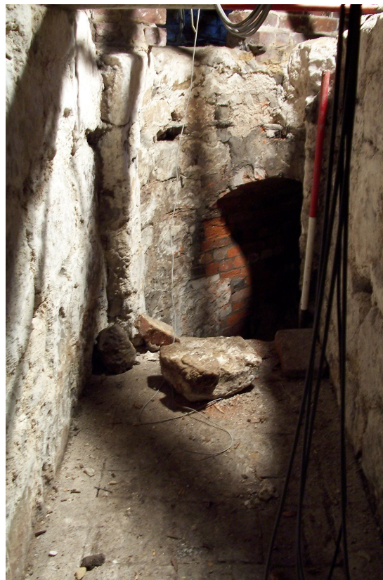
Plate 7: View looking SW along passage from cellarage entrance
