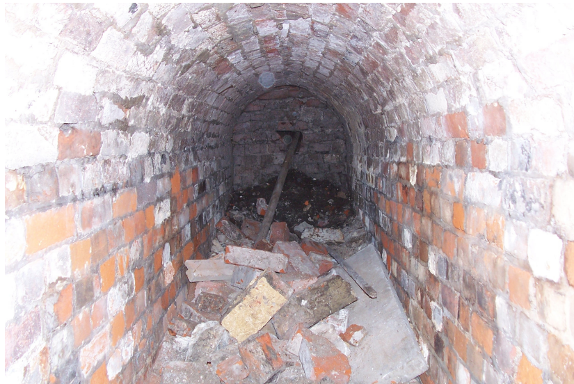
Plate 8: View looking NW showing brick tunnel from chamber to western side of No. 19.
