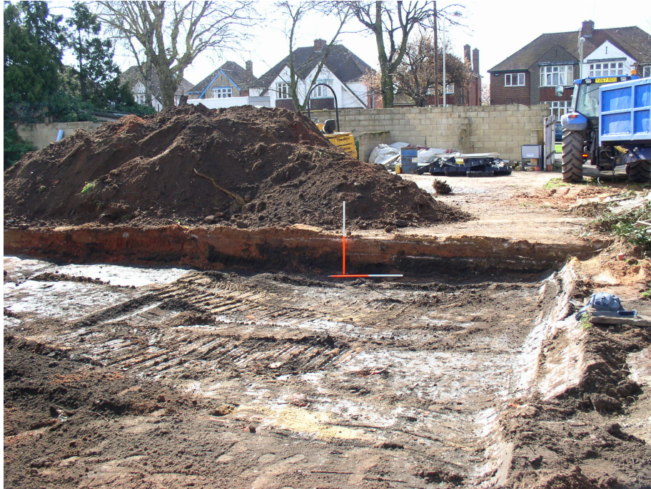
Plate 2: Excavated area, phase 1, looking S
