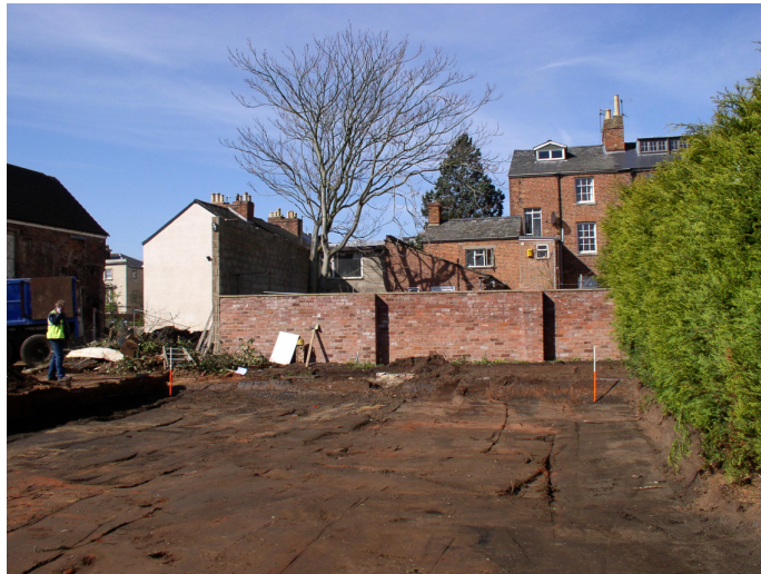
Plate 1: Excavated area (Phase 1), looking W
