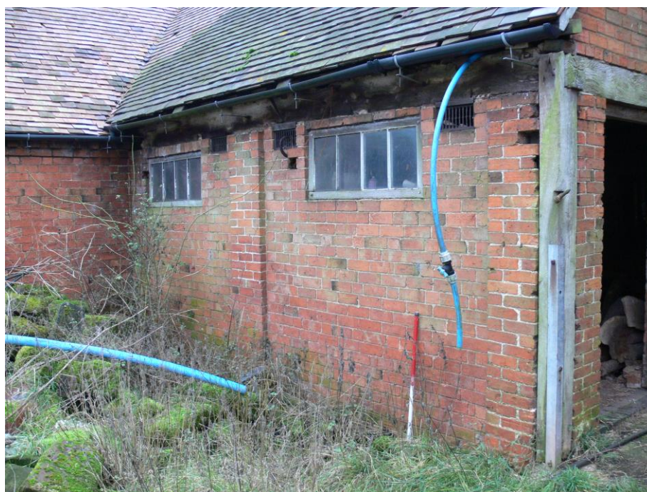
Plate 9 View looking SE showing N-facing elevation of southern range of Barn 3 showing original eaves cornice replaced by timber wall-plate
