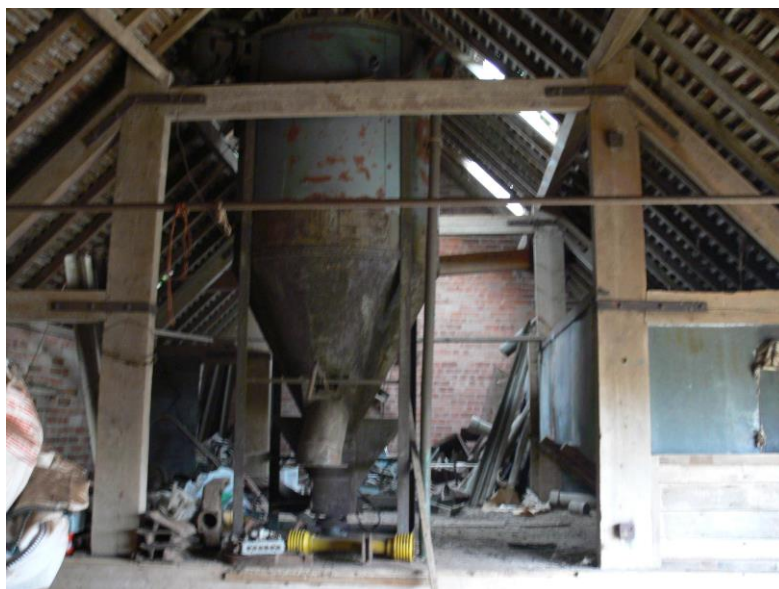
Plate 33: View looking W showing roof construction of Barn 2 with queen-post trusses
