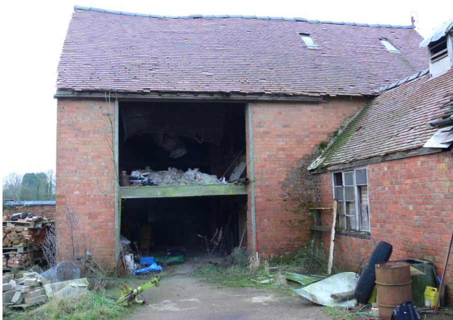
Plate 28: View looking S showing N-facing elevation of Barn 2 with wagon entrance
