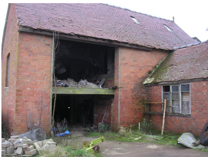
Plate 35: View looking SW showing construction break between Barn 2 and extension to N
