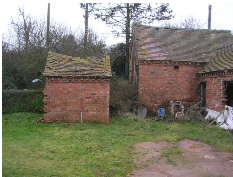
Plate 25: View W showing swill house and freestanding building ('boar pen') situated immediately to the S
