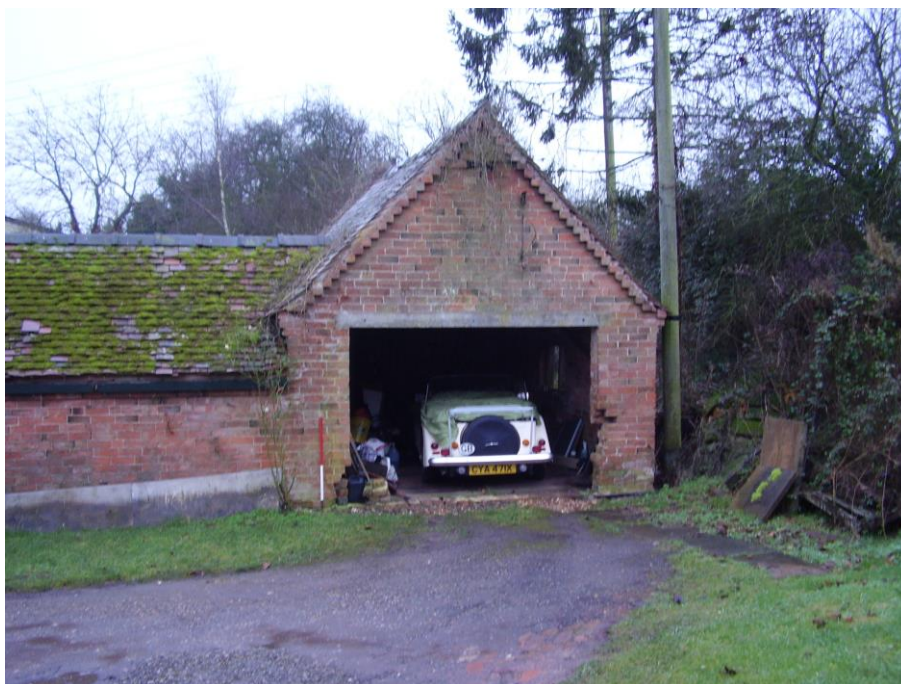
Plate 26: View looking S showing N-facing gable elevation of Barn 6 with modern carport inserted
