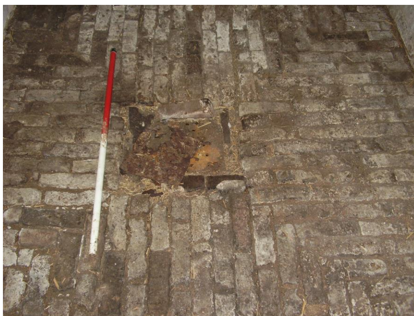
Plate 16: Plan view showing cobbled flooring and drain in L-shaped compartment of Barn 4
