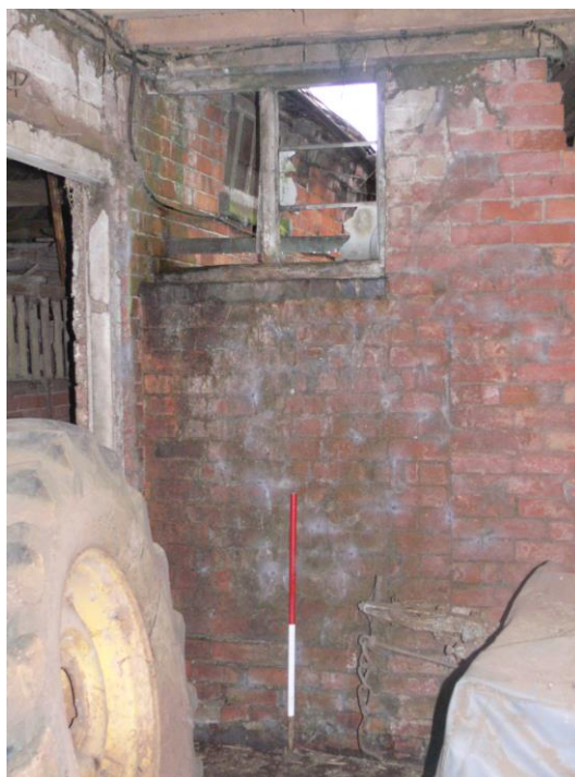
Plate 31: View N showing bricked-up doorway in NW corner of Barn 2
