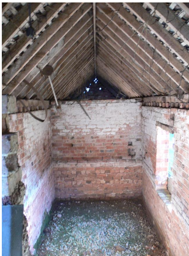
Plate 24: Internal view W showing gable wall of pigsty range with evidence of raised floor level
