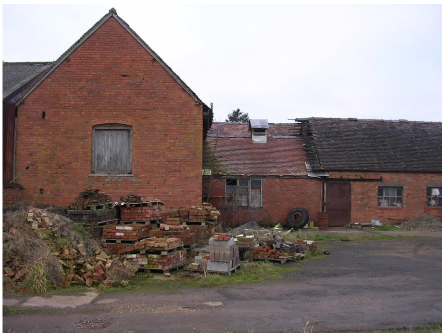
Plate 29: View looking W showing E-facing gable elevation of Barn 2 and extension to N
