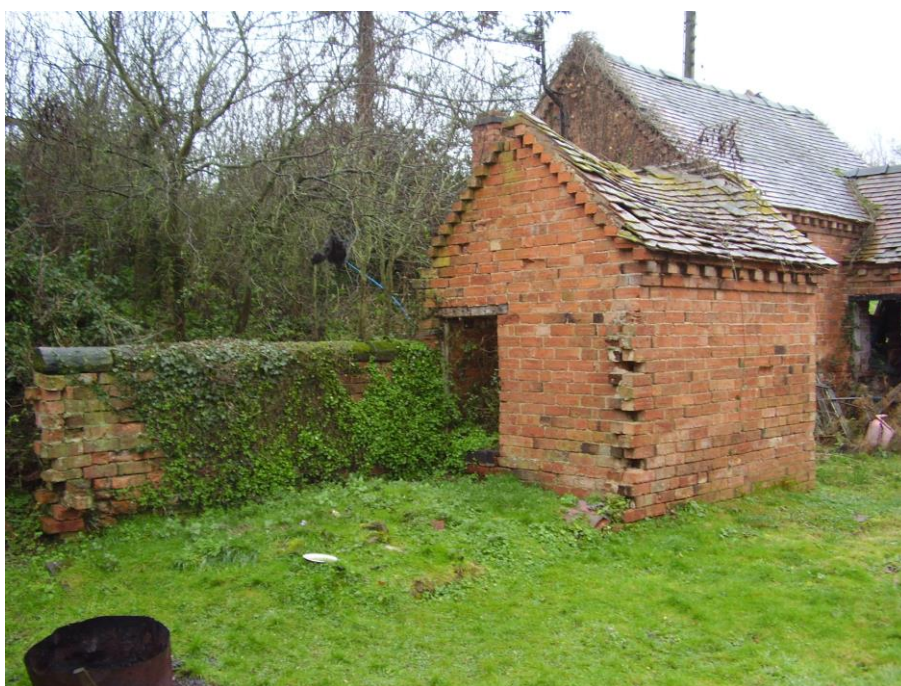
Plate 27: View looking NW showing 'boar pen' and remains of adjoining enclosure wall with 'swill house' to rear
