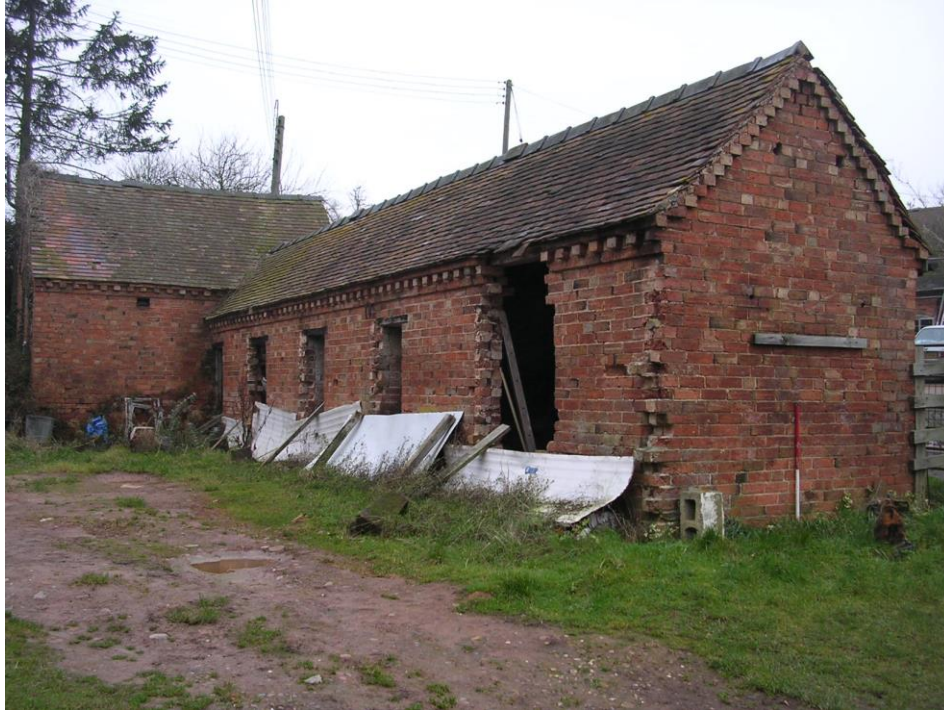
Plate 23: View NW showing gabled pigsty range with projecting wing at the W end built to accommodate a swill house
