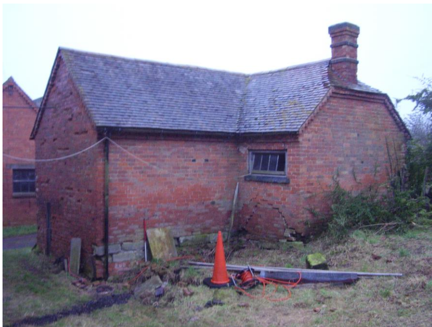
Plate 15: View SW showing rear N-facing elevation of Barn 4 with gabled N wing with half-hipped roof surmounted by chimneystack
