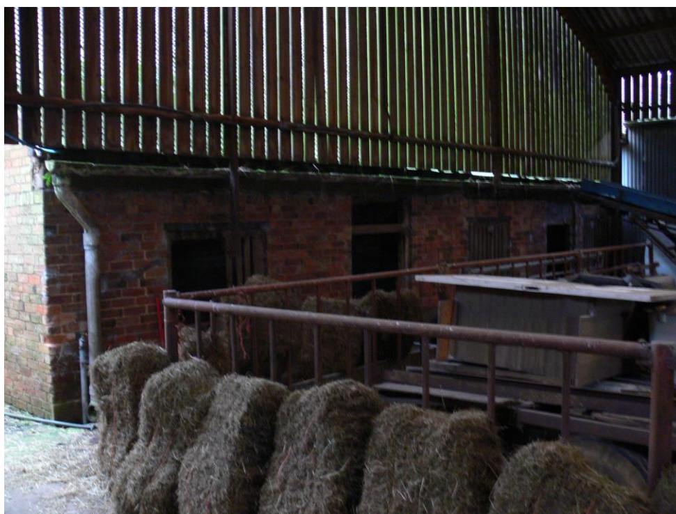
Plate 11: View looking NE showing S-facing elevation of Barn 3
