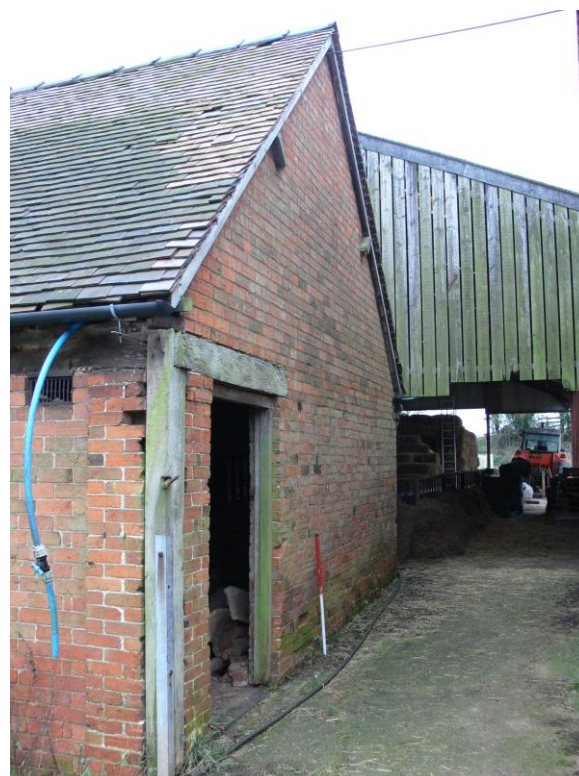
Plate 10: View looking S showing W facing gable of Barn 3
