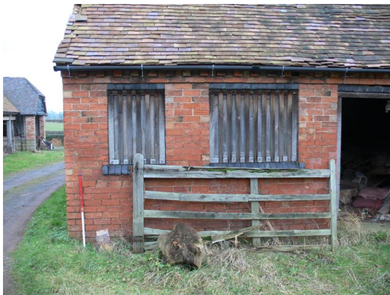
Plate 5: View E showing detail of N end of W-facing principal elevation of Barn 3, showing dentilled eaves
