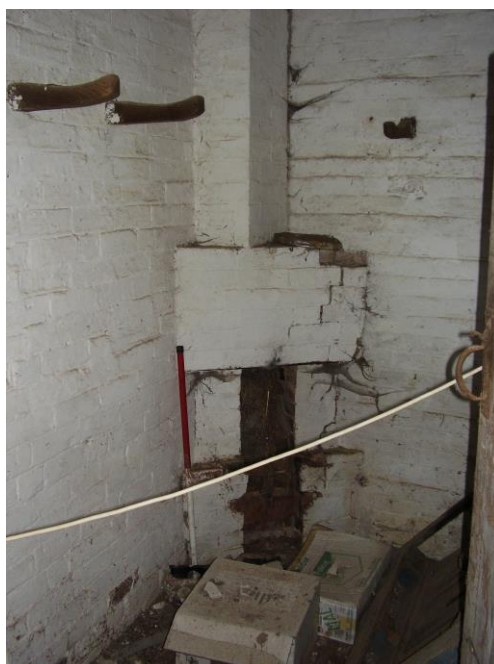
Plate 18: View looking N showing harness room in Barn 4 with fireplace in NW corner
