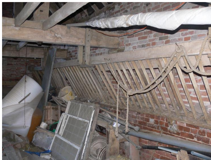
Plate 21: Internal view SE, showing racks mounted along N-facing wall of barn
