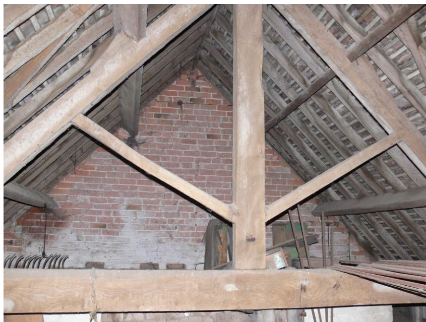
Plate 7: View S showing kingpost roof truss in Barn 3
