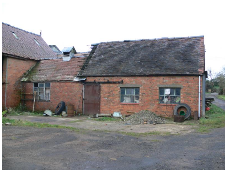
Plate 37: View looking W showing E-facing elevation of brick extension to Barn 2
