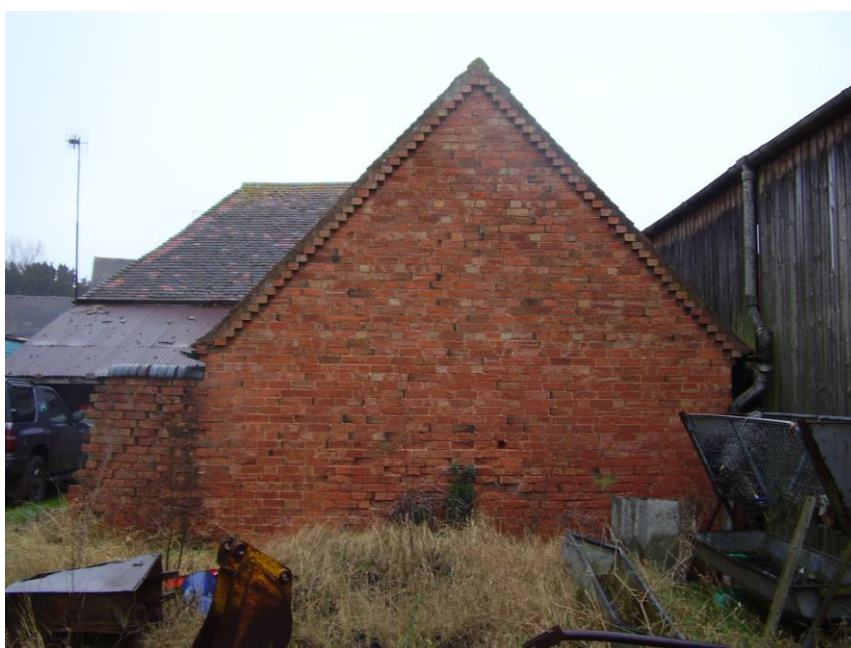
Plate 20: View N showing S gable end of extension to Barn 5
