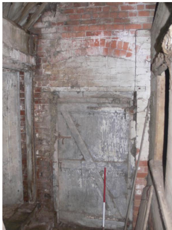
Plate 13: View E showing bricked-up segmental arched doorway at E gable end of Barn 3 with later flat-headed doorway inserted
