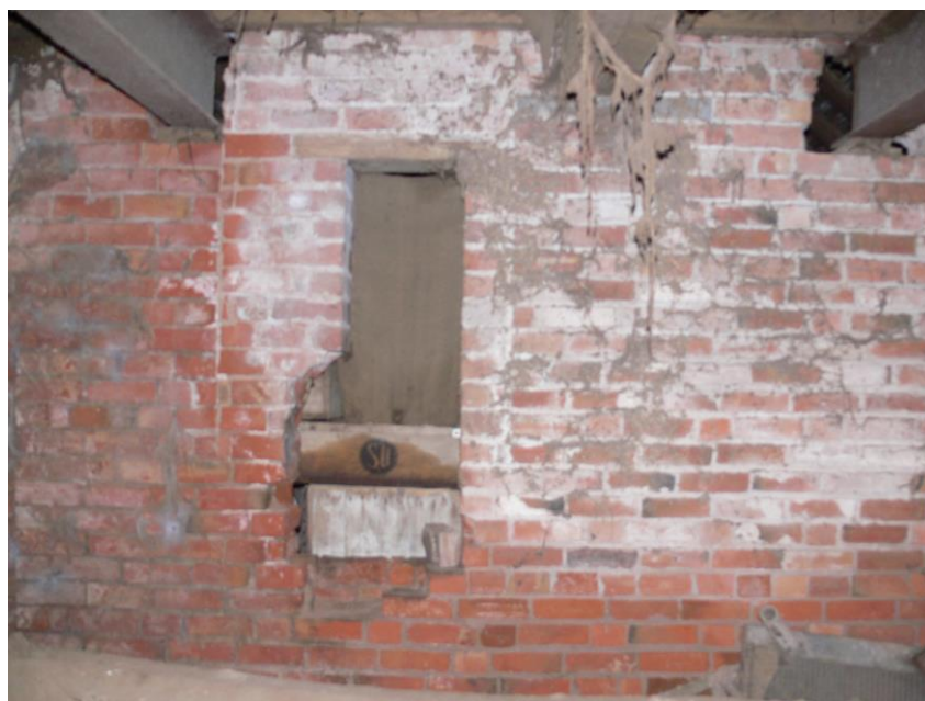
Plate 32: View N showing bricked-up window in S-facing wall of Barn 2
