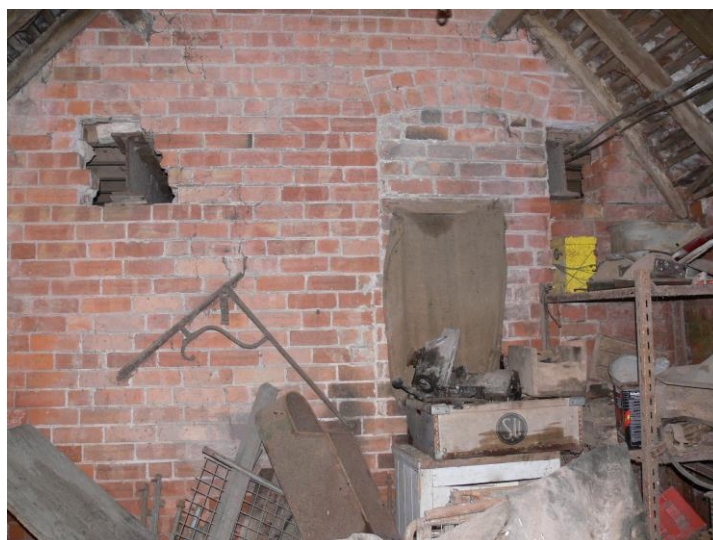
Plate 36: View looking W showing bricked-up window at S end of extension to Barn 2
