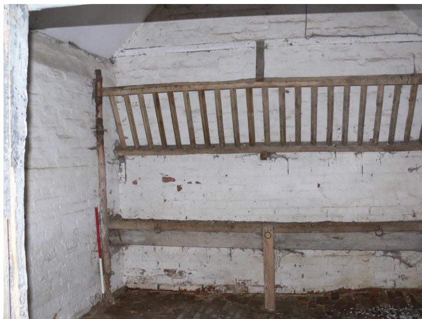
Plate 17: Internal view N showing wooden hayrack and trough attached to N wall
