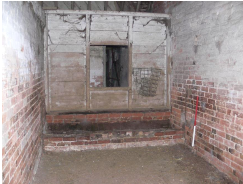
Plate 12: View N showing brick-lined trough and wooden partition wall on N side of southern range of Barn 3
