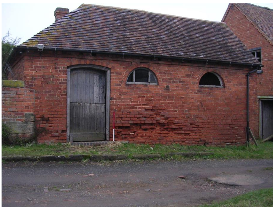
Plate 14: View N showing S-facing elevation of Barn 4
