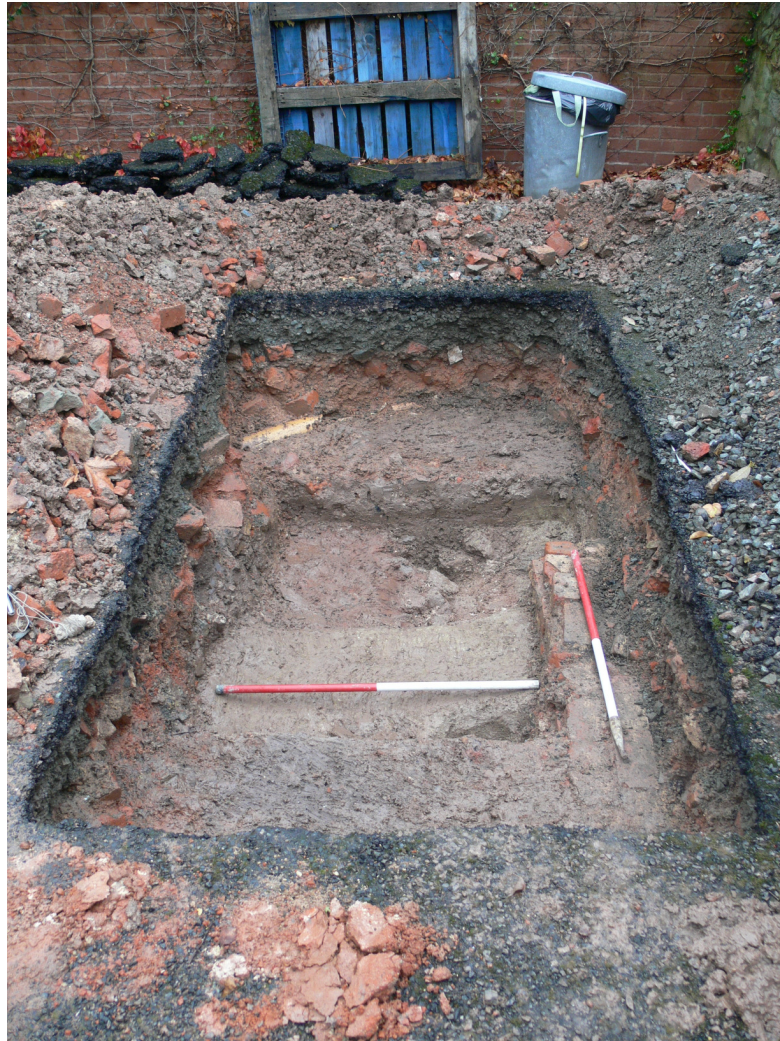
Plate 1: Trench overview, looking NE
