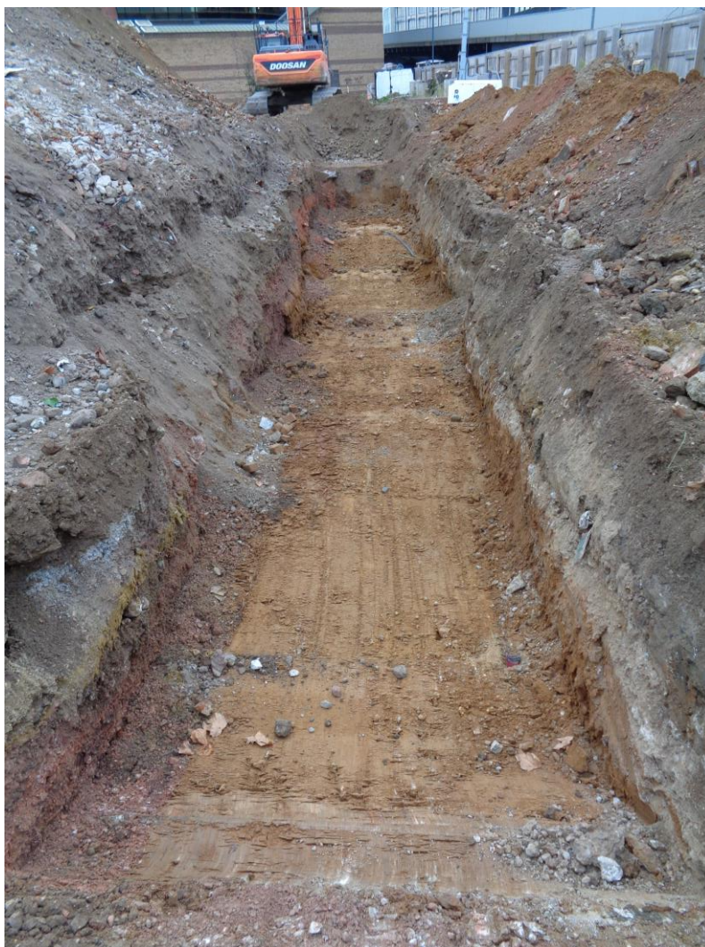
Plate 2: View WNW of Trench 002
