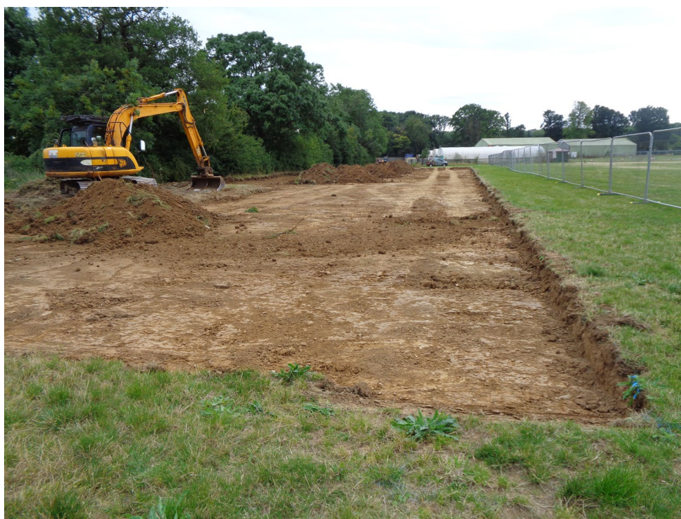
Plate 2: SW-facing, showing Trench 001
