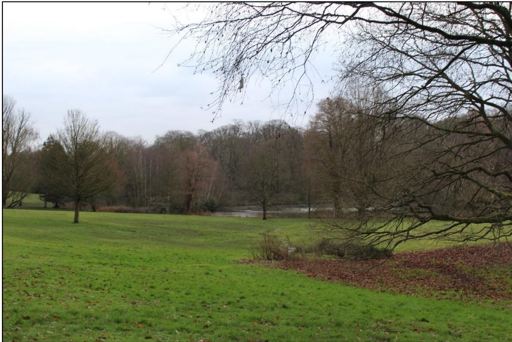
Viewpoint 4: View looking SW towards Wood Pond with inspection chamber for drainage run visible in foreground
