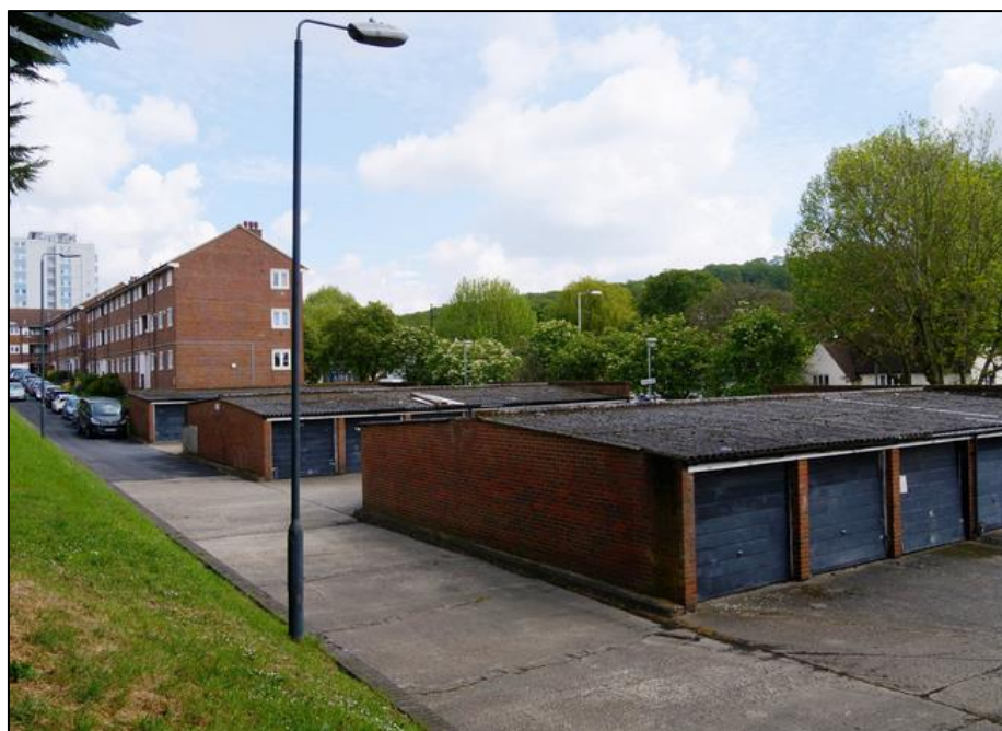
Plate 1: View looking E across site occupied by lockup garages, with modern council flats in background
