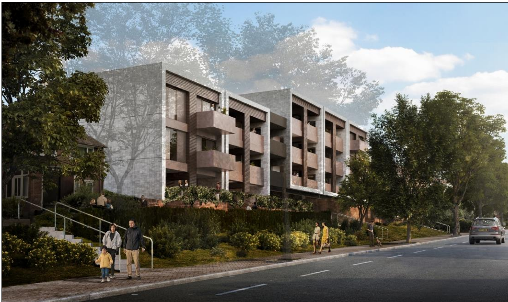
Fig. 6: CGI Visual showing E frontage of proposed new residential development fronting onto Well Hall Road (Reproduced by courtesy of Shedkm Architects)
