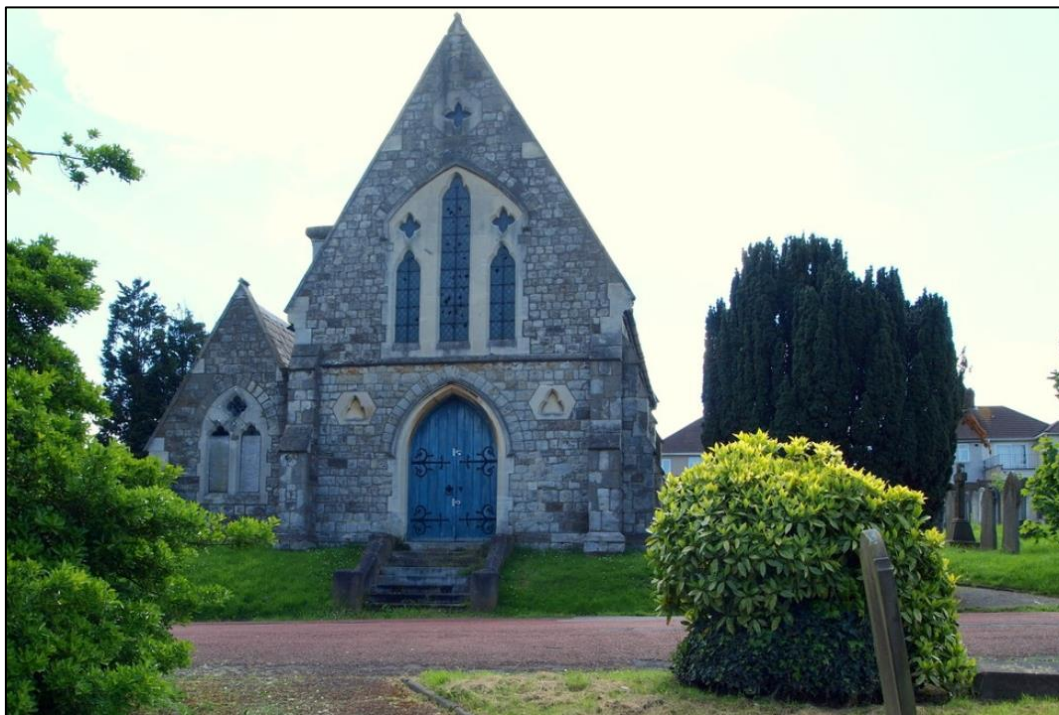
Plate 10: View SW towards nonconformist chapel and beyond towards the SW boundary of the cemetery bordered by 1930s houses along Dunblane Road
