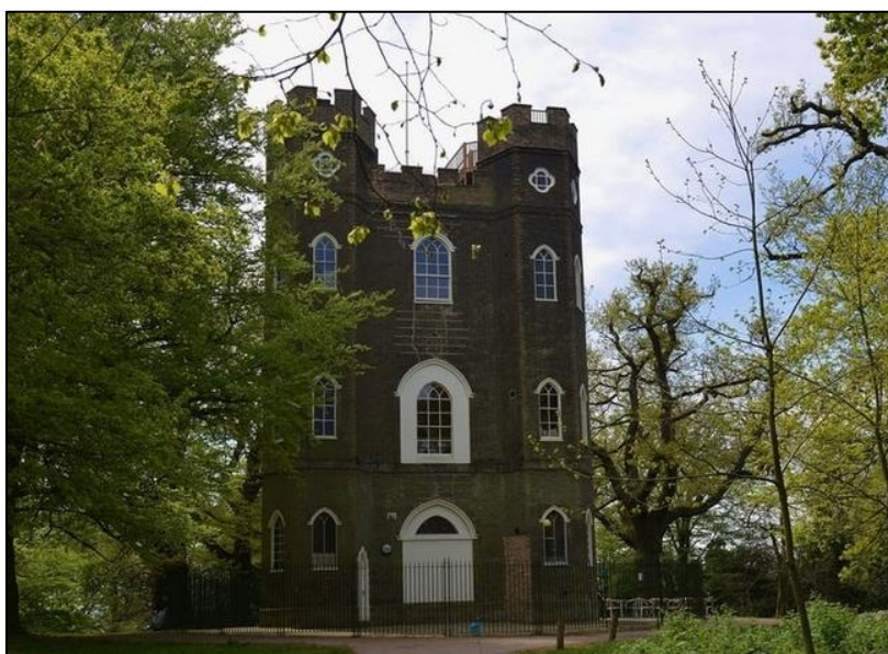
Plate 7: View looking S towards the N front of Severndroog Castle, a Grade II* Listed building erected in 1784
