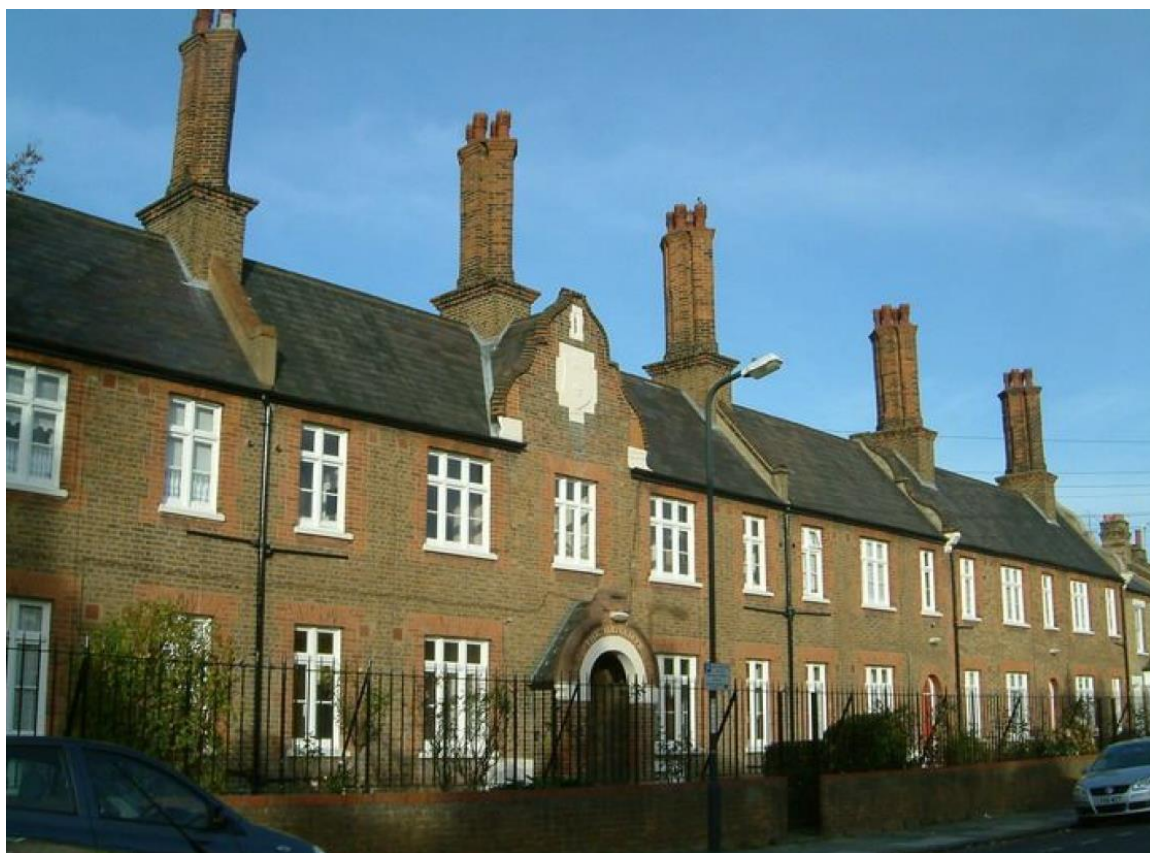
Plate 4: View NE towards Hatcliffe Almshouses on Tuskar Street, originally built in 1857
