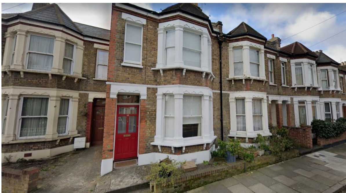
Plate 5: View S towards row of two-storey early 20 th century terraced houses along the S side of Tuskar Street
