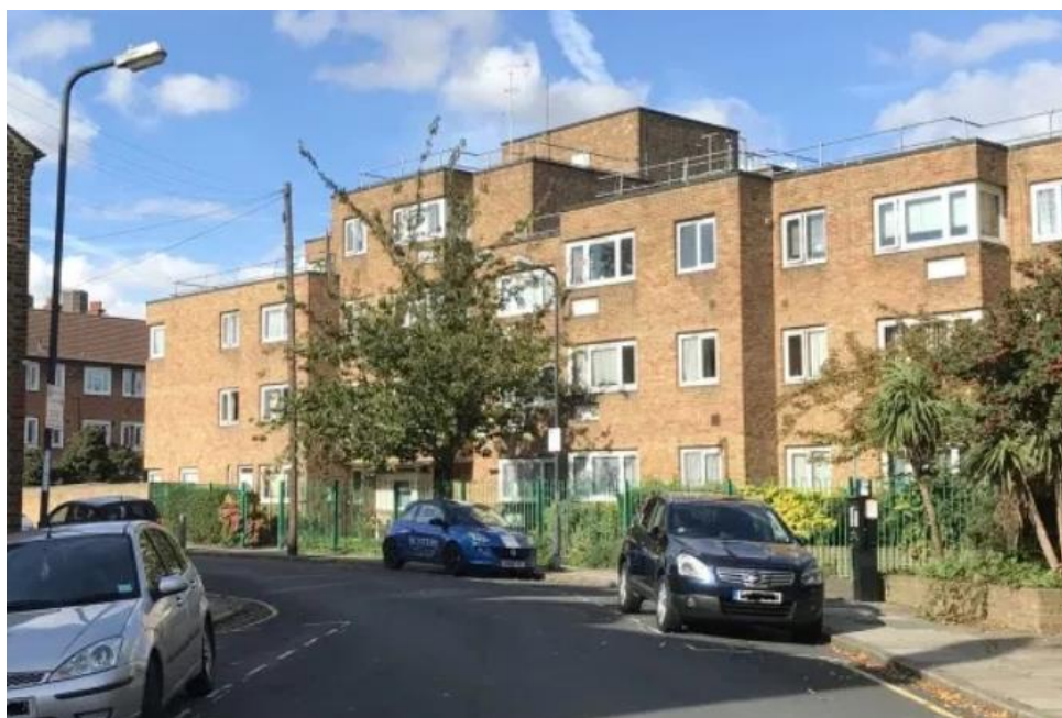
Plate 1: View looking NW along Tuskar Street showing the late 1970s sheltered housing prior to demolition
