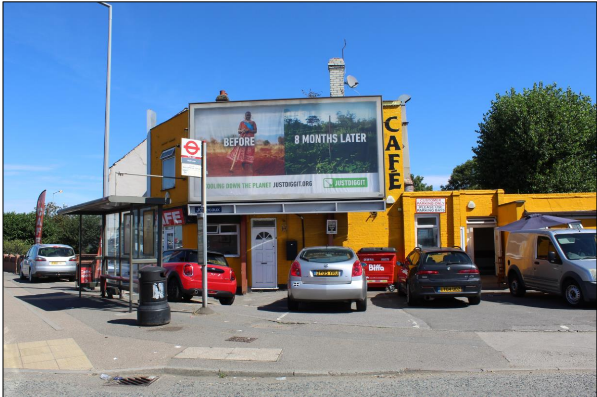
Plate 1: View looking N from Westward Road towards the existing premises at No.335 Hall Lane
