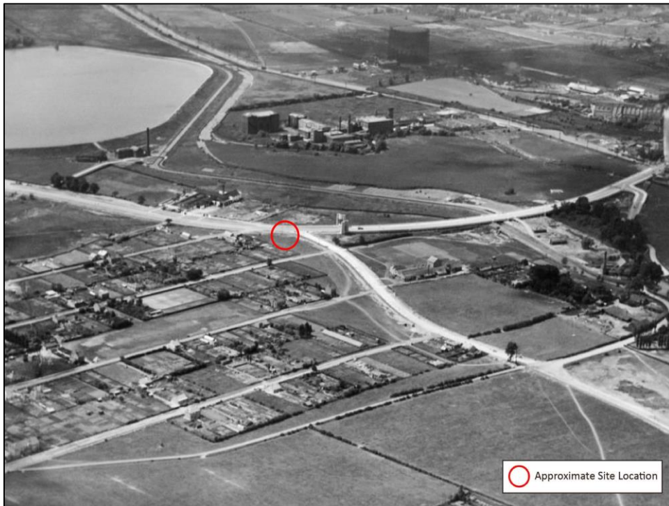
Fig. 15: Extract from an oblique aerial photograph of Chingford taken in June 1927, looking SW and showing the site located at the W end of Westward Road, immediately E of the newly-constructed North Circular Road (Reproduced by courtesy of the Historic England Archive)
