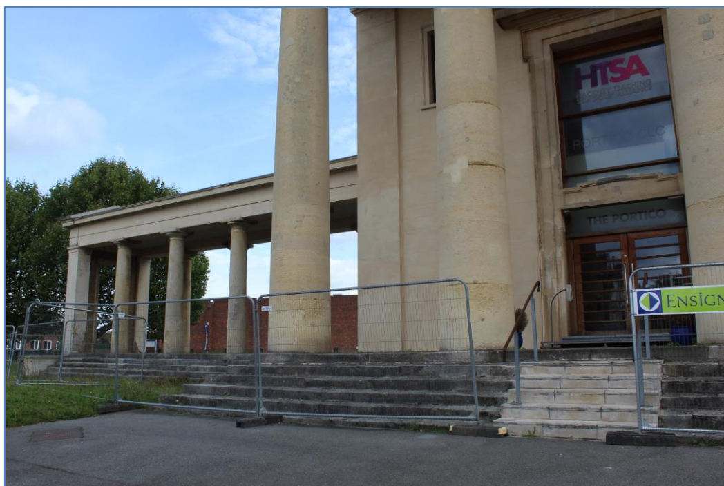
Plate 2: View NE showing colonnade to N of portico
