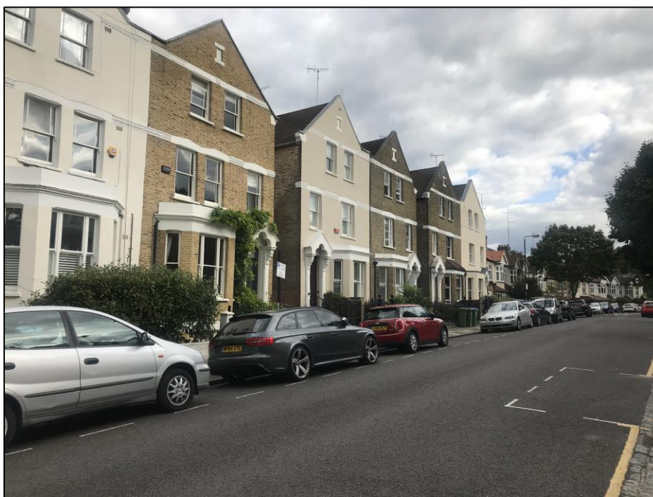
Plate 4: Oblique view SE looking towards No. 29 and neighbouring semi-detached villas built in the early 1880s along the E side of Mycenae Road
