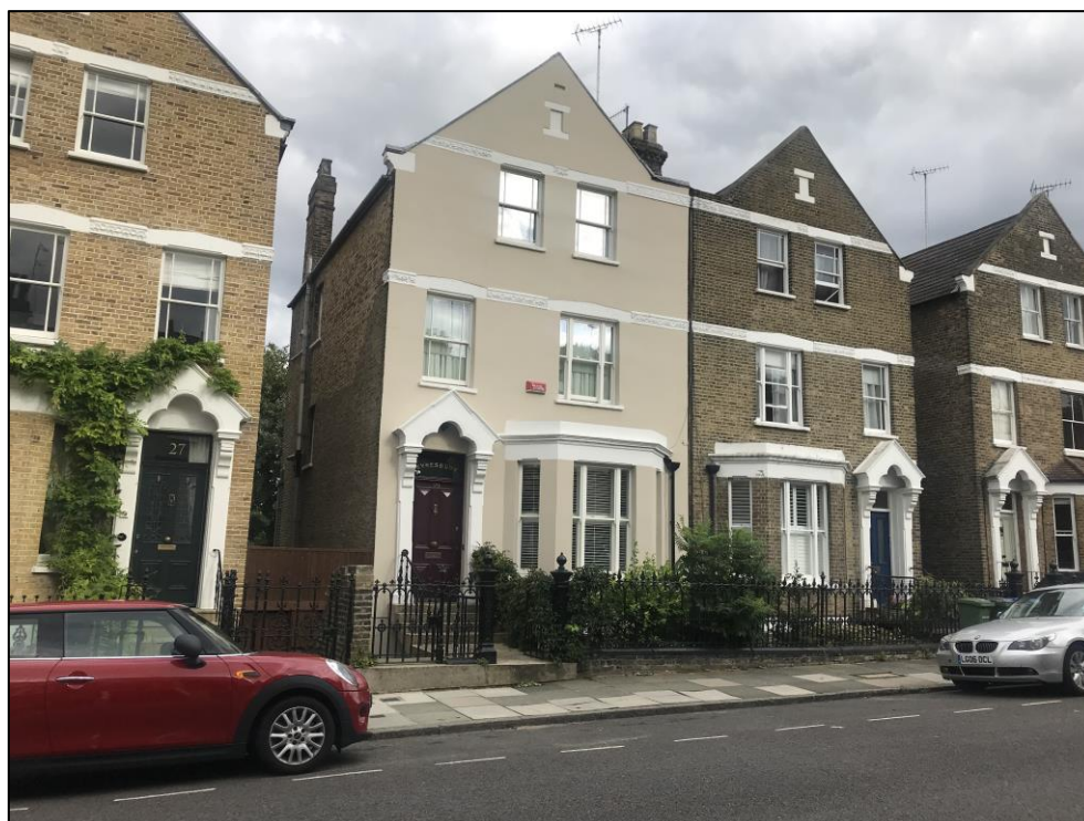
Plate 3: Oblique view looking ESE showing No. 29 Mycenae Road and adjoining semi-detached houses of late 19 th century date
