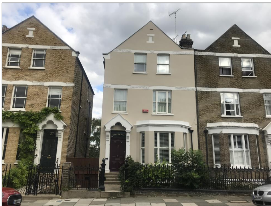
Plate 1: View looking E showing exterior of No. 29 Mycenae Road
