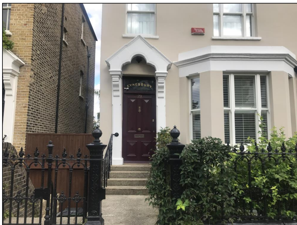
Plate 2: View showing gabled entrance porch to No. 29 Mycenae Road with projecting bay window to right
