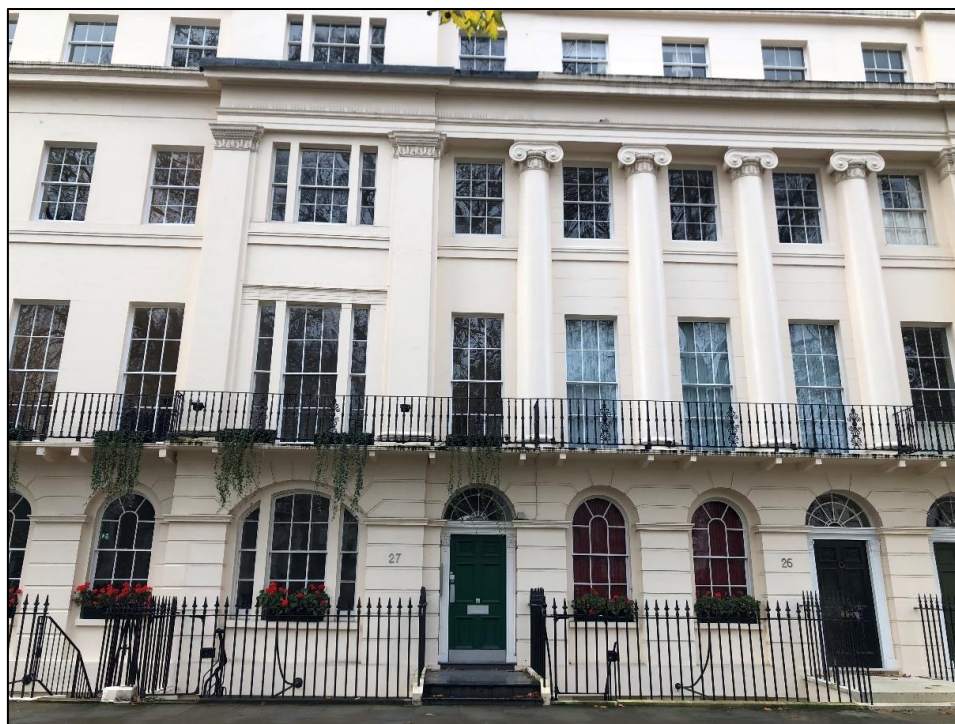
Plate 2: View looking W showing the front elevation of No. 27 Fitzroy Square
