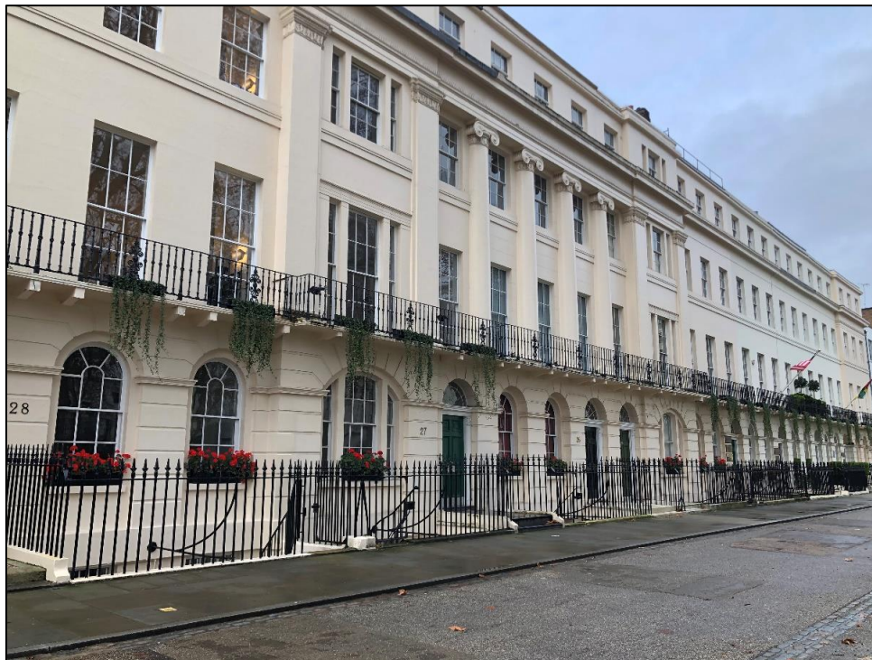
Plate 1: Oblique view looking NW showing the terrace at Nos. 20-32 Fitzroy Square
