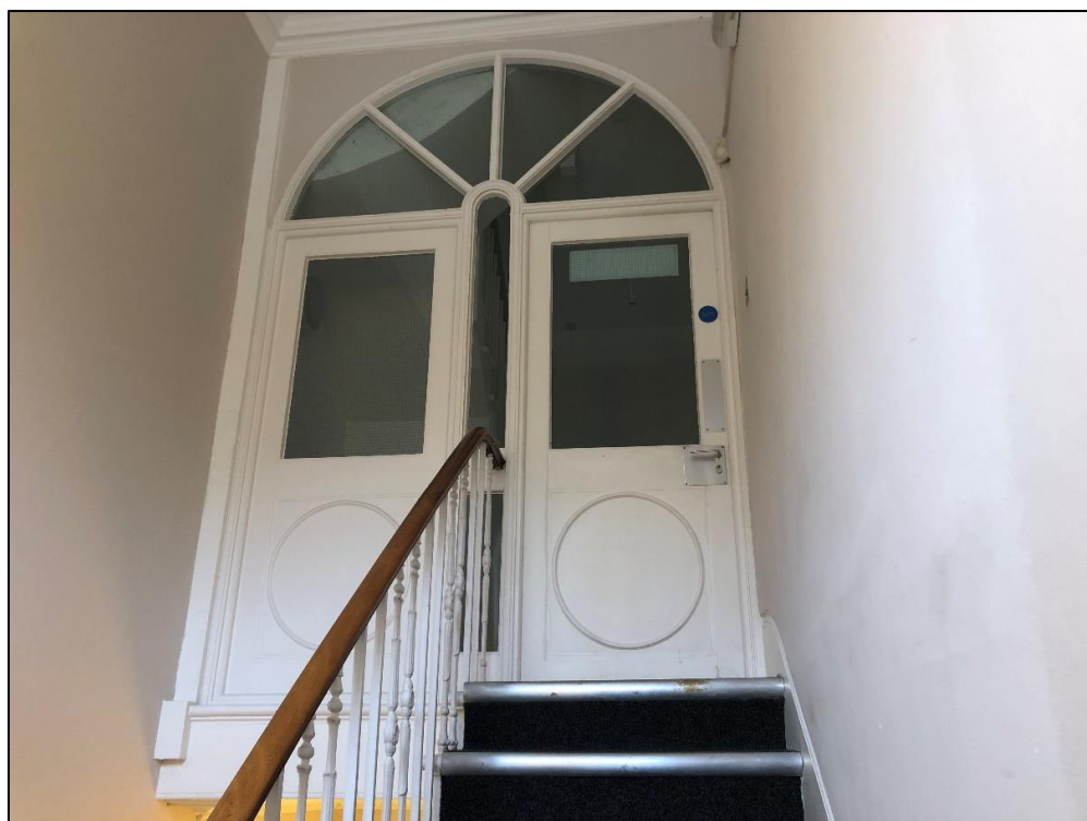
Plate 24: View looking up staircase towards glazed door to second floor landing
