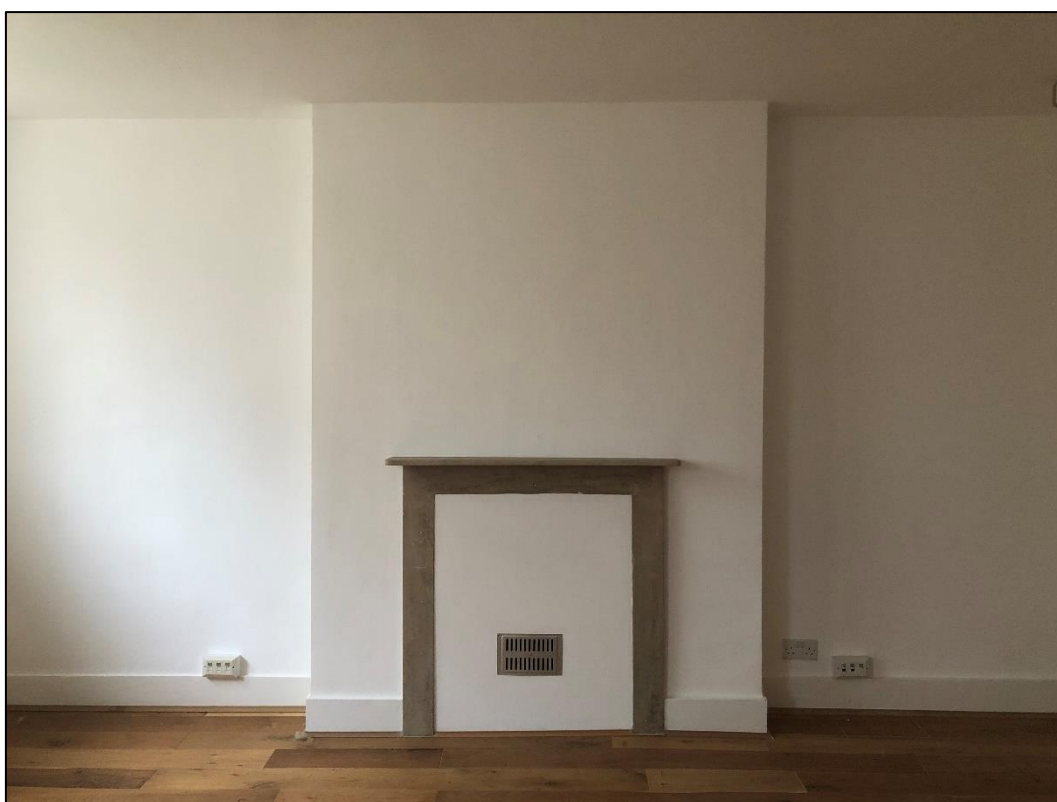
Plate 40: View looking S towards blocked fireplace in third floor front room
