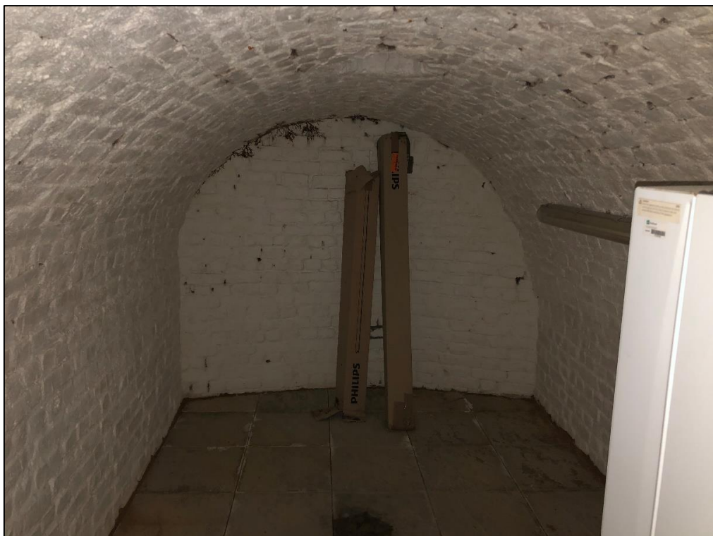
Plate 52: View looking E showing barrel vaulted roof in basement
