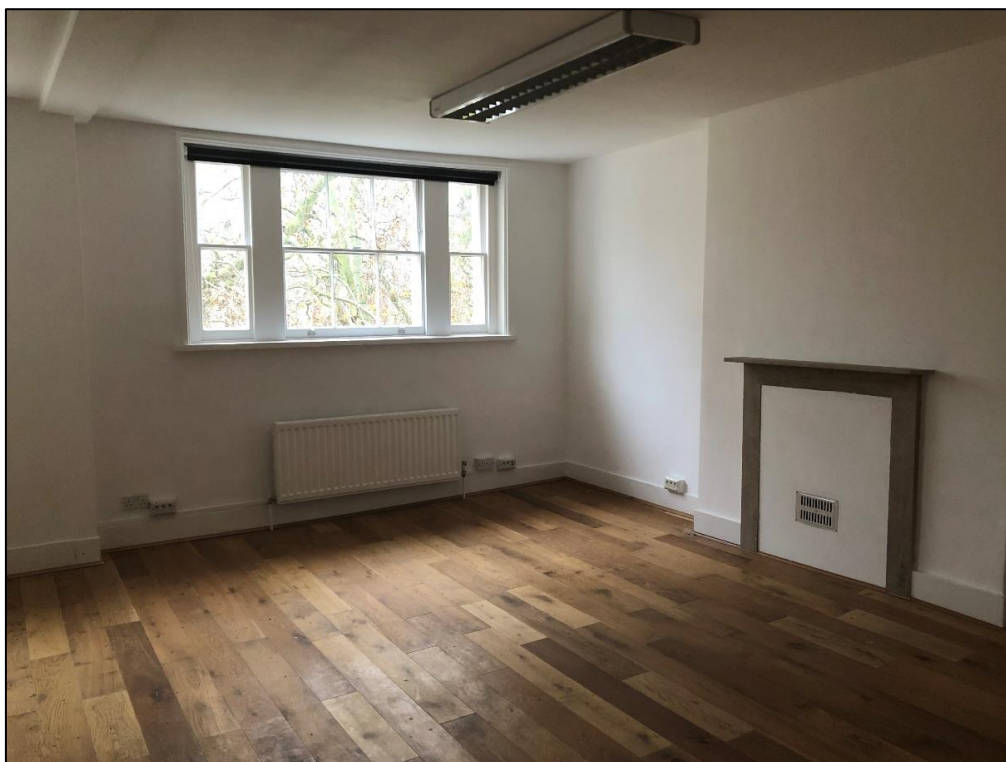
Plate 39: General view looking SE across third floor front room
