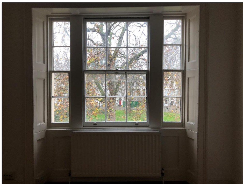
Plate 30: View looking E showing detail of tripartite sash window in second floor front room
