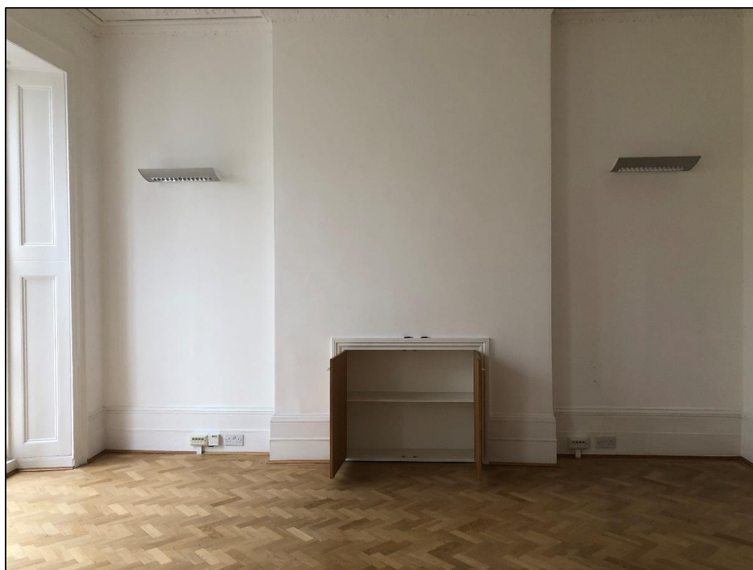
Plate 20: View looking S showing former fireplace (now wall cupboard) in S wall of first floor front room
