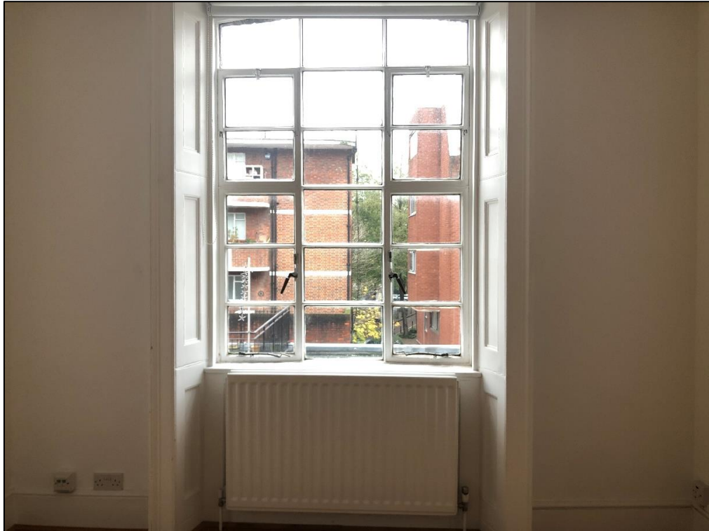
Plate 35: View looking W showing casement window in second floor back room
