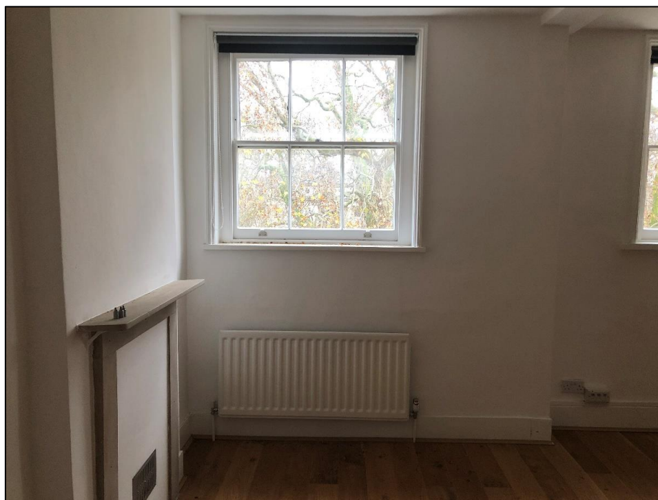
Plate 42: View looking E showing sash window and fireplace in the N half of the third floor front room
