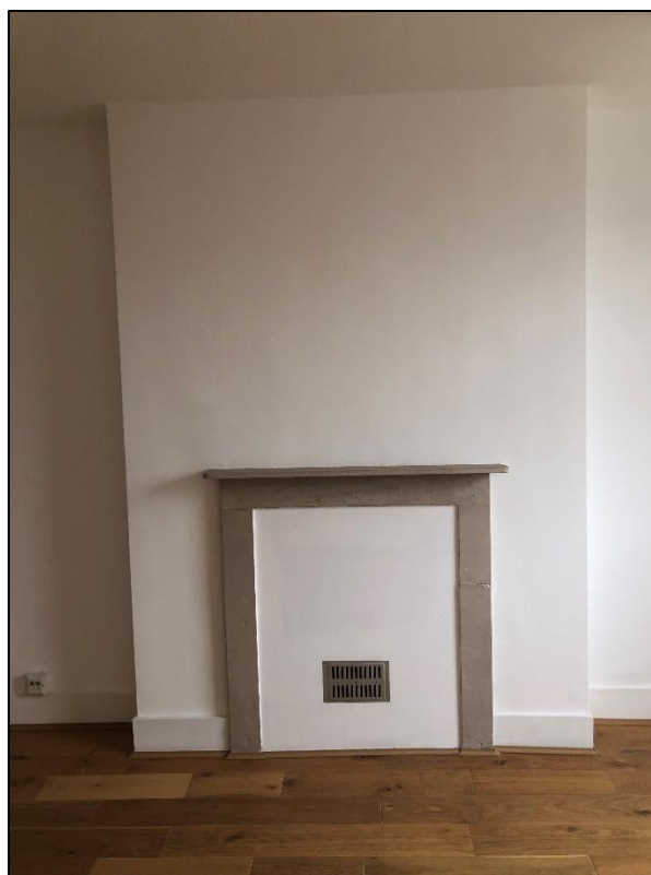
Plate 45: View looking S showing fireplace in S wall of back room on third floor
